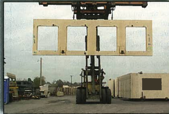
Fig. 22. Handling of precast panels was facilitated by cast lift inserts.
