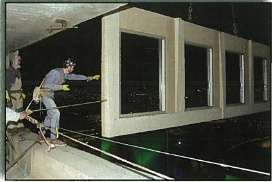
Fig. 28. By utilizing the tower crane at night, the precast concrete erectors maximized the efficient use of equipment by all trades on the St. Regis project.
