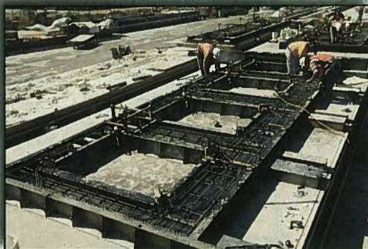
Fig. 18. Steel reinforcement bar cages were suspended with additional form supports to ensure quality control of final finish appearance.
