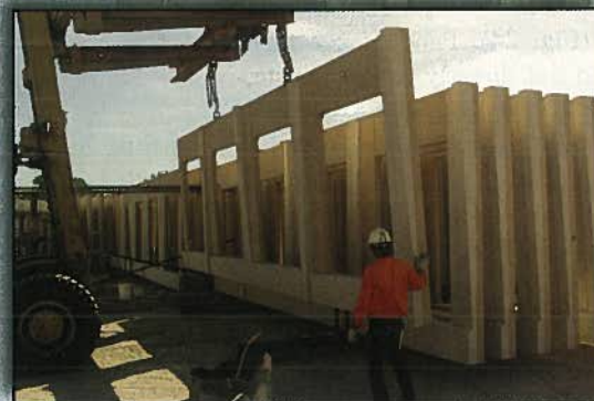
Fig. 23. Precast panels are stored facing north to avoid ultraviolet-radiation bleaching.
