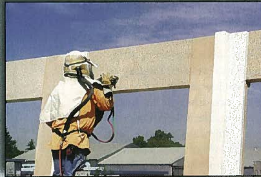
Fig. 21. Sandblasting required special care and attention by the finishing craftsmen and Clark Pacific's West Sacramento, Calif., manufacturing facility.
