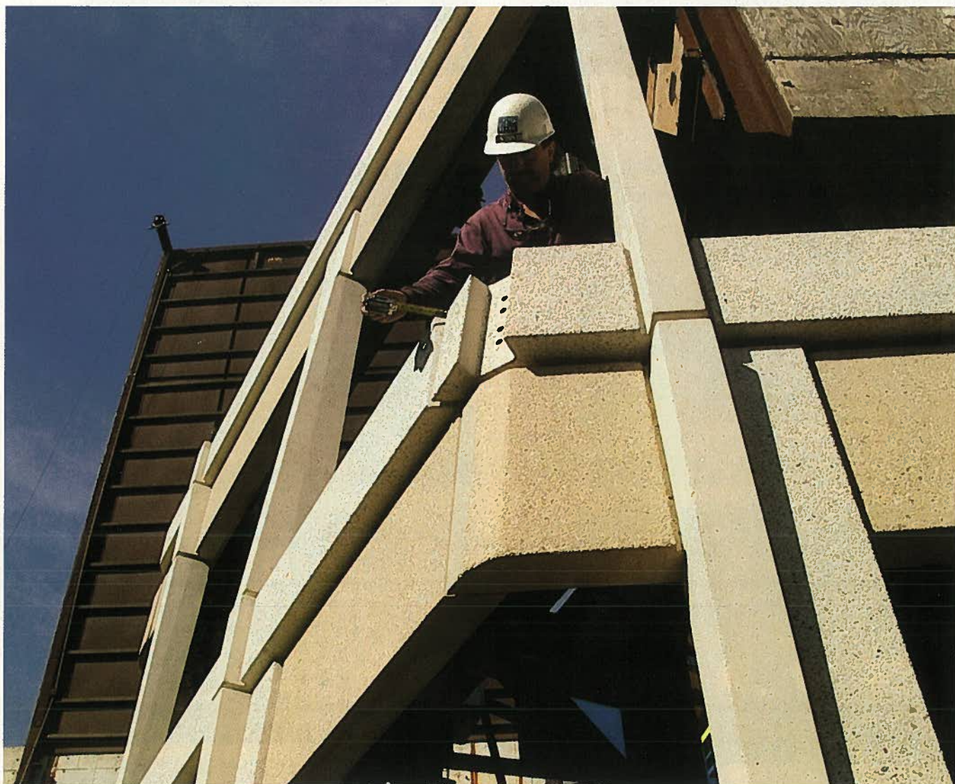
Fig. 31. Erection of full-scale mock-up chamfers is shown for the St. Regis Hotel & Residences.
