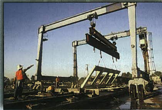
Fig. 20. Panels are stripped in the morning.
