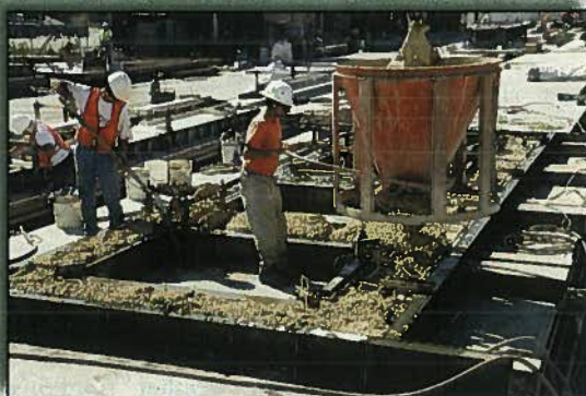
Fig. 19. The placement of concrete is shown being poured into forms.
