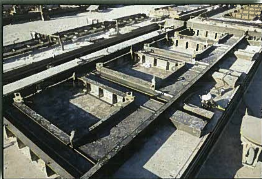
Fig. 16. Deep raised steel forms were used for forming the punched precast concrete window panels.
