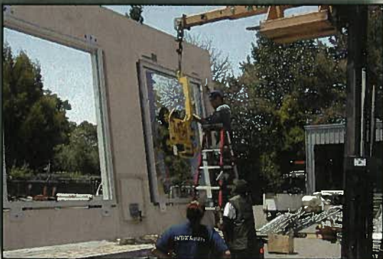
Fig. 26. Pre-glazing of wall panels prior to erection is an excellent example of utilizing the optimum efficiencies possible with precast concrete manufacturing.
