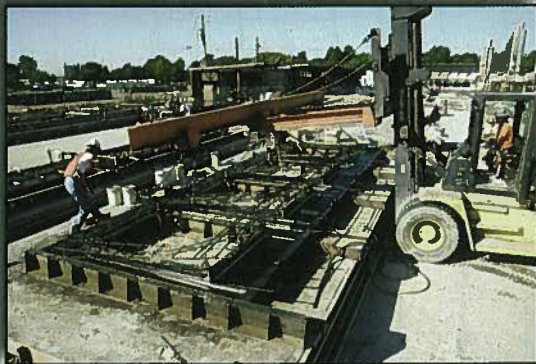
Fig. 17. The placement of pre-tied steel reinforcing cage is shown being put into form.
