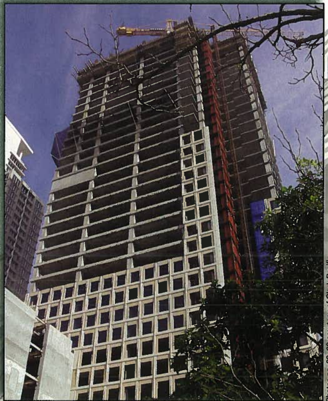
Fig. 30. Erection of preglazed and finished precast wall panels resulted in rapid story completion for the St. Regis Hotel & Residences.
