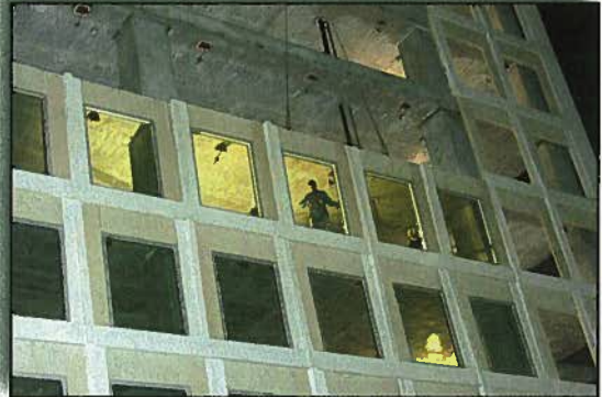
Fig. 29. This photo shows nighttime erection of precast concrete wall panels.
