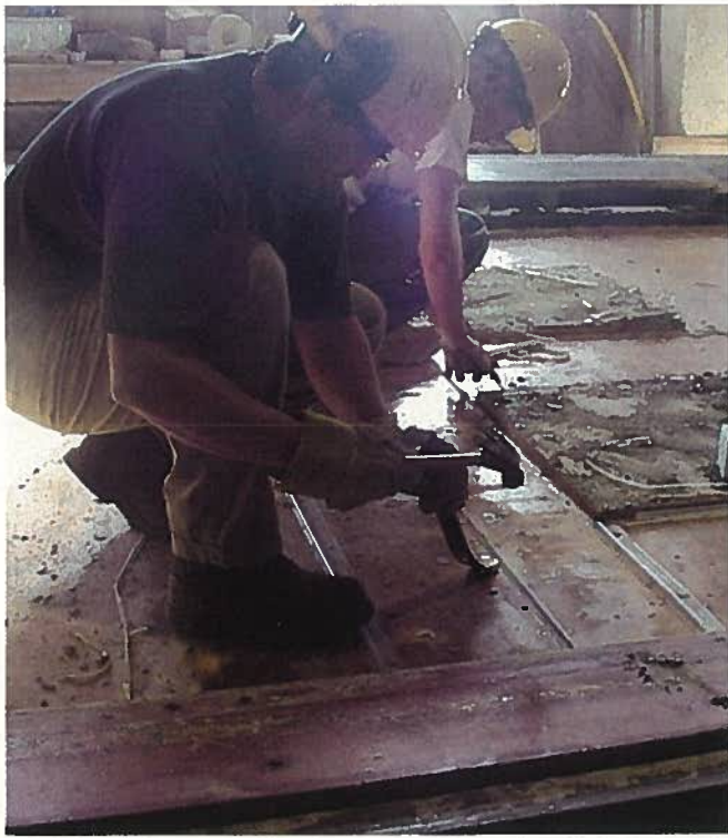
Fig. 5. Bed setup is a major area of waste in precast concrete plants and offers many opportunities for reducing waste through more efficient procedures, standardization, and improved material flow.
