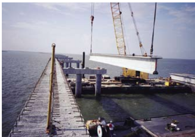
Fig. 10. Erection of 78 in. (1980 mm) deep Florida bulb tee girder.
