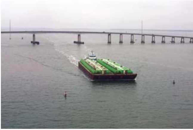
Fig. 11. Potential ship impact forces controlled the design of the Intracoastal Waterway, or main channel section, of the bridge.
