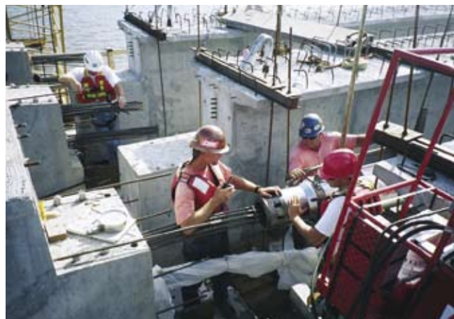
Fig. 21. Installation of post-tensioning tendons.
