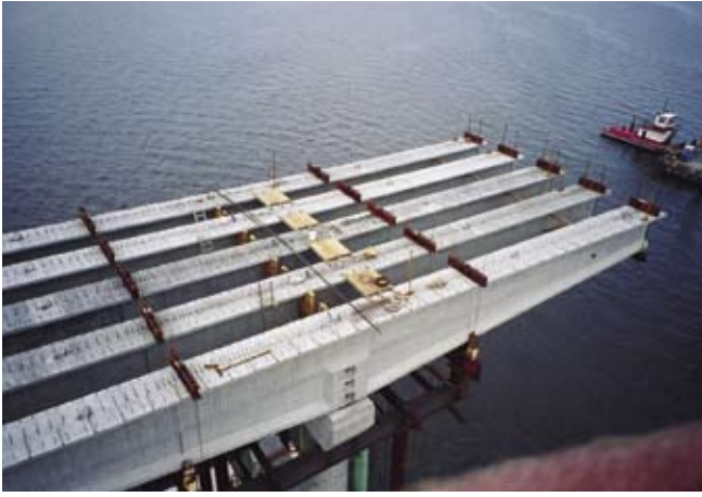
Fig. 14. Precast concrete haunch segments with girder depth varying from 6.7 to 12 ft (2.0 to 3.7 m).
