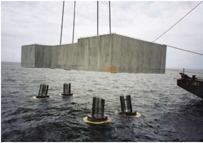
Fig. 17. Erection of precast concrete stay-in-place footing forms saved erection time.
