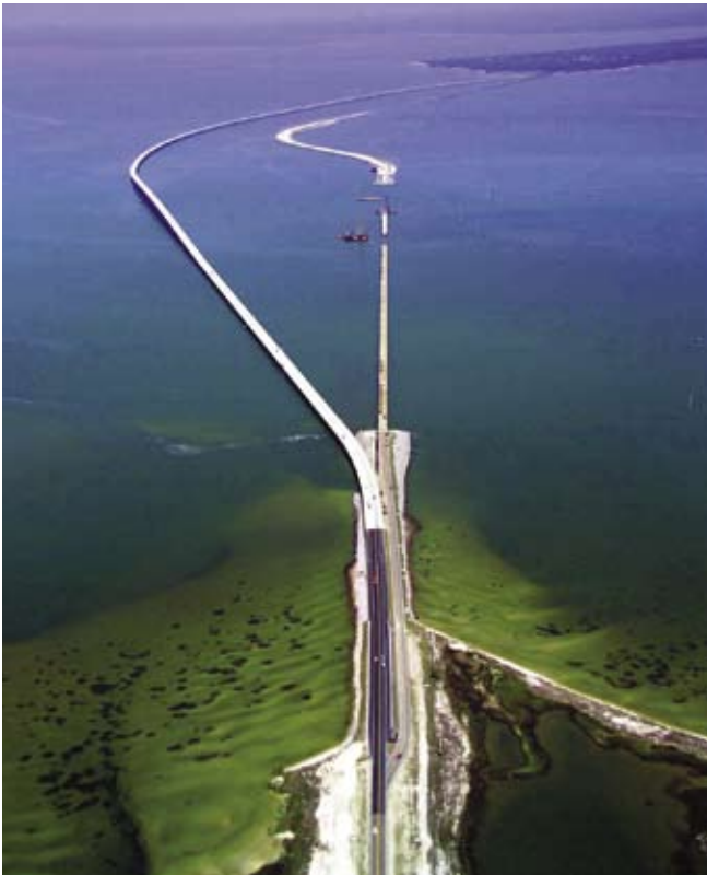
Fig. 2. Aerial photo shows St. George Island at the bottom of the frame and looks northward toward the small Bird Island causeway and onward to the Florida mainland. The new replacement bridge was constructed to the west (on the left above) of the old bridge.
