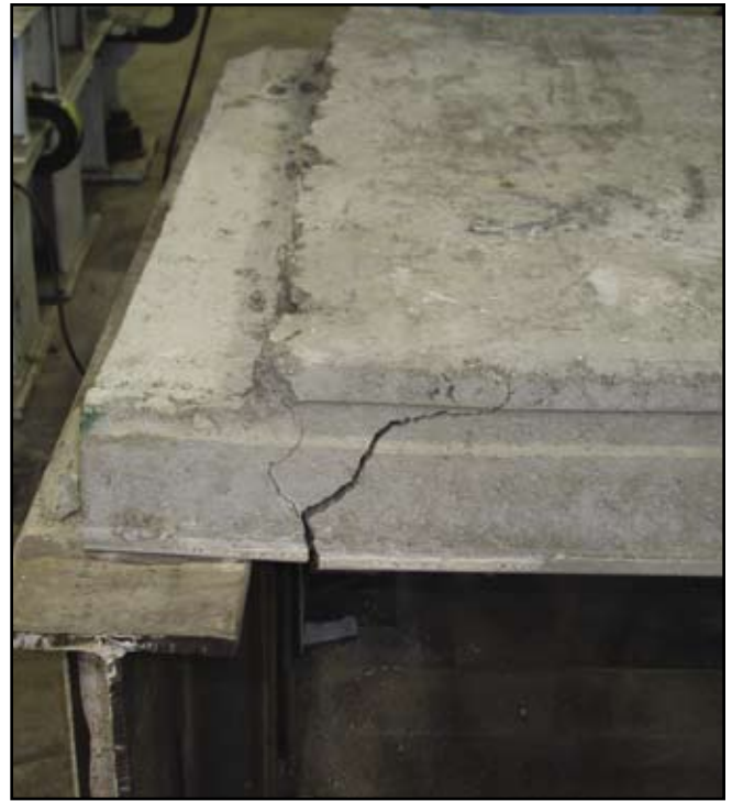
Fig. 5. Typical failure in hollow-core slab.
