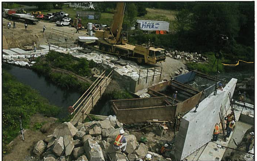
Fig. 15. Day 2, 11:17 a.m.: Setting abutment panels.
