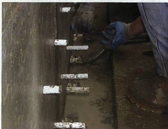
Fig. 25. Closeup of grouting splice sleeve.
