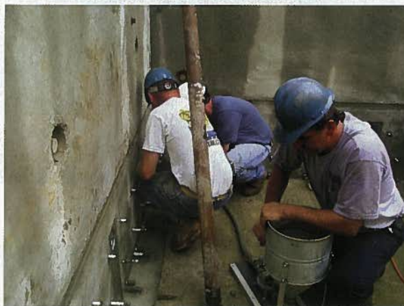
Fig. 24. Grouting splice sleeves.
