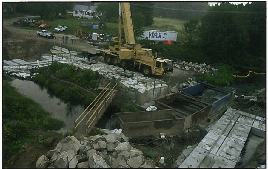
Fig. 14. Day 1, 5:05 a.m.: Footings complete.
