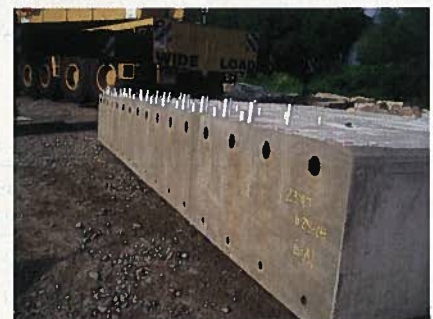
Fig. 13. Abutment stem element, front side down.
