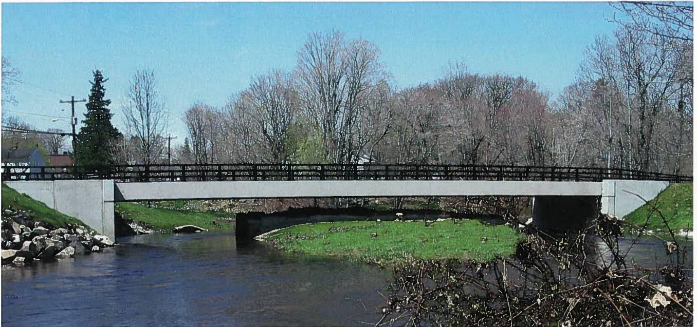
Fig. 1. View of Mill Street Bridge.
