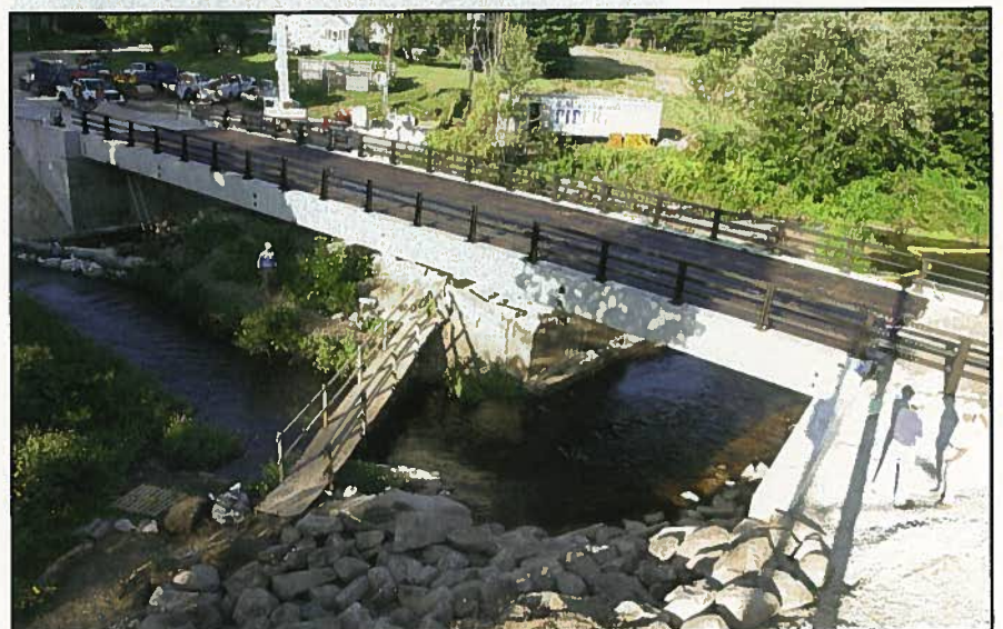
Fig. 22. Day 8, 5:40 p.m.: Deck membrane complete, awaiting pavement.
