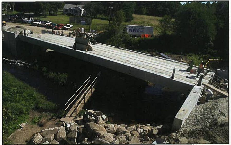
Fig. 20. Day 7, 10:27 a.m.: Preparing for transverse post-tensioning.
