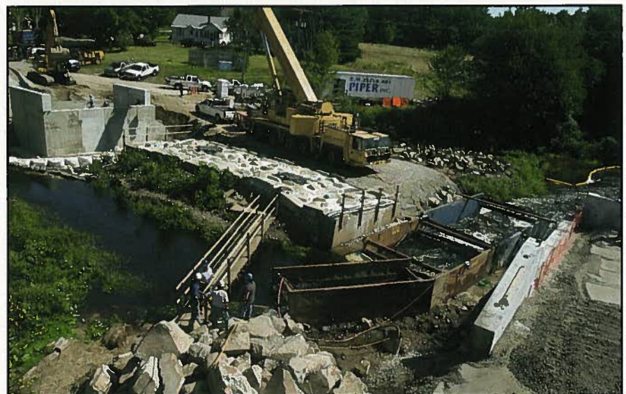
Fig. 16. Day 4, 10:47 a.m.: Backfilling substructure.
