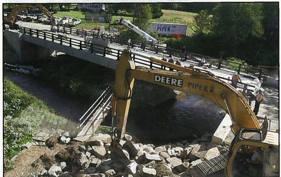
Fig. 21. Day 8, 9:40 a.m.: Completing riprap.
