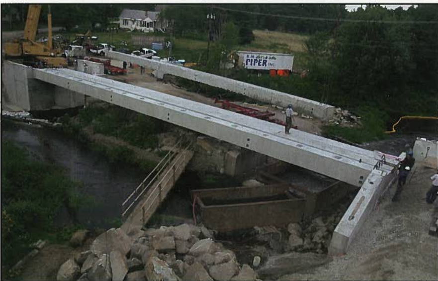
Fig. 18. Day 5, 7:37 p.m.: Setting fourth box beam.
