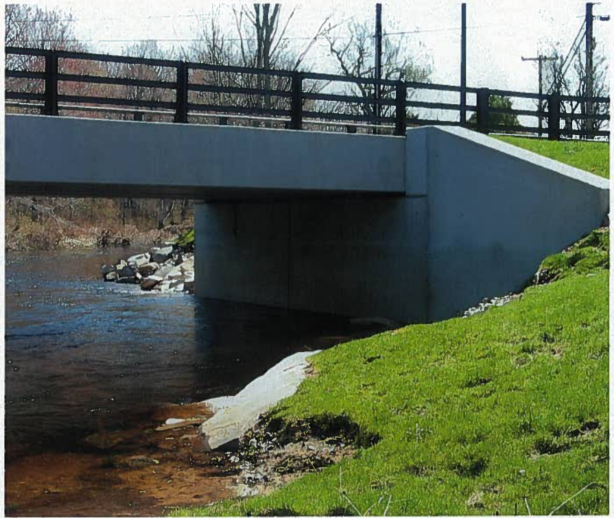
Fig. 26. View of the completed south abutment.
