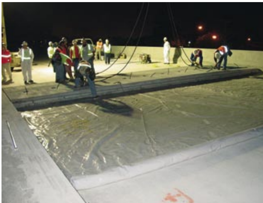
Fig. 11. The polyethylene sheeting is rolled out over the concrete base just prior to the placement of each panel.
