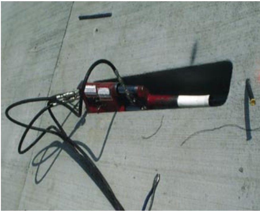
Fig. 13. A monostrand stressing ram is used to tension the post-tensioning strands from the central stressing pockets.
