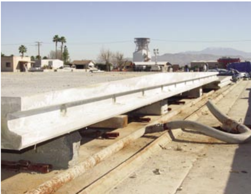
Fig. 9. Precast panel after removal from the forms, showing its unique cross section.
