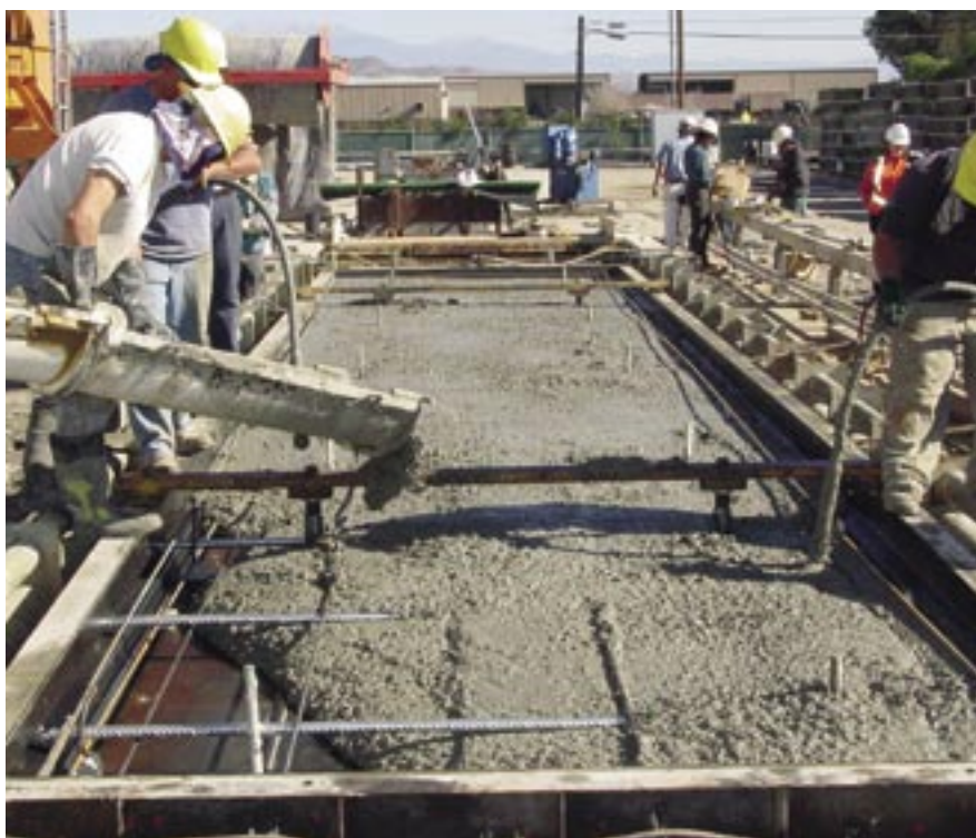
Fig. 8. Concrete placement for a base panel.
