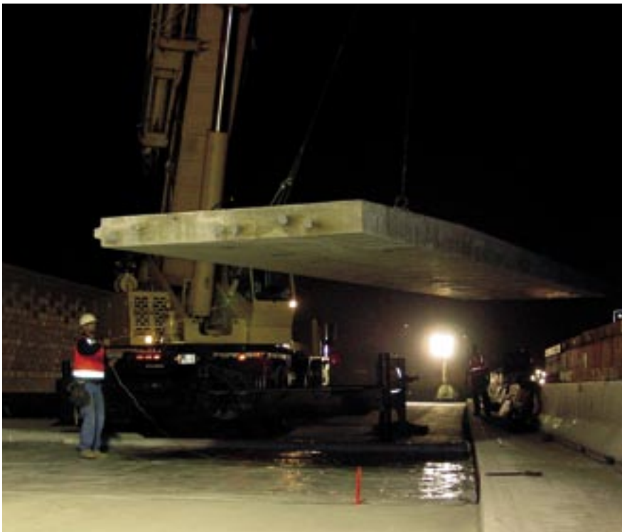
Fig. 10. During installation, each panel is lifted off the truck, swung over the concrete barrier, and set in place.
