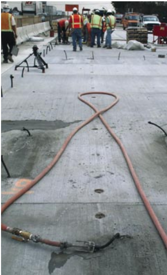
Fig. 14. Grout is pumped into the post-tensioning tendons from ports at the central stressing pockets.
