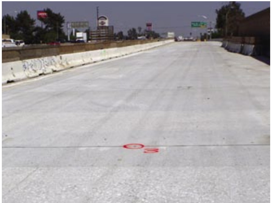
Fig. 15. The finished precast pavement prior to opening to traffic.
