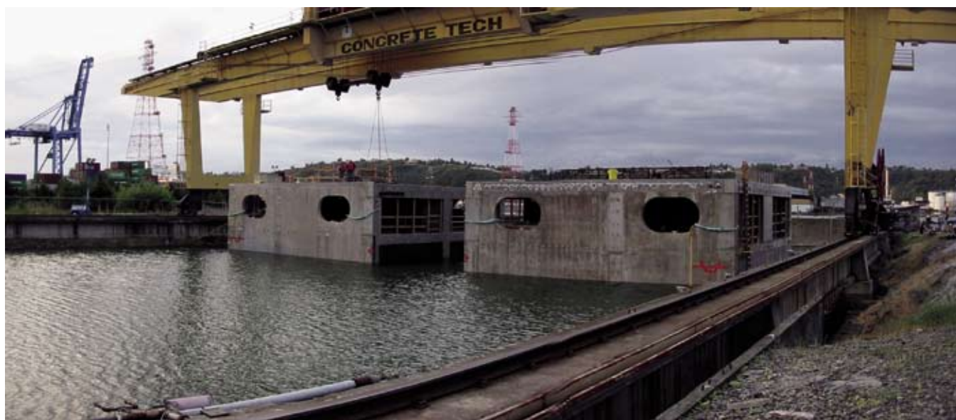
Fig. 19. Completed test bed module during flooding of CTC's graving dock.
