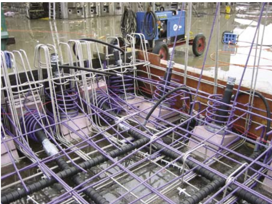
Fig. 11. External panel reinforcement shows arrangement of corrosion-resistant metals selected to achieve 100-year repair-free service life of HSLWC: (Type 316) stainless steel and fusion-bonded epoxy-coated steel.
