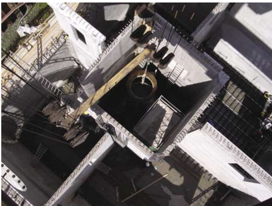
Fig. 17. Overhead view of MHP precast concrete construction with walls in place.
