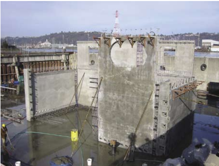
Fig. 15. Partial erection of MHP precast concrete wall panels at CTC Tacoma, Washington, graving dock facility.
