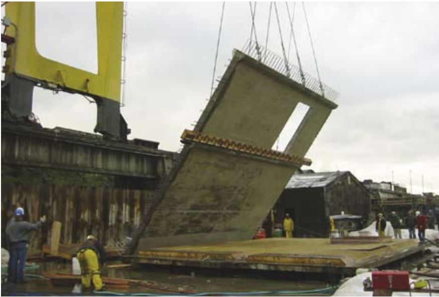
Fig. 14. Erection at CTC precasting facility showing hoisting of precast concrete wall panel.
