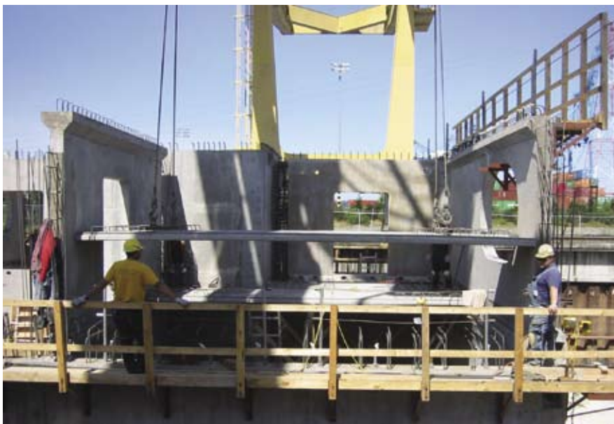
Fig. 16. Hoisting of precast concrete deck panel.
