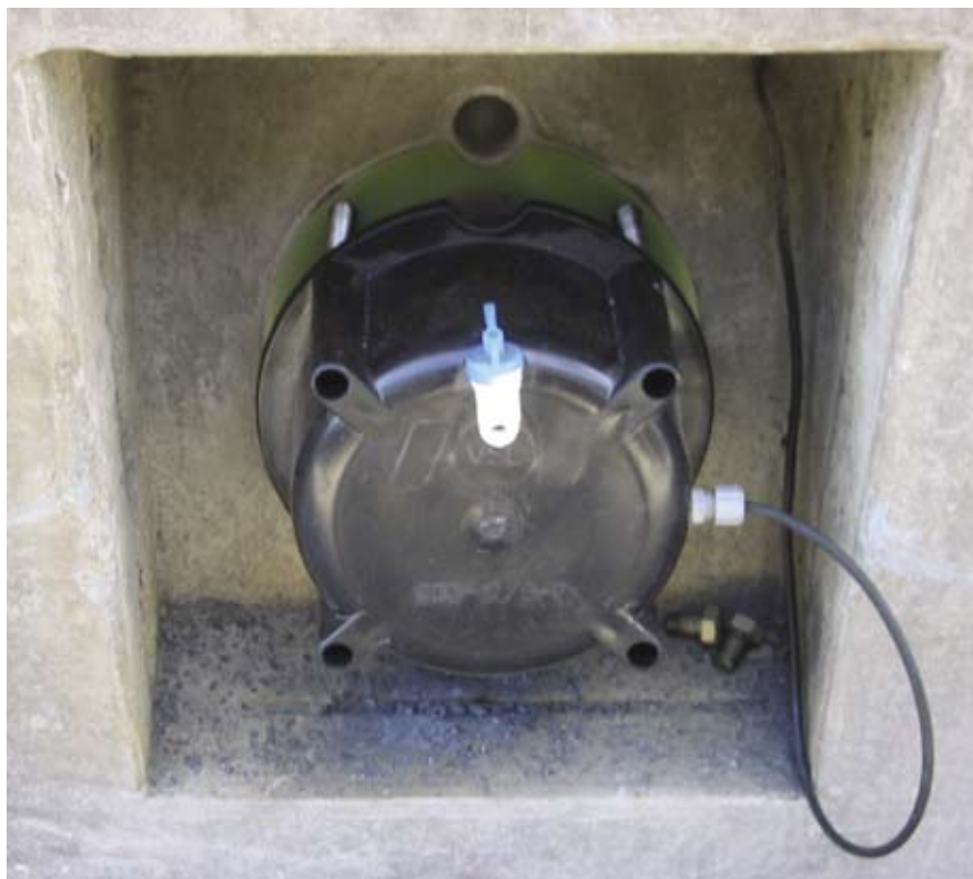
Fig. 12. The second module used a combination of encapsulated post-tensioning tendons and anchors and encapsulated, electrically isolated tendons.
