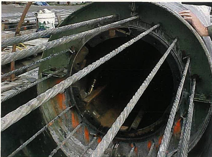
Fig. 9. Closeup of collapsible hydraulic core form. (Courtesy of Pomeroy Corporation)
