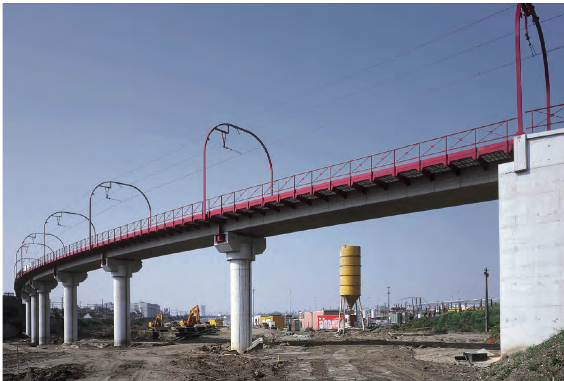
Fig. 13. Side view of single-track viaduct, extending about 495 ft (151 m) in length. (Courtesy of Tucrail)
