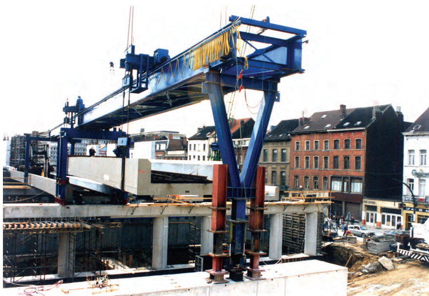
Fig. 7. Erection of precast, prestressed U-shaped deck at Brussels South Station using launching truss. (Courtesy of Tucrail)
