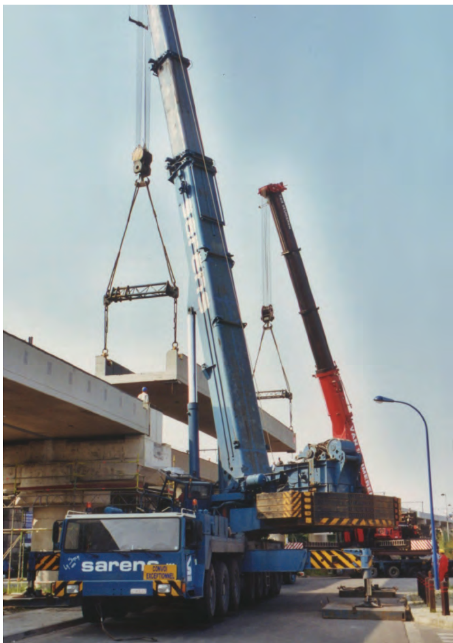
Fig. 10. Two cranes are used to install U-shaped deck near Brussels South Station. (Photograph by Bernard Espion)
