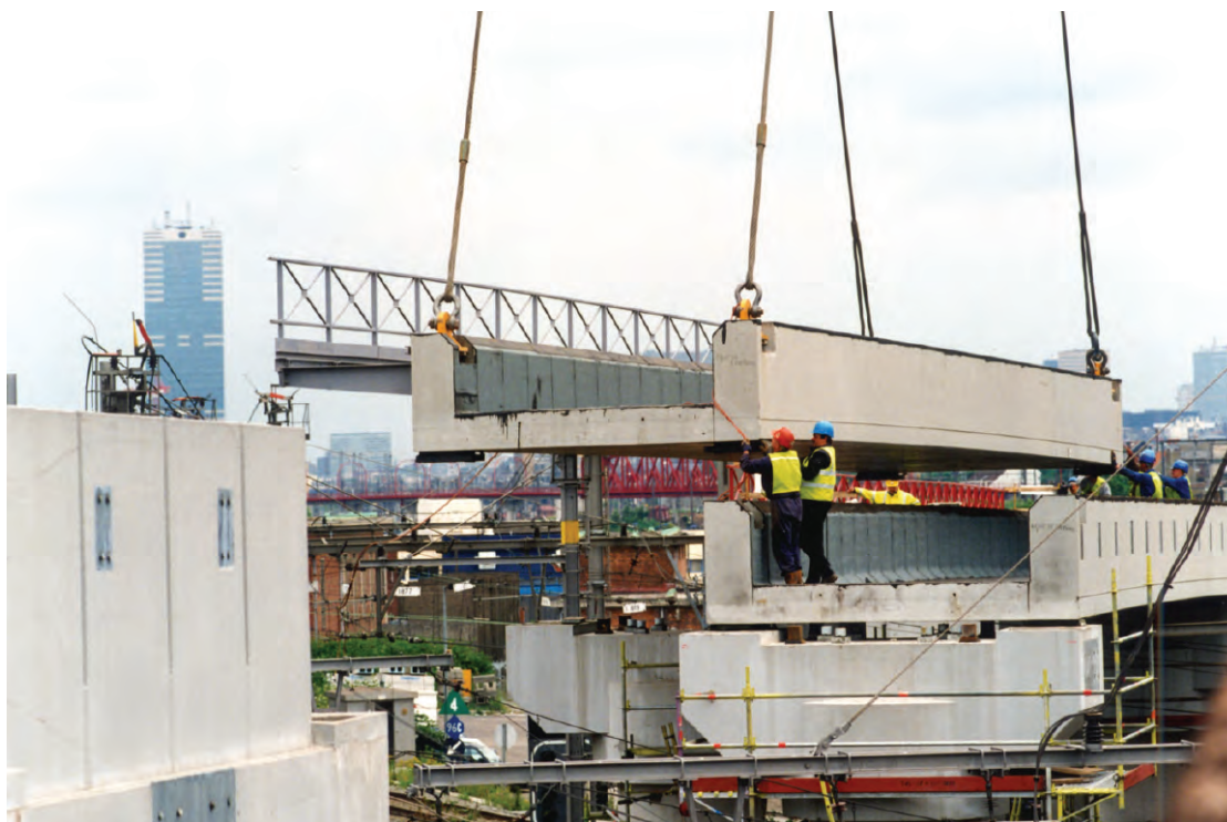
Fig. 11. Installation of U-shaped deck near Brussels South Station. (Courtesy of Tucrail)
