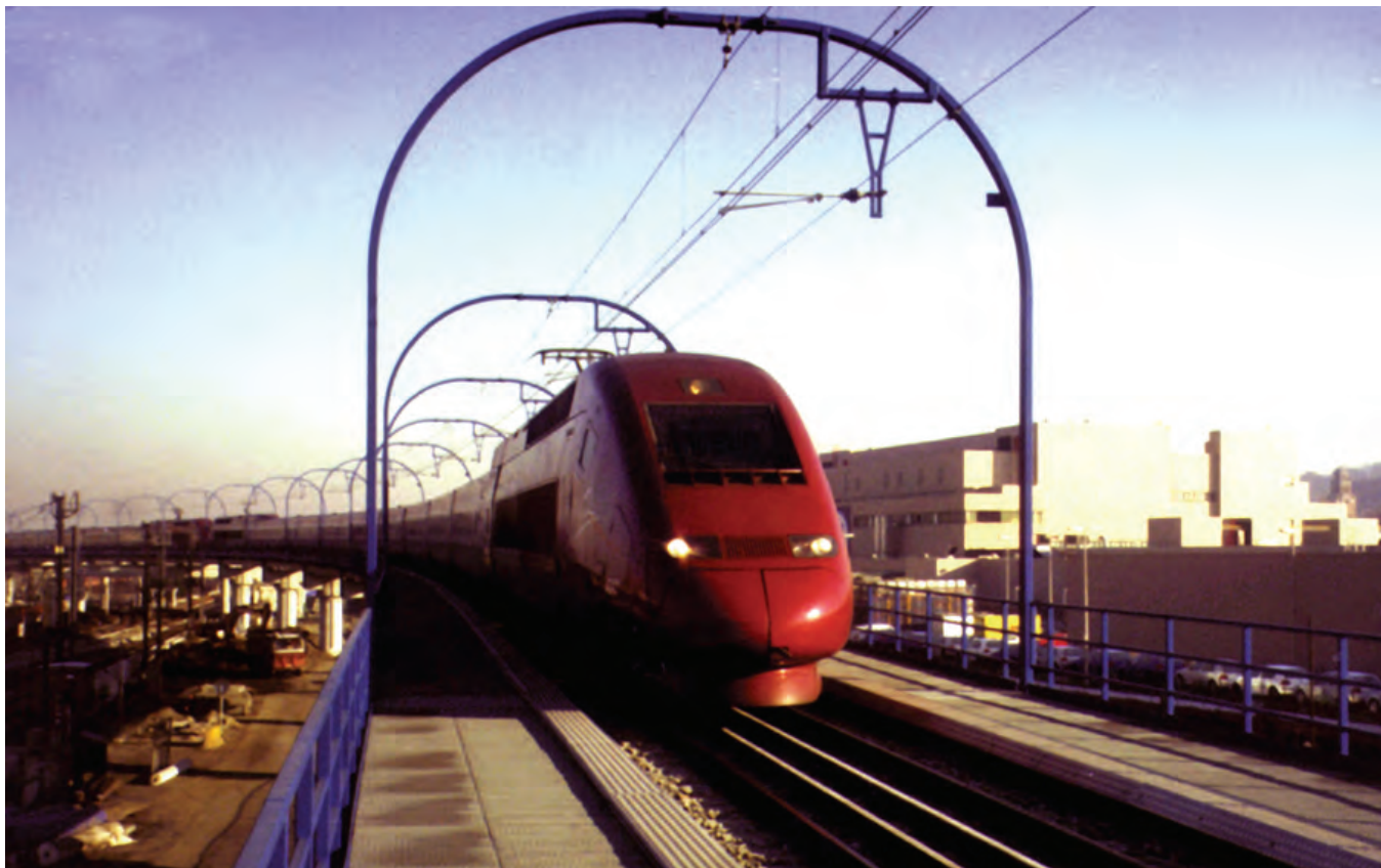
Fig. 1. An innovative composite precast, prestressed precambered U-shaped concrete deck is providing the structural support for the high speed railway trains in Belgium. (Courtesy of TUCrail)
