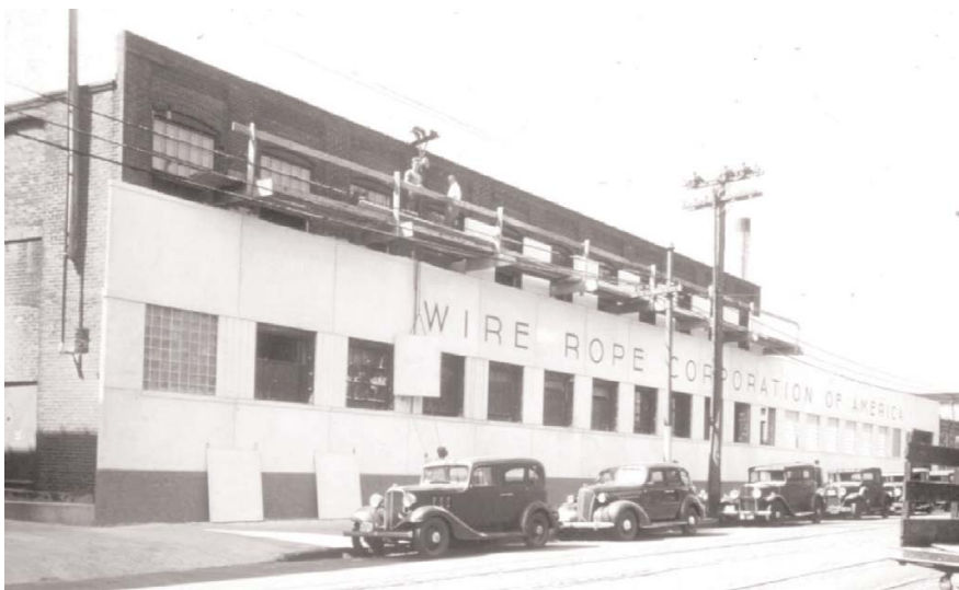
Fig. 28. Mo-Sai panels were used as veneer on masonry construction for this project in New Haven, Connecticut.
