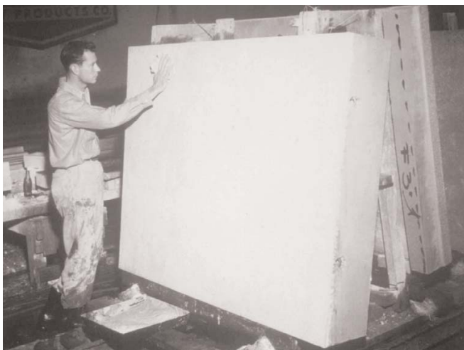
Fig. 24. After panel is brushed, it is "smeared in" to fill in holes and imperfections.
