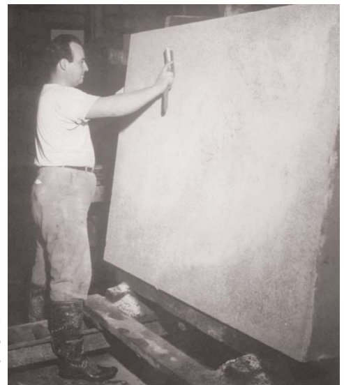
Fig. 23. Face is wire brushed to expose aggregate.
