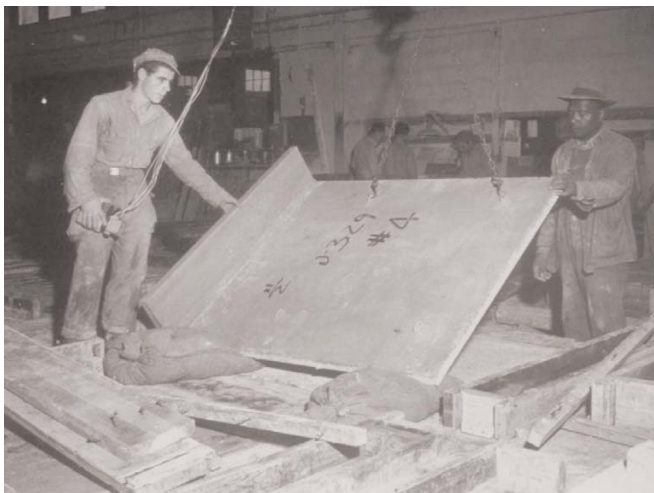
Fig. 22. Stripping the panel from the mold with excelsior filled sack to protect edges from chipping.
