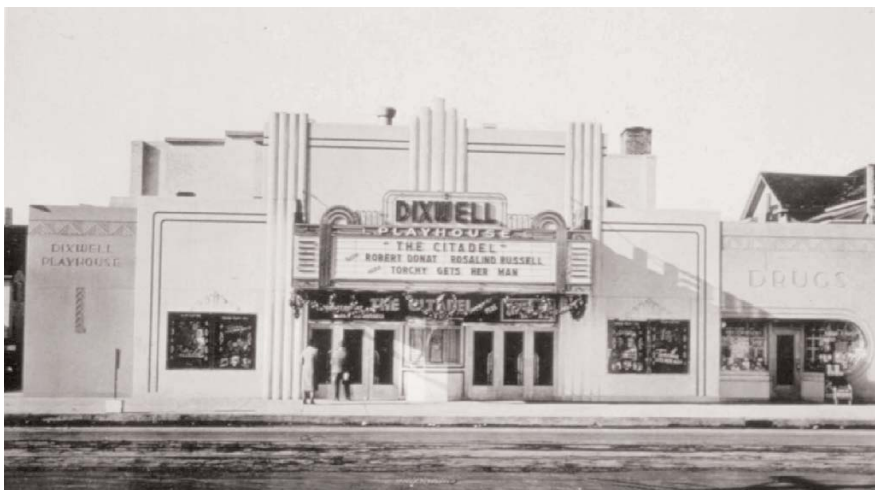
Fig. 27. Dixwell Playhouse, Hamden, Connecticut used Mo-Sai panels as veneer for masonry construction.
