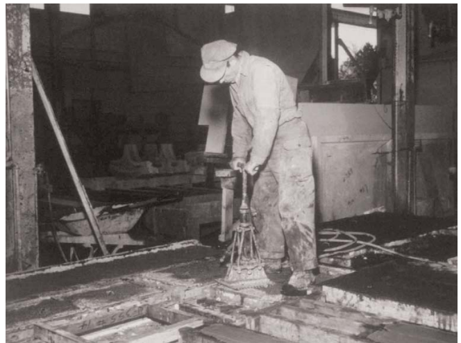
Fig. 21. Vibration of slab in its final stages. Top of side forms are being vibrated to help mix go into place at slab ends.
