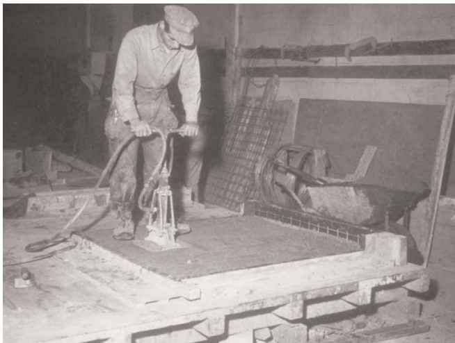
Fig. 20. The backing mix being vibrated into place.
