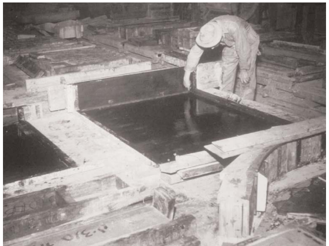
Fig. 13. Worker filling in the joints of mold with molding plaster to prevent leaks. Mold is for 2 in. (50 mm) slab with 10 in. (250 mm) return.
