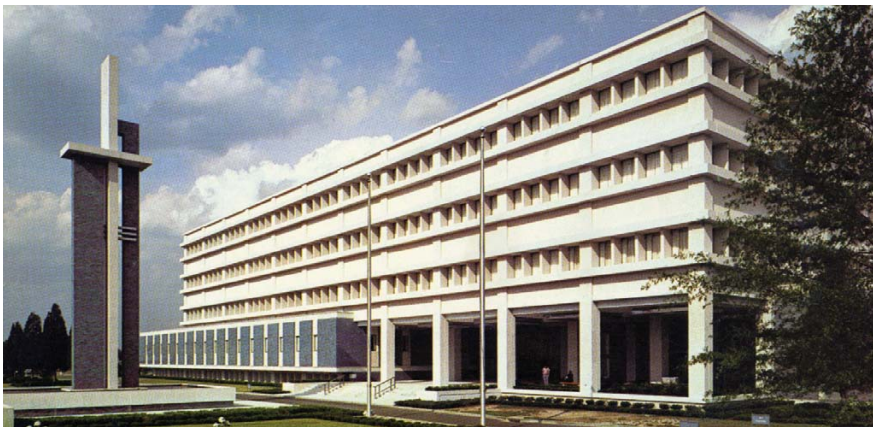
Fig. 1. Blue Cross-Blue Shield Office Building, Richmond, Virginia.
