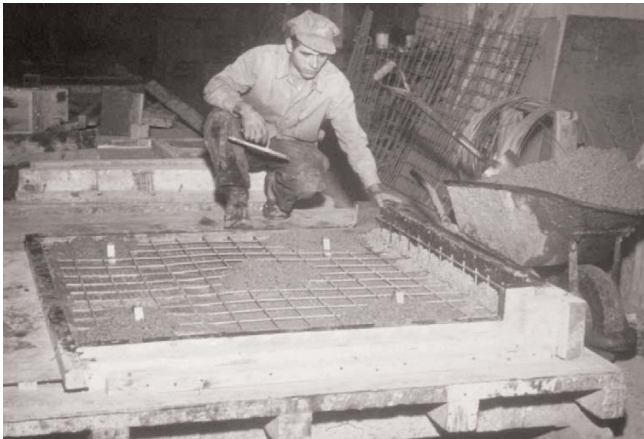
Fig. 18. Reinforcement held in proper position on top of vibrated facing by small mounds of backing mix under the mesh.
