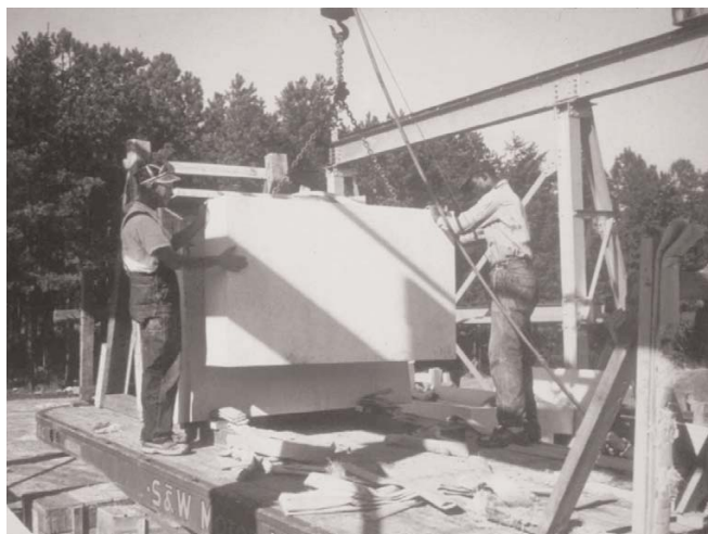
Fig. 25. Mo-Sai panels being loaded on truck which has wooden A frame easels.
