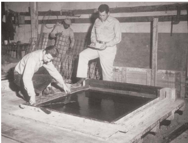
Fig. 14. Inspector checking Mo-Sai mold for size, shape and trueness.
