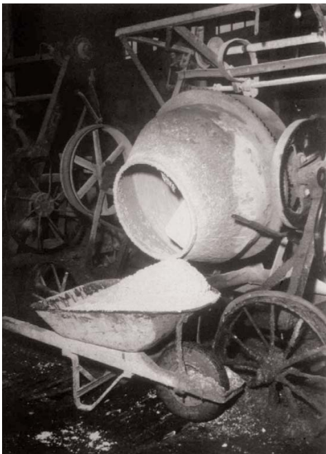
Fig. 16. Note stiffness of low water-cement ratio facing mix just discharge from mixer.
