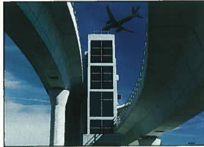
Co-Winner Best Non-Highway Bridge AirTrain Light Rail System John F. Kennedy International Airport Queens, New York
