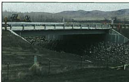
Winner Best Bridge with Spans Between 65 and 135 ft (20 and 41 m) Little Oak Creek Bridge Corson County, South Dakota
