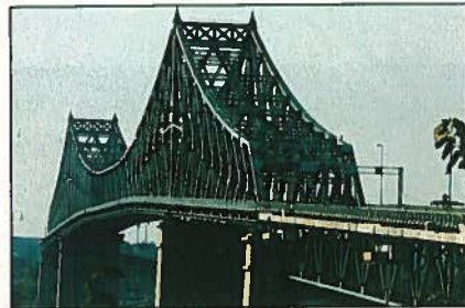
Winner Best Rehabilitated Bridge Jacques Cartier Bridge Montreal, Quebec, Canada
