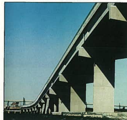
Winner Best Bridge with Spans Greater than 135 ft (41 m) Ocean City-Longport Bridge Ocean City, New Jersey
