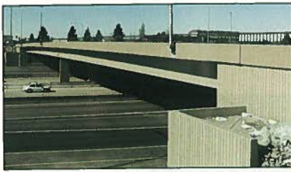
Winner Best Owner-Designed Bridge 38th Street Bridge Tacoma, Washington
