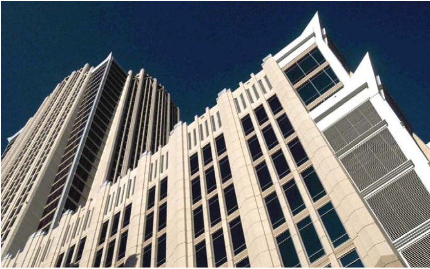
Fig. 6. Bold geometry in design allows the Hearst Tower to hold its own against the taller nearby structures.
