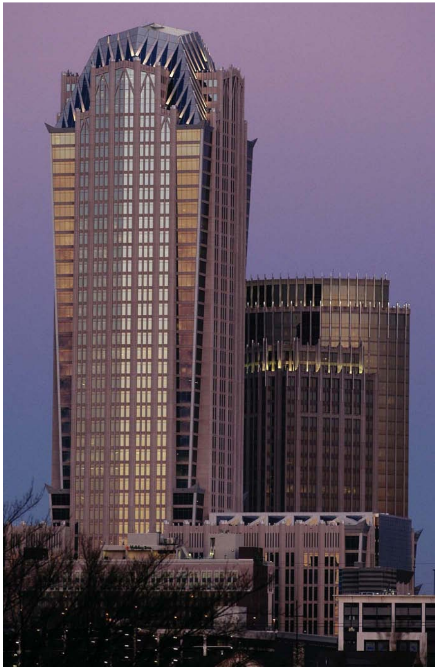
Fig. 1. Charlotte's Hearst Tower, a landmark 47-story commercial office structure in the heart of the city's financial district.
