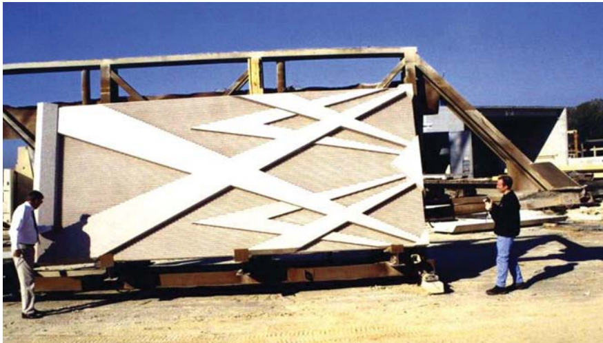
Fig. 10. A finished panel at the precaster's yard.
