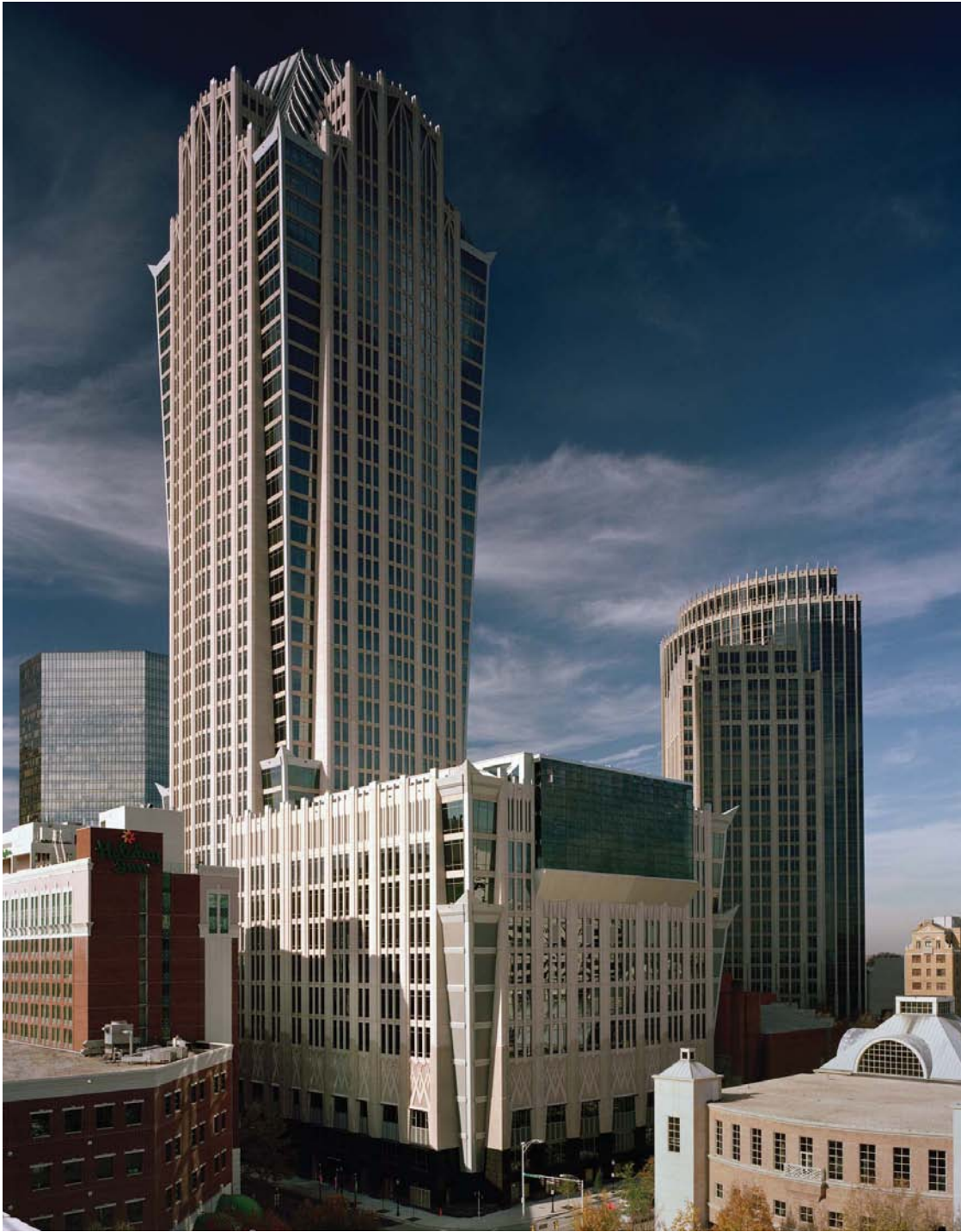
Fig. 15. The Hearst Tower rises boldly, standing as a proud landmark structure for the Charlotte skyline.
