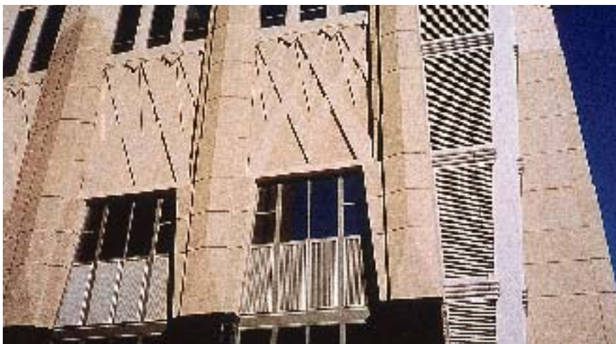
Fig. 11. The molds for these intricately detailed art deco pieces with a high degree of surface relief took almost two weeks to fabricate.
