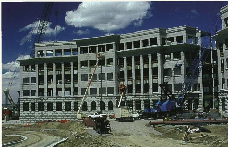
Fig. 15. Nearing the end of the installation of the architectural precast façade.
