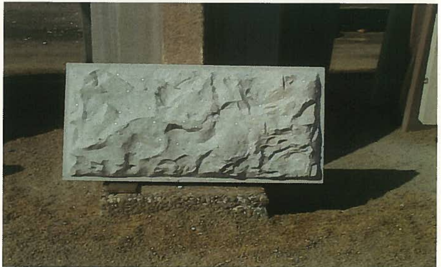
Fig. 13. A finished precast panel after acid washing the surface to expose quartz crystals.
