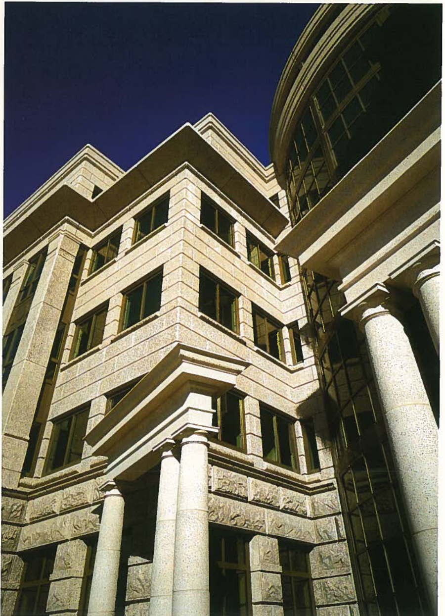
Fig. 6. Tapered Roman-Tuscan columns with the appearance of horizontal "stonework" joints, and prescribed architecture for historically precise entablature.
