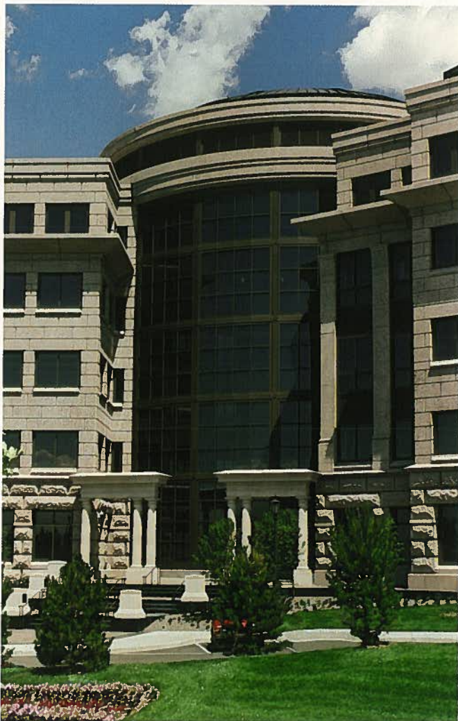
Fig. 2. Close-up view of the classic portals at the main visitor entrance, a glass-walled, domed rotunda, fronted by tapered Roman-Tuscan columns and entablature.
