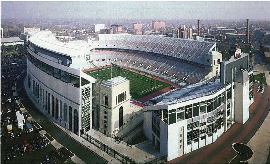
Fig. 6. The Horseshoe's original footprint is retained via an architectural break at the opening to the south end zone. (Photograph © 2002 Brad Feinknopf, Feinknopf Photography)
