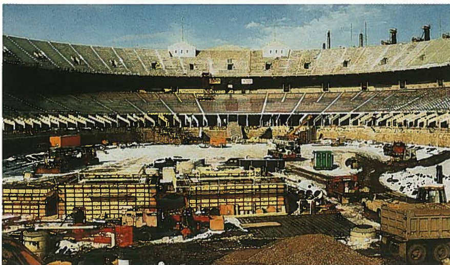
Fig. 9. Precast concrete erection moves simultaneously down from the north end zone.
