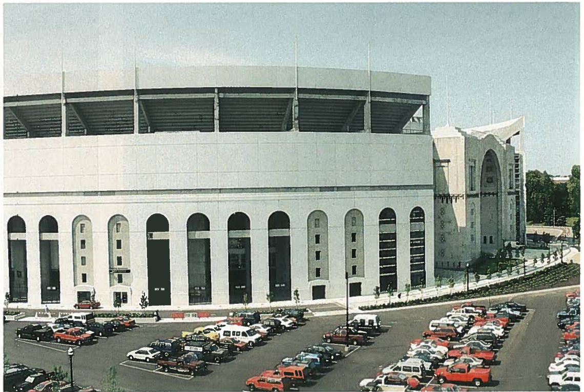
Fig. 18. New architectural precast wall panels blend the powerfully arcaded forms of the stadium expansion with the "old" architecture of the north rotunda.
