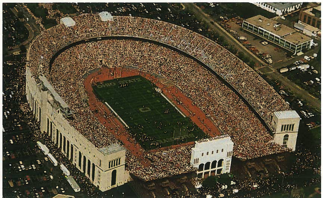
Fig. 3. Original stadium showing cornerstone towers and temporary bleachers at south end zone.
