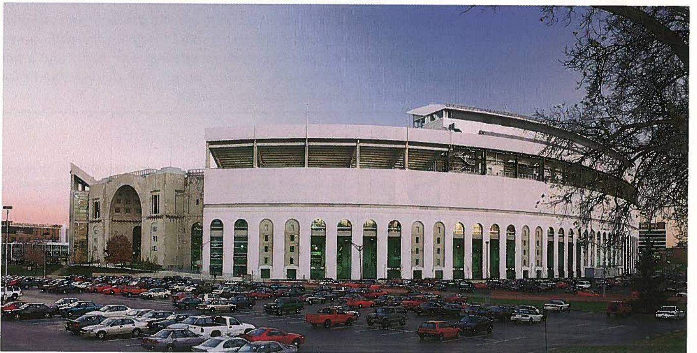
Fig. 22. The new precast exterior serves to complement, rather than compete with, the existing construction. (Photograph © 2002 Brad Feinknopf, Feinknopf Photography)
