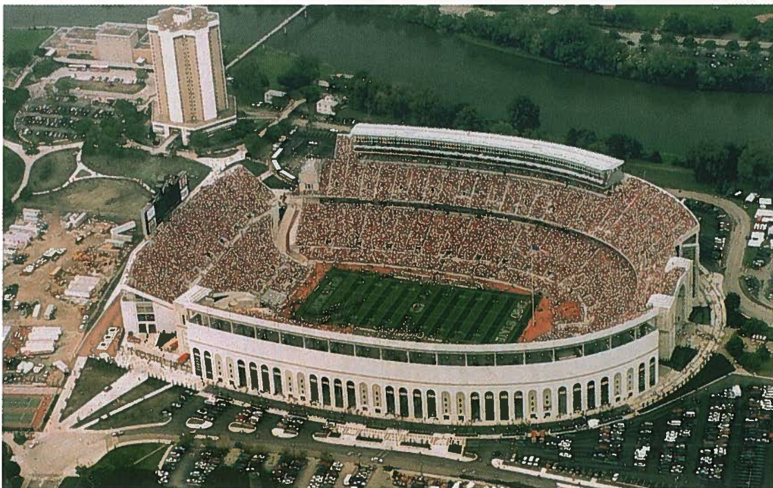
Fig. 7. Aerial view of the Ohio Stadium, looking west to the Oletangy River and showing south end zone entrance ramps and the narrow erection access on the east side of the stadium.
