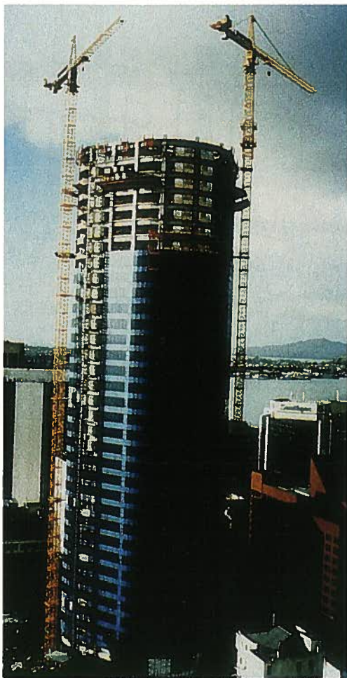
Fig. 15. Construction of the 152 m (499 ft) tall ANZ Tower using System 2 in Auckland, New Zealand.
