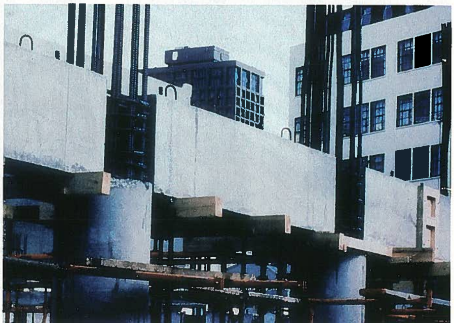
Fig. 12. Construction of a building frame using System 1 in New Zealand.
