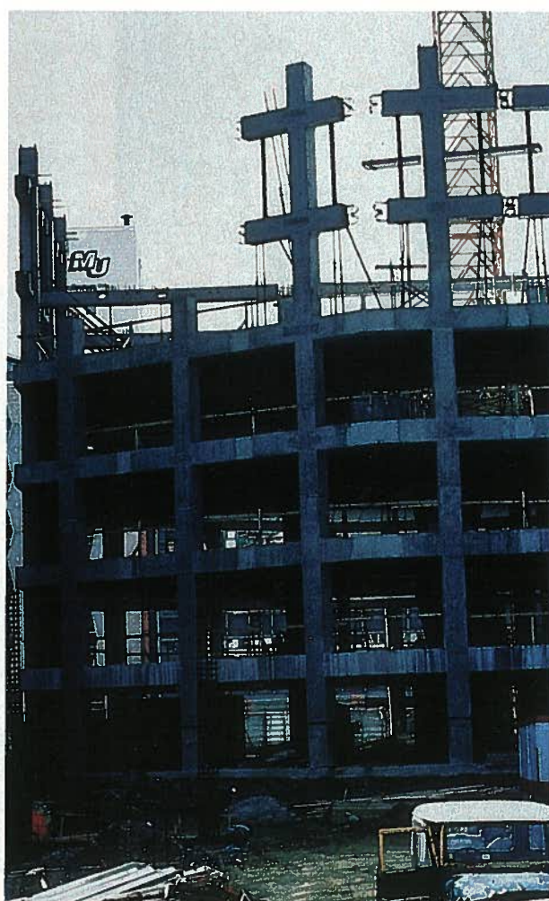
Fig. 16. Construction of the 13-story perimeter frame of Unisys House using two-story high cruciform-shaped precast units (System 3) in Wellington, New Zealand.
