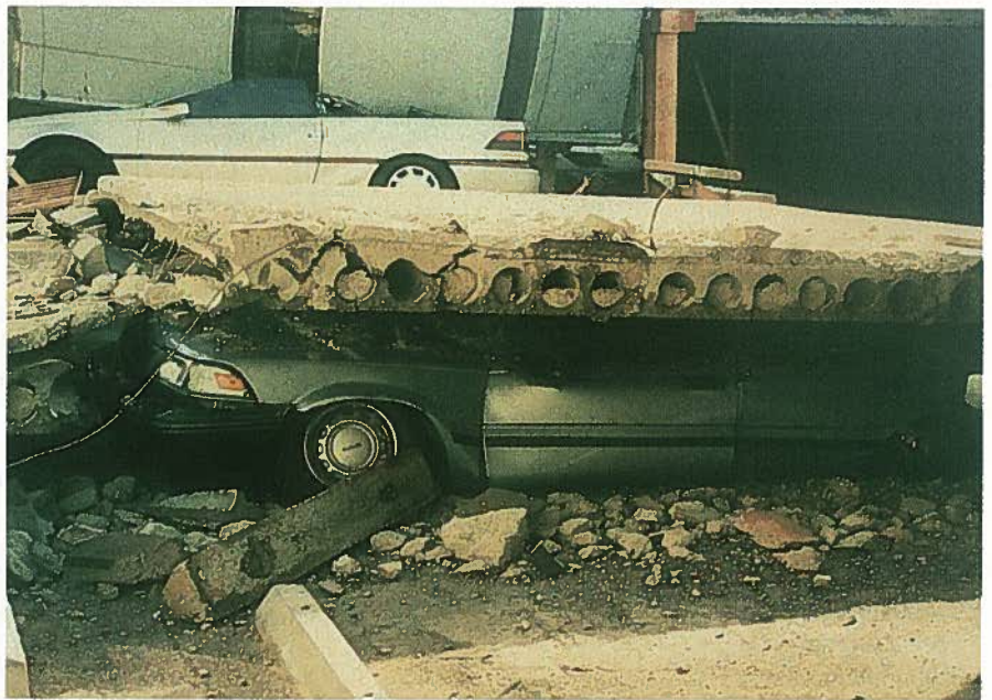
Fig. 8. Collapse of a hollow-core floor as a result of the 1994 Northridge earthquake.
