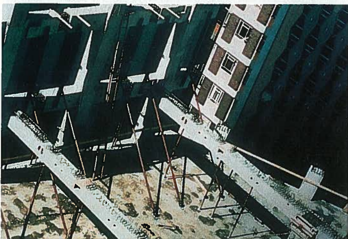
Fig. 16. Construction of the 13-story perimeter frame of Unisys House using two-story high cruciform-shaped precast units (System 3) in Wellington, New Zealand.
