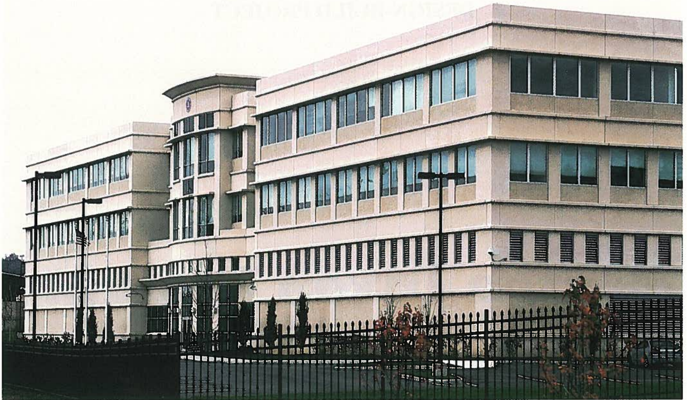
Overview of Martha Dixon Building, Pittsburgh, Pennsylvania. Photographer: Roy Engelbrecht.
