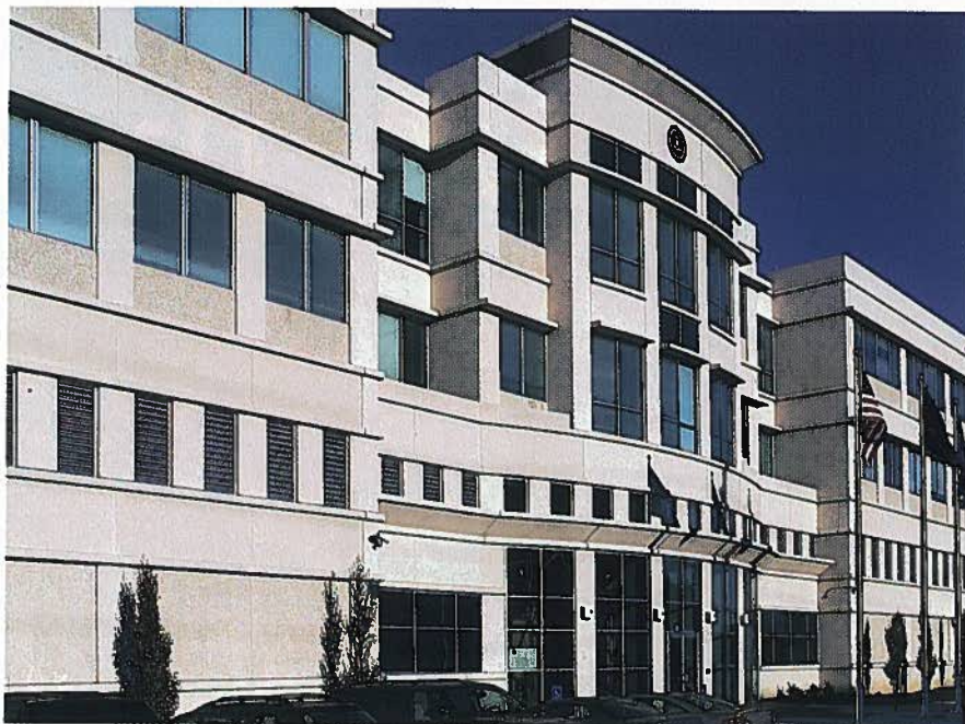
Side view of Martha Dixon Building. Photographer: Roy Engelbrecht.
