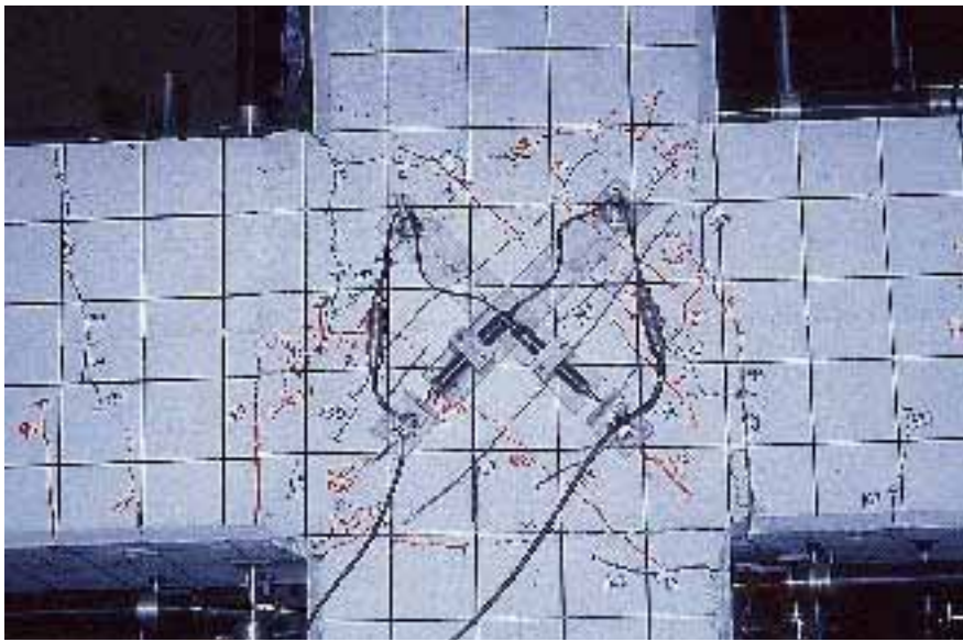
Fig. 7a. Joint damage of Specimen J1 at design drift of 2 percent.
