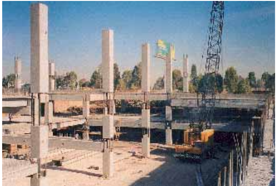
Fig. 1. Type of precast concrete frame construction studied.
