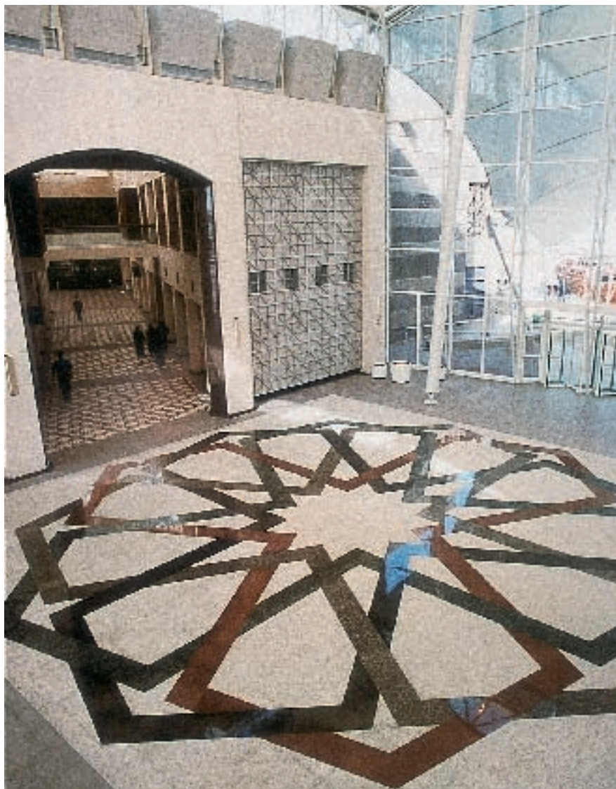
Fig. 13. Stone and tile were used on the floor and at the base of the walls, joining architectural precast panels that continued to the roof. Courtesy: Gustavo Ferrari.
