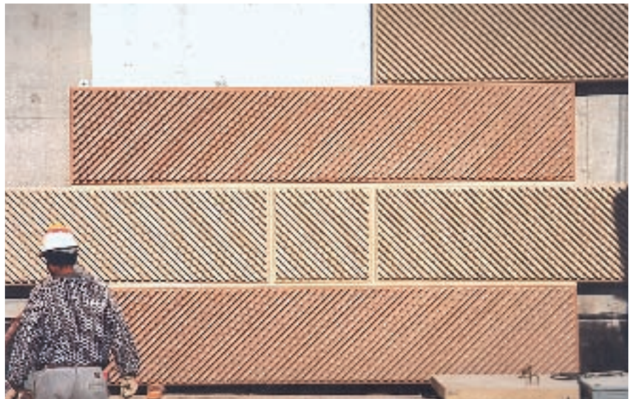
Fig. 5. The precast concrete walls were cast in alternating bands of color and diagonal ribs to emphasize the changing light patterns during the day.
