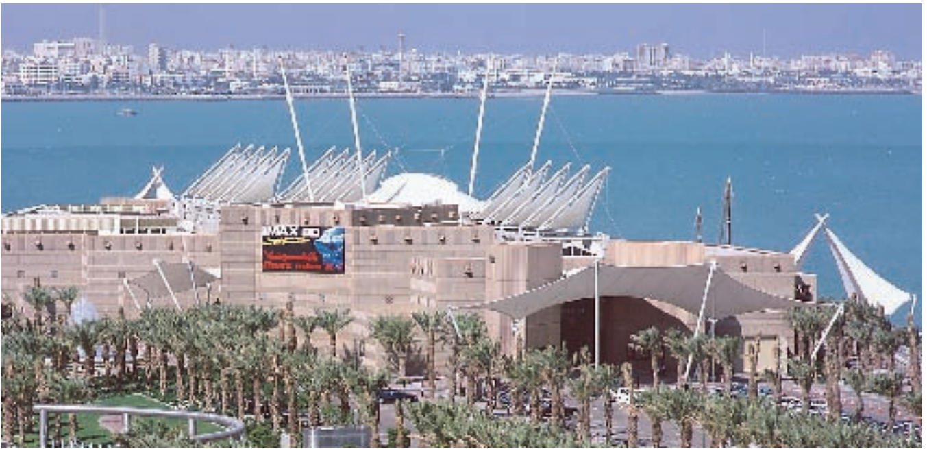
Fig. 1. The architectural and structural design of The Scientific Center in Kuwait City, Kuwait, was planned to evoke textures from the desert and the swooping lines of sailboats and nomadic tents. Courtesy: Gustavo Ferrari.
