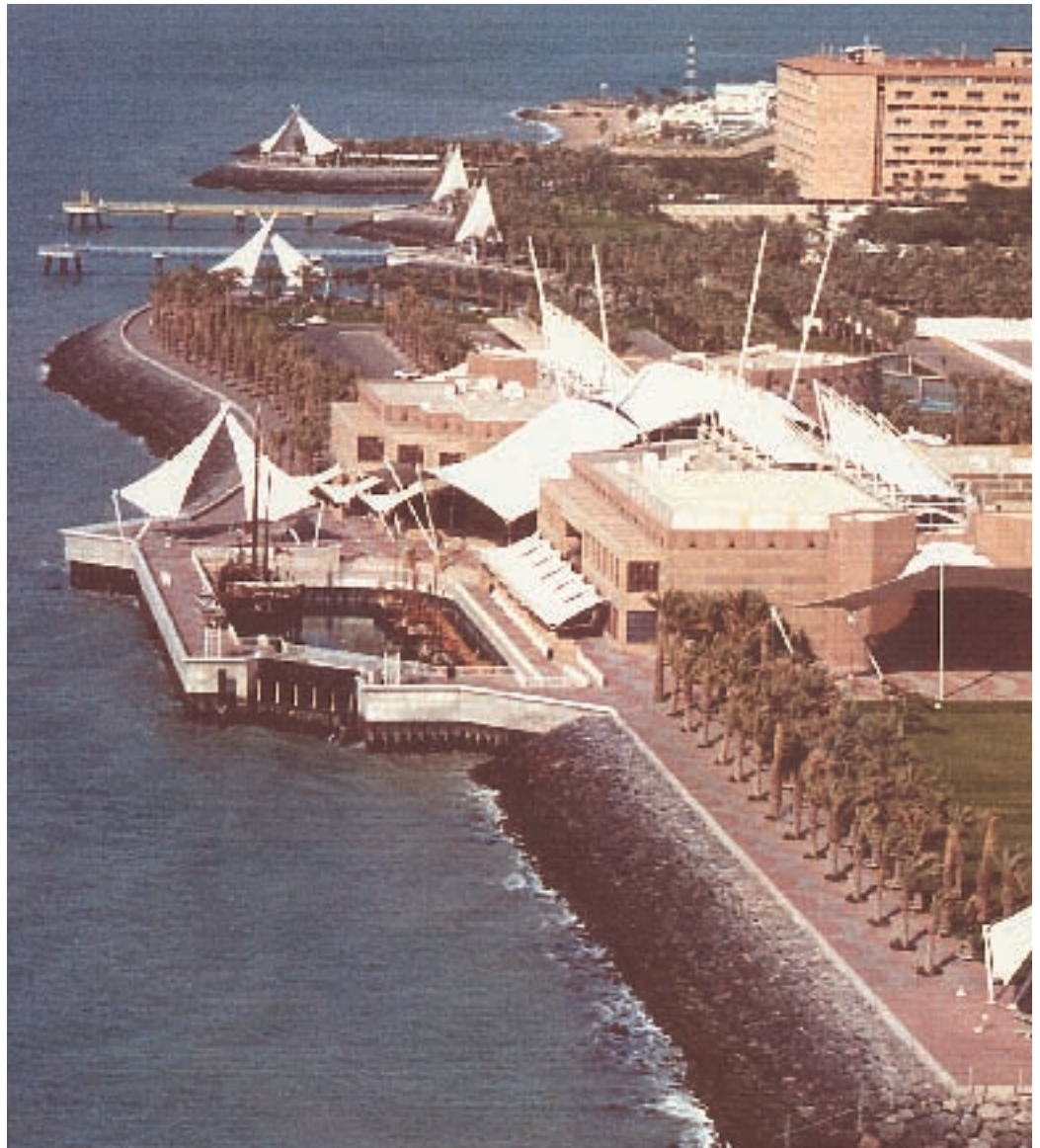
Fig. 17. The retaining wall along the harbor consists of a continuous precast concrete beam that includes a bench for visitors.
