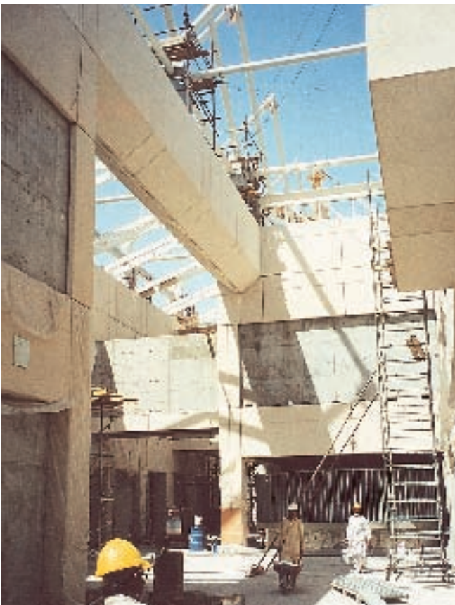
Fig. 11. Slightly whiter precast concrete panels were used on the interior of the two-story exhibition areas to provide better lighting.
