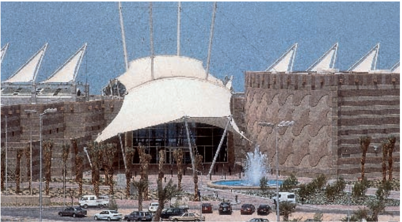
Fig. 8. The north wall features a two-level “wave” pattern made of architectural precast panels in two contrasting colors. Courtesy: Gustavo Ferrari.
