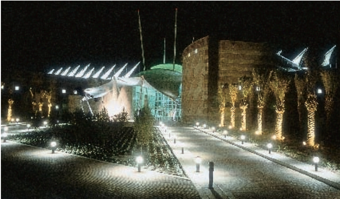
Fig. 4. The Center's dramatic entries overhung with fabric structures become a focal point at night. Courtesy: Gustavo Ferrari.
