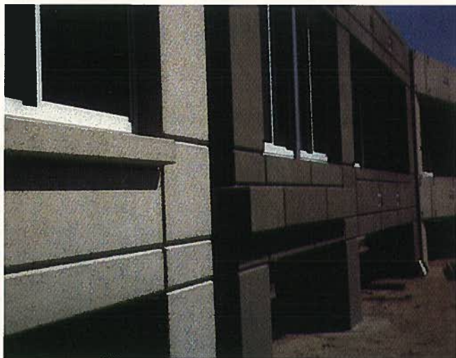
Fig. 18. Mockup of architectural precast panel assembly at precaster's yard.
