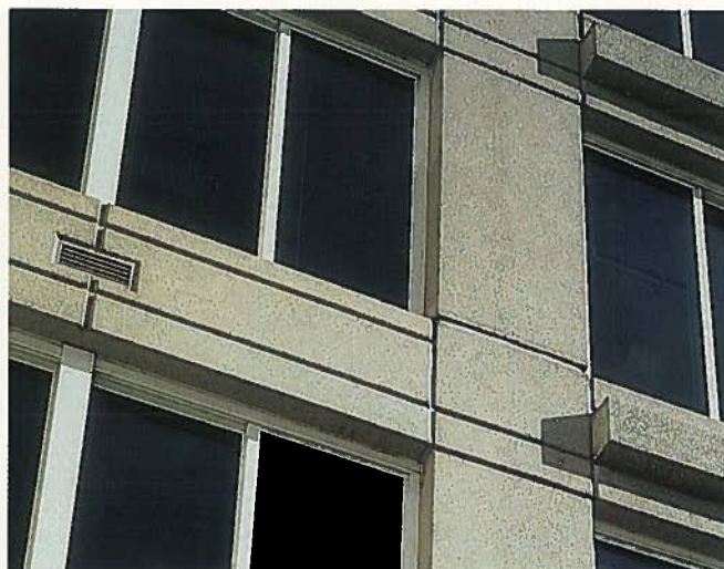
Fig. 19. Architectural precast panel assembly installed on building façade.
