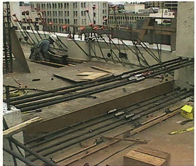
Fig. 9. DDC reinforced frame beam.
