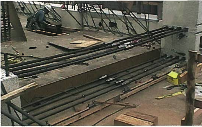
Fig. B3. DDC reinforced beam frame.
