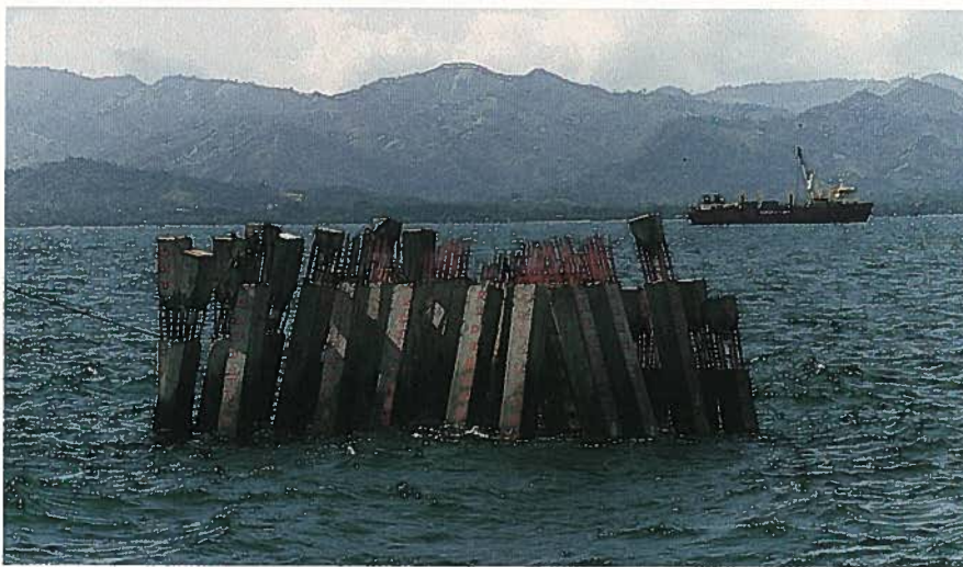
Fig. 7. A view of the piles for a berthing dolphin after being driven into position.
