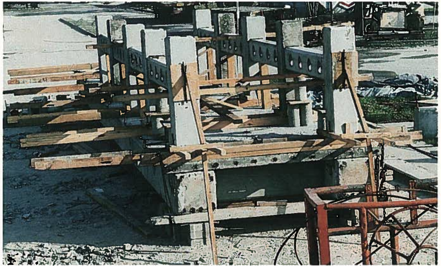
Fig. 19. Partial assembly of the western pedestrian bridge at the precast plant.
