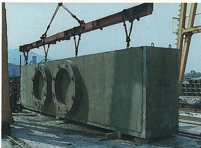
Fig. 12. Front and rear view of "Box 13," assembled at the precast plant from five precast, prestressed concrete panels and reinforcing steel cage for the cast-in-place concrete.
