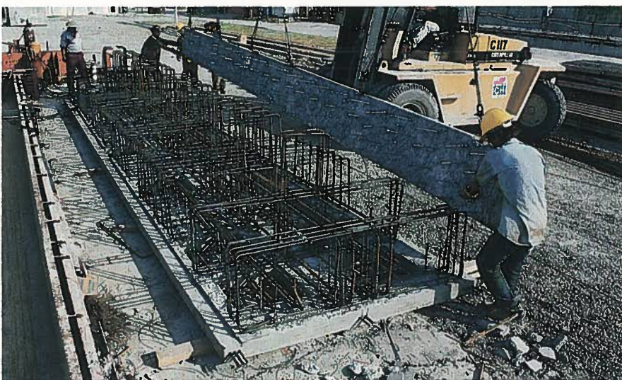
Fig. 15. The precast portion of the pier cap consisted of five individual precast panels that were fabricated and assembled together, along with the reinforcing steel cage, at the precast plant.
