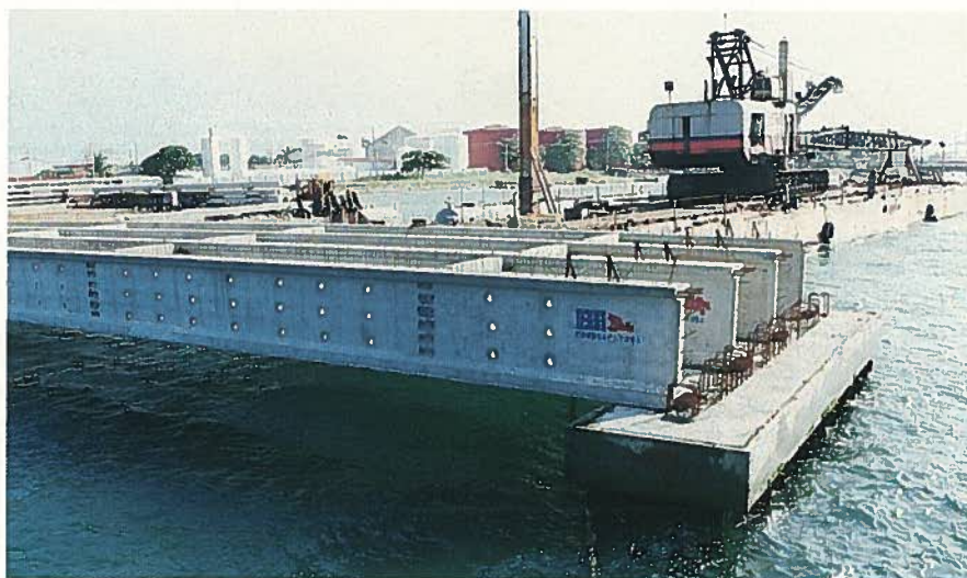
Fig. 17. Precast girders bearing on a completed pier cap.
