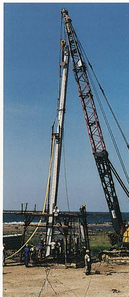
Fig. 5. A precast concrete pile being jettied down into the soil.
