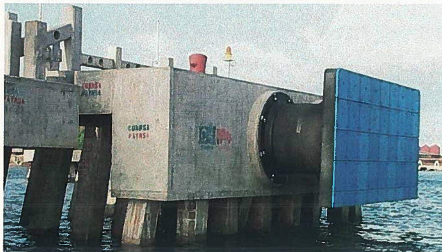
Fig. 13. View of the dolphin system complete with fender and face panel.
