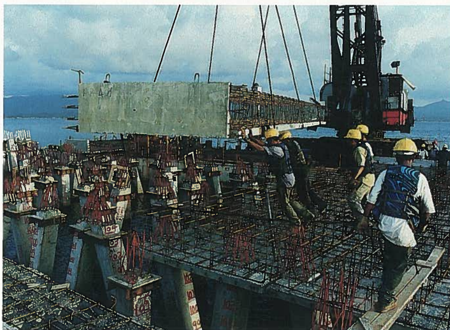
Fig. 10. Positioning one of the precast box units, with reinforcing steel cage, over the precast concrete piling of the operations platform.
