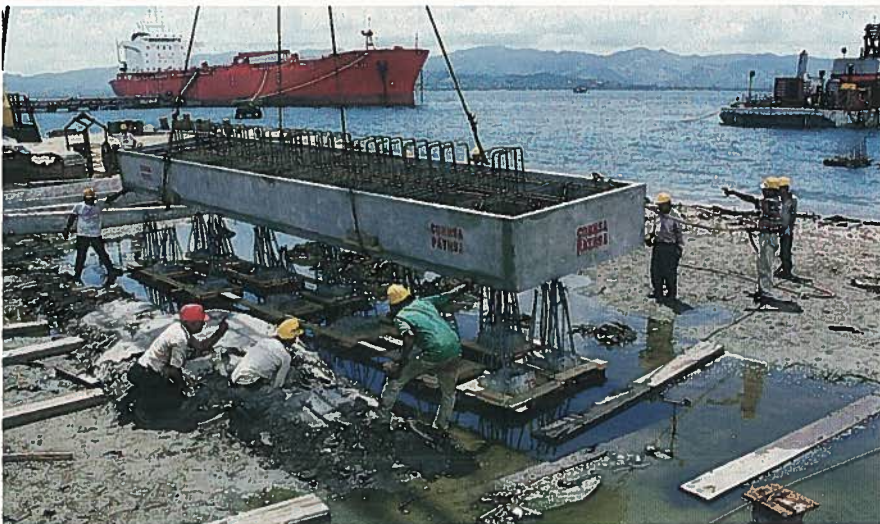
Fig. 16. A precast pier cap box unit being lowered into position atop the precast piling. Note the extension of reinforcement from the top of the pier cap.
