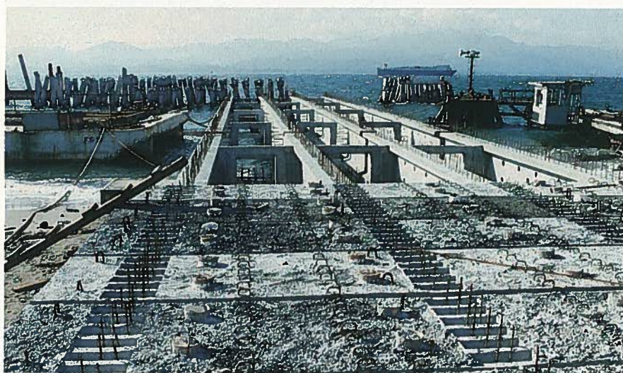
Fig. 18. A longitudinal perspective of the access bridge, showing the precast girders, diaphragms, and deck panels. Note the projection of reinforcement from the top of the girders into the deck topping.
