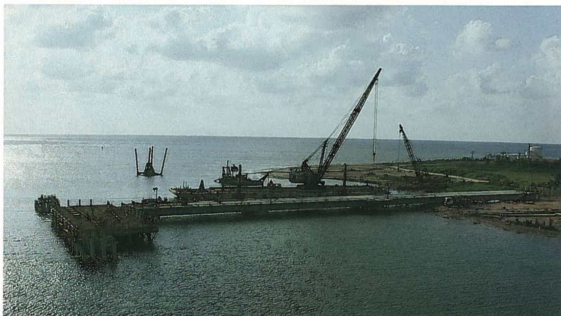
Fig. 1. Construction in progress on the Texaco Wharf Maritime Port Facility, Puerto Cortés, Honduras. A total of 533 precast concrete components were used on the project.
