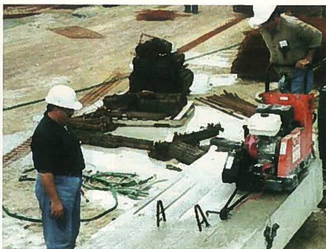
Fig. 3. Cutting grooves for near surface mounted CFRP bars.
