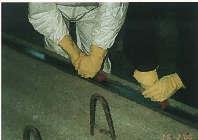
Fig. 5. Bonding CFRP strips to surface.
