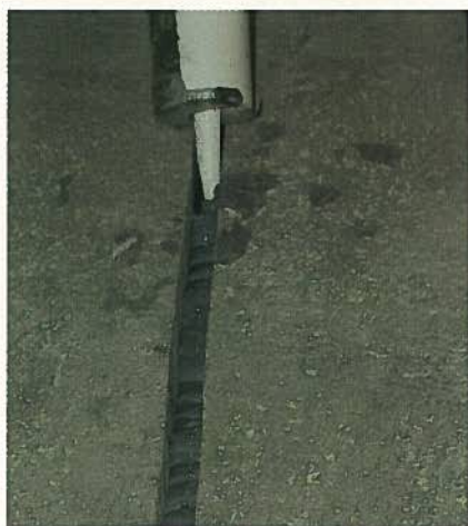
Fig. 6a. Filling grooves with epoxy.
