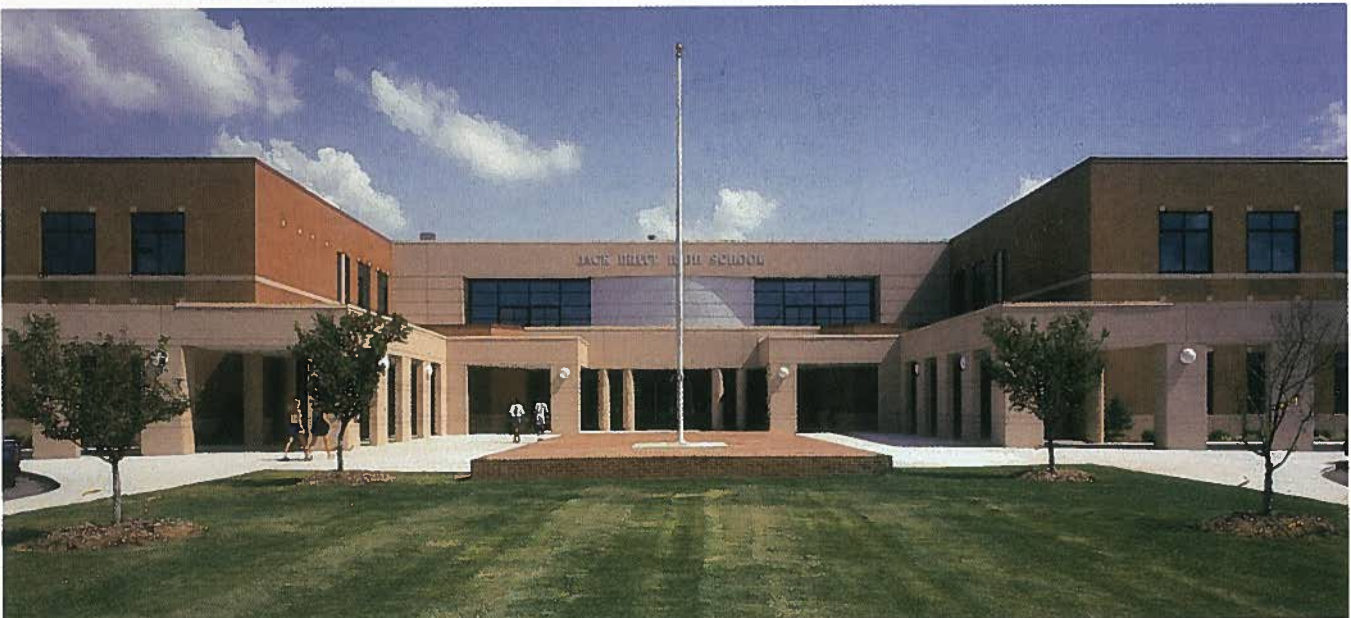
Fig. 1. The precast concrete panels with thin-brick veneer gave Jack Britt High School the look and feel of a traditional brick masonry building, but made construction faster and less costly.
