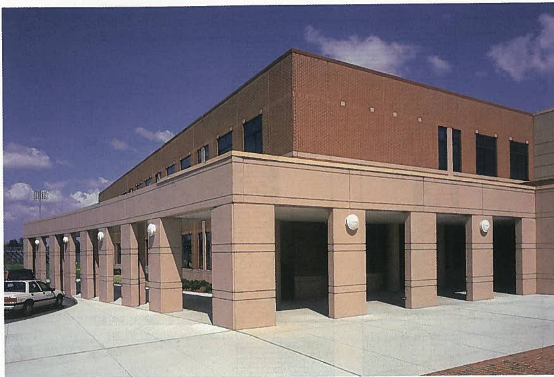
Fig. 3. Sandblasted precast concrete around the building's perimeter (foreground), provided an attractive contrast to the insulated precast concrete wall panels with thin brick (background).
