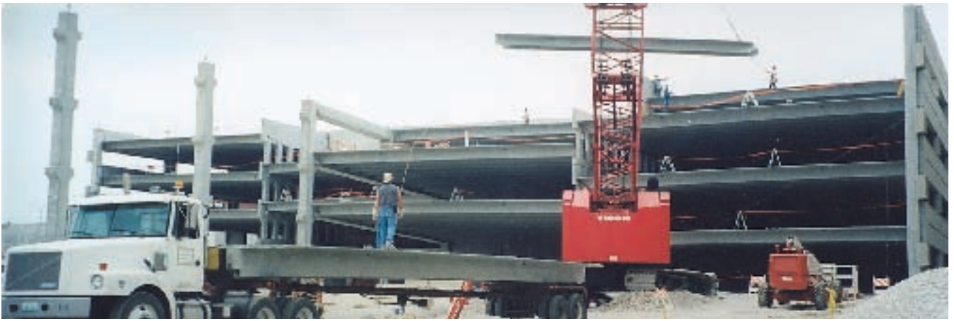
Fig. 17. Overview of erection of precast parking structure.
