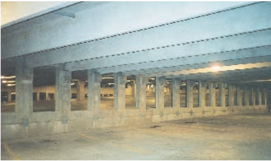
Fig. 6. Interior litewalls allow bay-to-bay ventilation, visibility, and light distribution.
