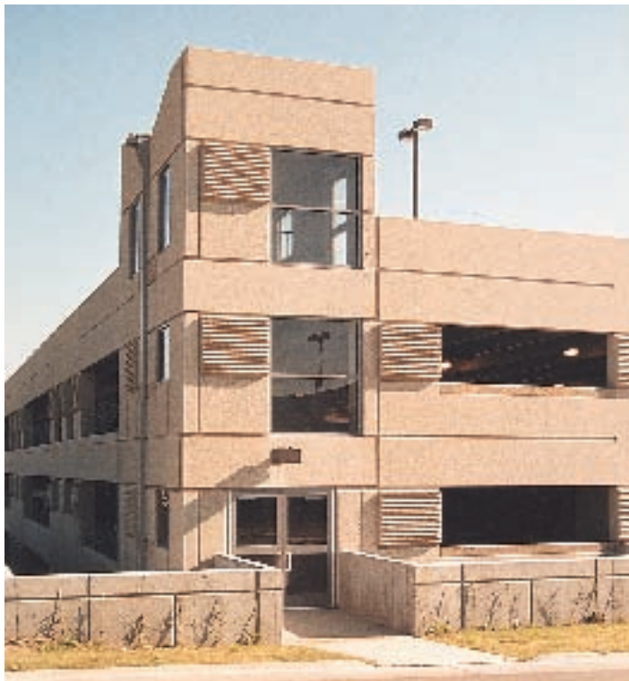
Fig. 3. Ribbed details were used on column covers to add a decorative touch.
