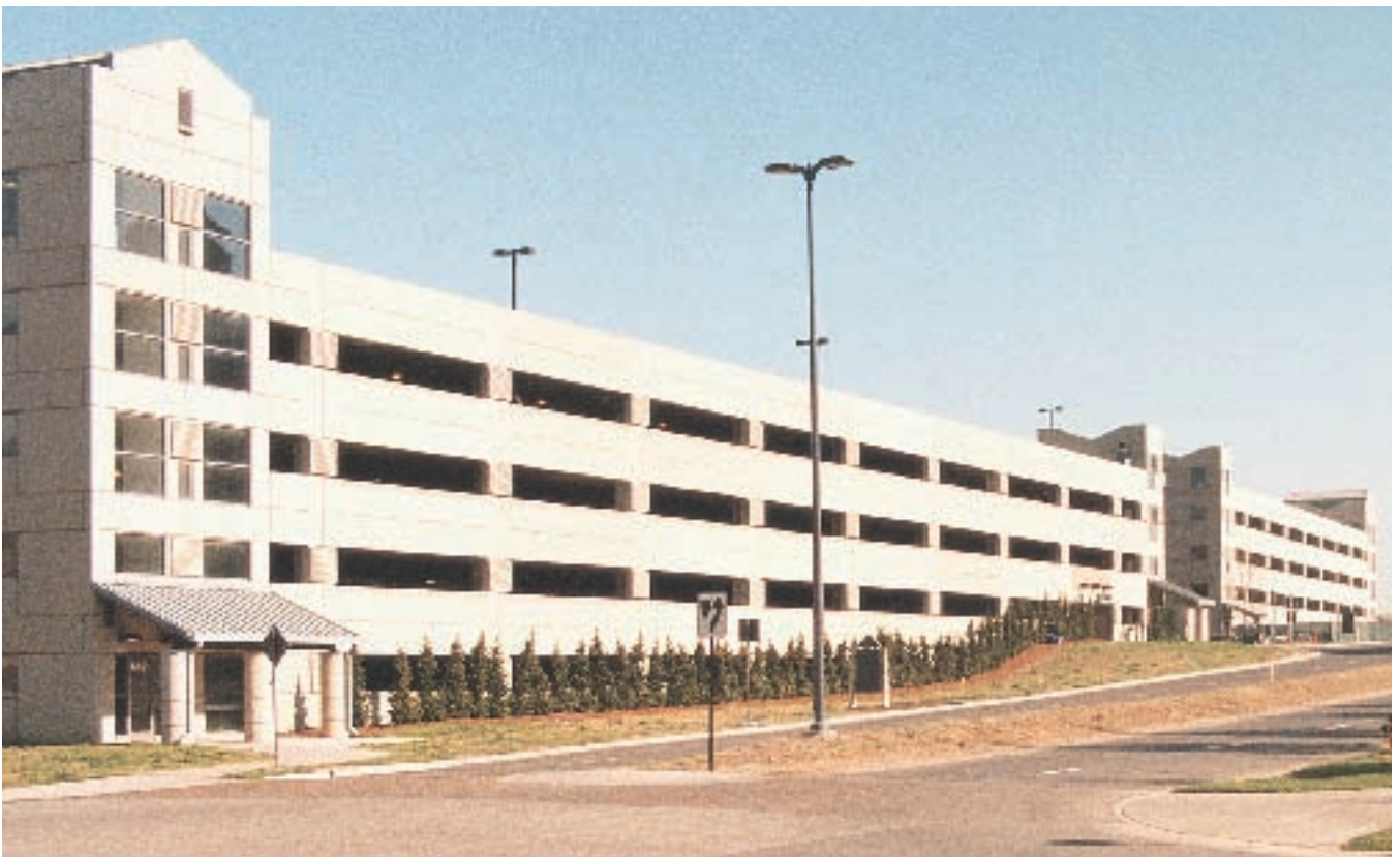
Fig. 18. Finished view of parking structure.
