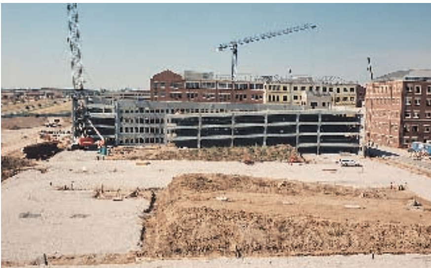
Fig. 16. The site's grade level drops 80 ft (24 m) from side to side, requiring the first floor of each parking structure to be carefully designed.
