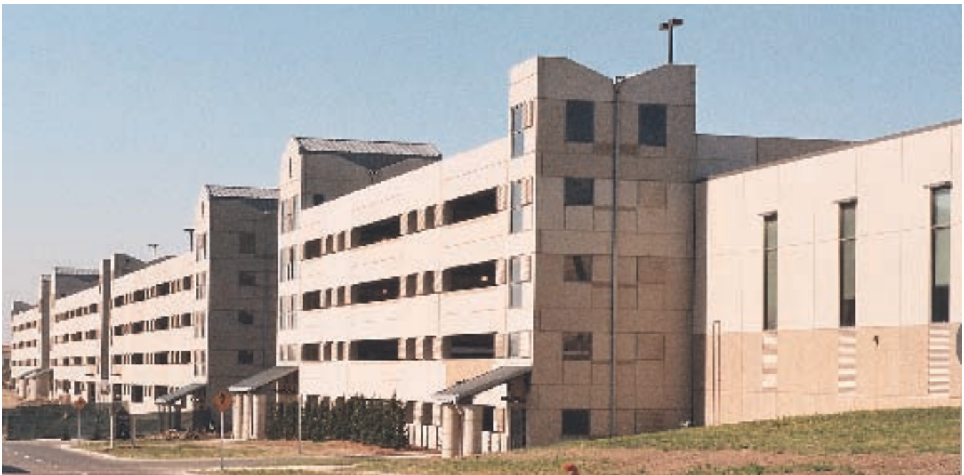
Fig. 13. Reveals, sandblasting, water washing, and a concrete retarder produced accent stripes on the façades.
