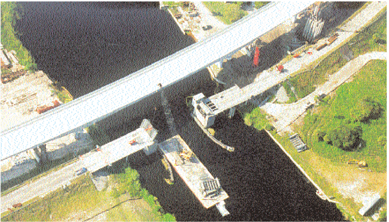
Fig. 20. Moore Haven Bridge nearing completion, Okeechobee Waterway, Florida.
