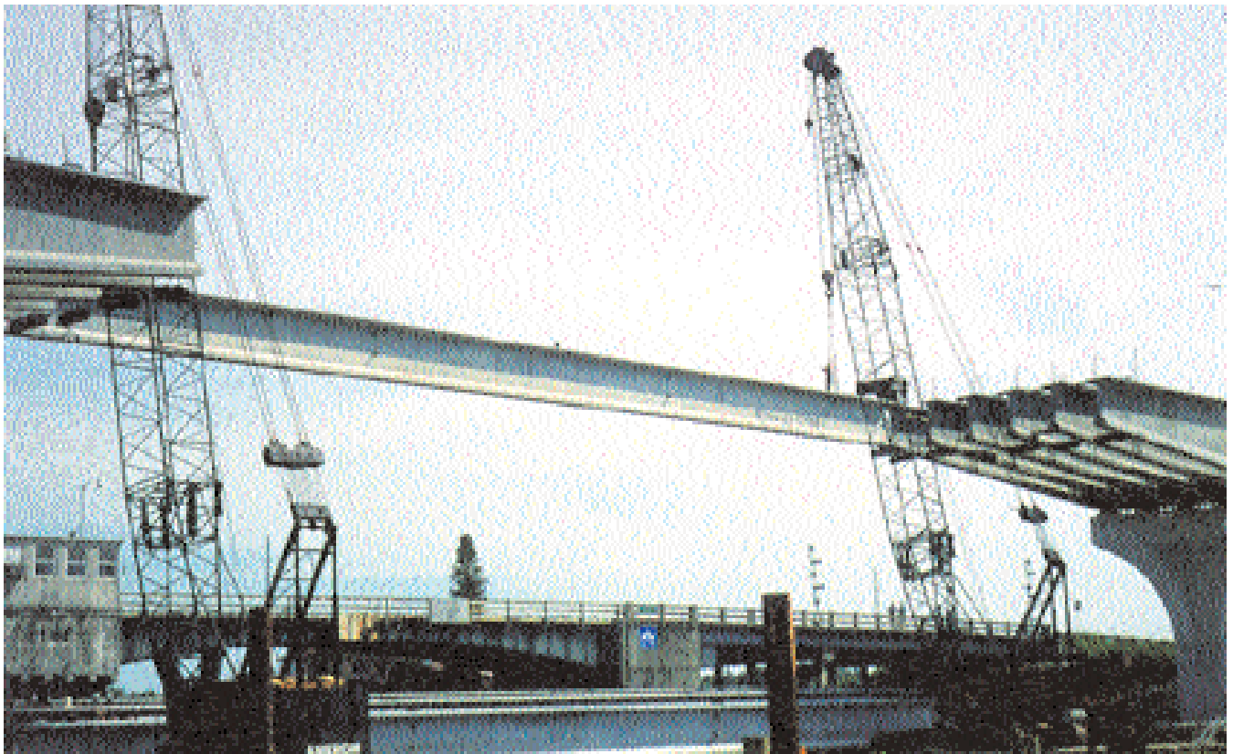
Fig. 18. Drop-in segment erection, Moore Haven Bridge, Okeechobee Waterway, Florida.
