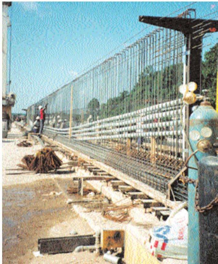
Fig. 16. Drop-in segment fabrication at the Moore Haven Bridge, Okeechobee Waterway, Florida.
