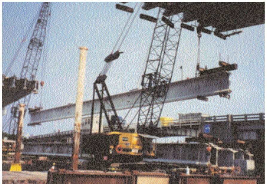
Fig. 17. Drop-in girder with strongbacks attached, Moore Haven Bridge, Okeechobee Waterway, Florida.
