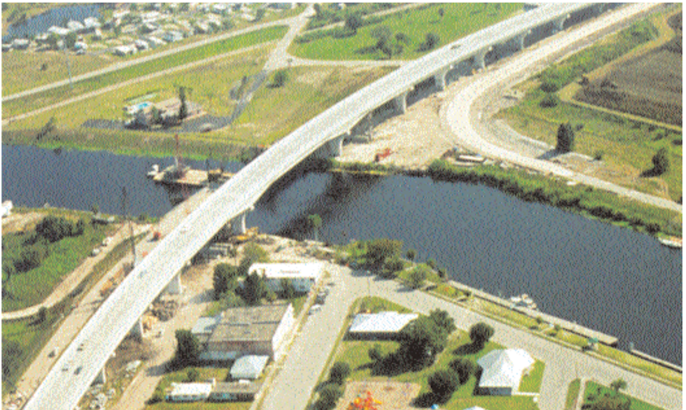
Fig. 1. Moore Haven Bridge over Okeechobee Waterway in Central Florida. At 320 ft (97.5 m), this bridge has currently the longest span using staged post-tensioning. Sverdrup Civil provided construction inspection of this bridge, and the channel unit was designed by Janssen and Spaans.
