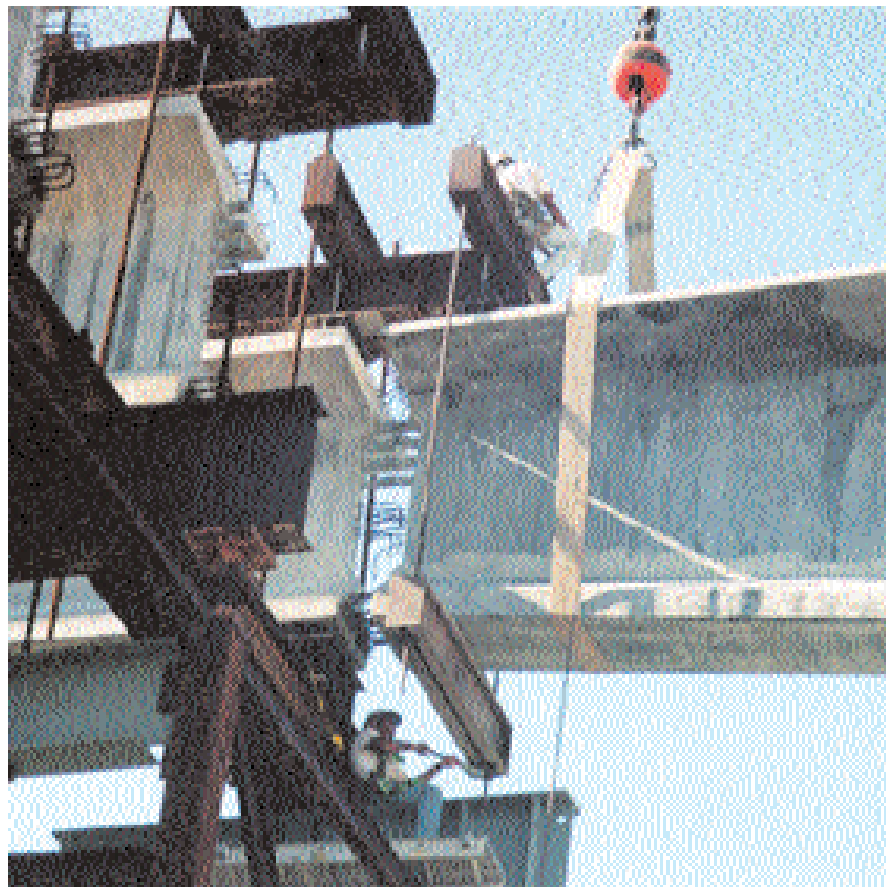
Fig. 19. Strongback installation at closure pour, Moore Haven Bridge, Okeechobee Waterway, Florida.
