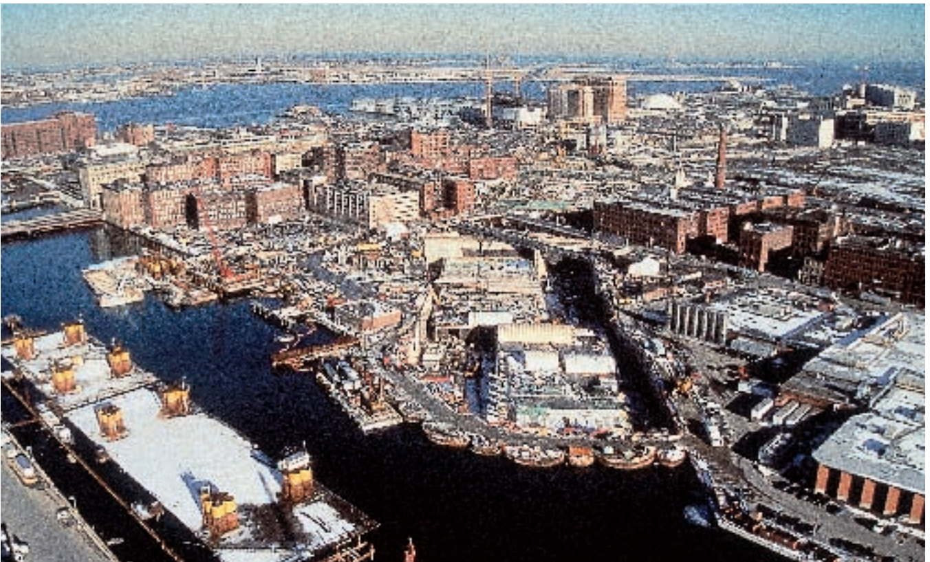
Fig. 6. Precast immersed tube tunnel under construction.
