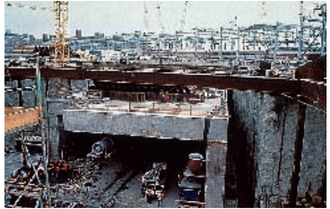
Fig. 5. Precast tunnel jacking.
