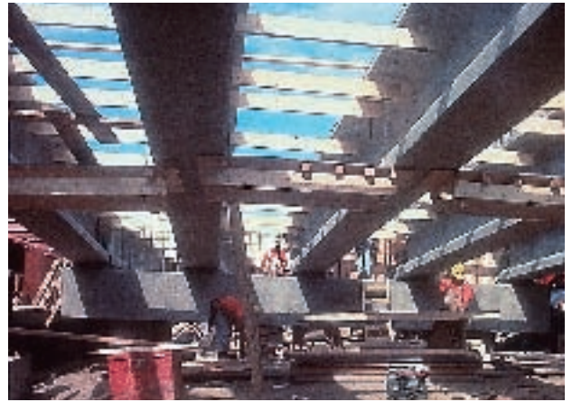
Fig. 12. New England bulb-tee girder construction.
