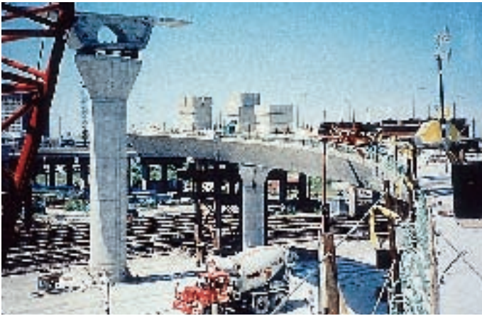
Fig. 11. Segmental concrete construction over North Station tracks.
