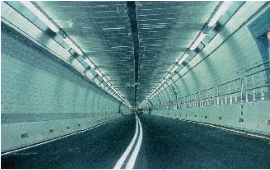
Fig. 7. Ted Williams Tunnel under Boston Harbor.
