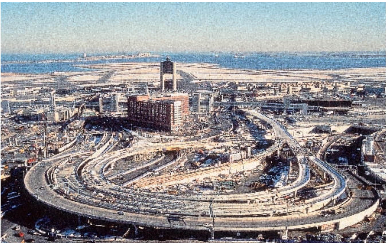
Fig. 8. Logan Airport Interchange under construction.
