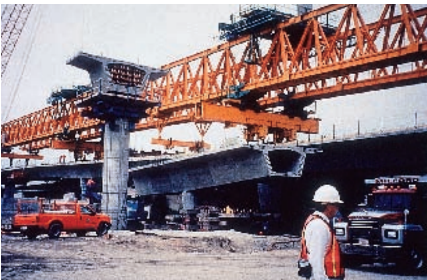
Fig. 3. Precast segmental erection.
