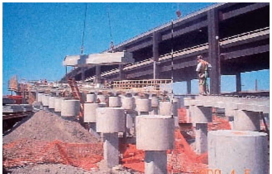
Fig. 13. Slab-on-pile erection.
