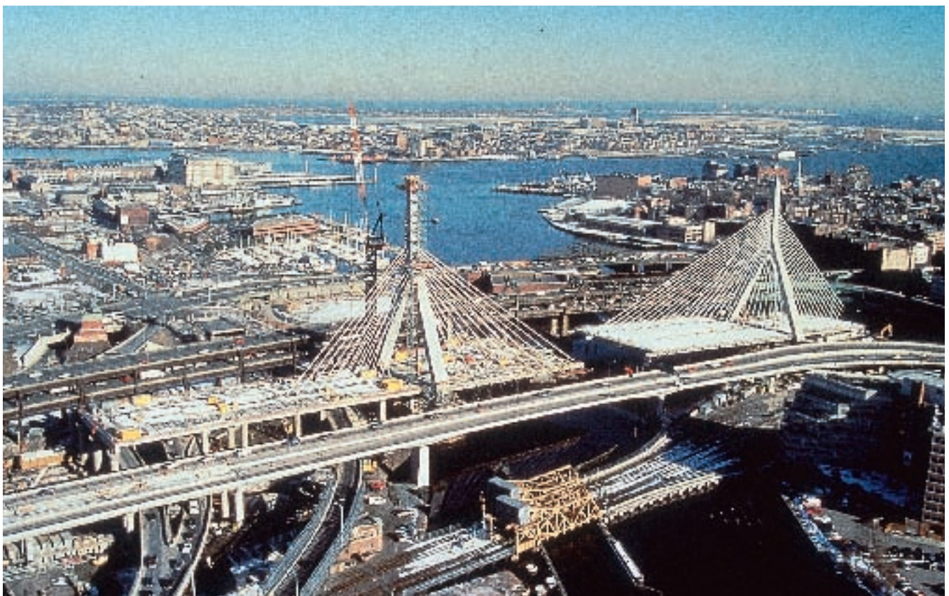
Fig. 10. Leonard B. Zakim Bunker Hill Bridge under construction.
