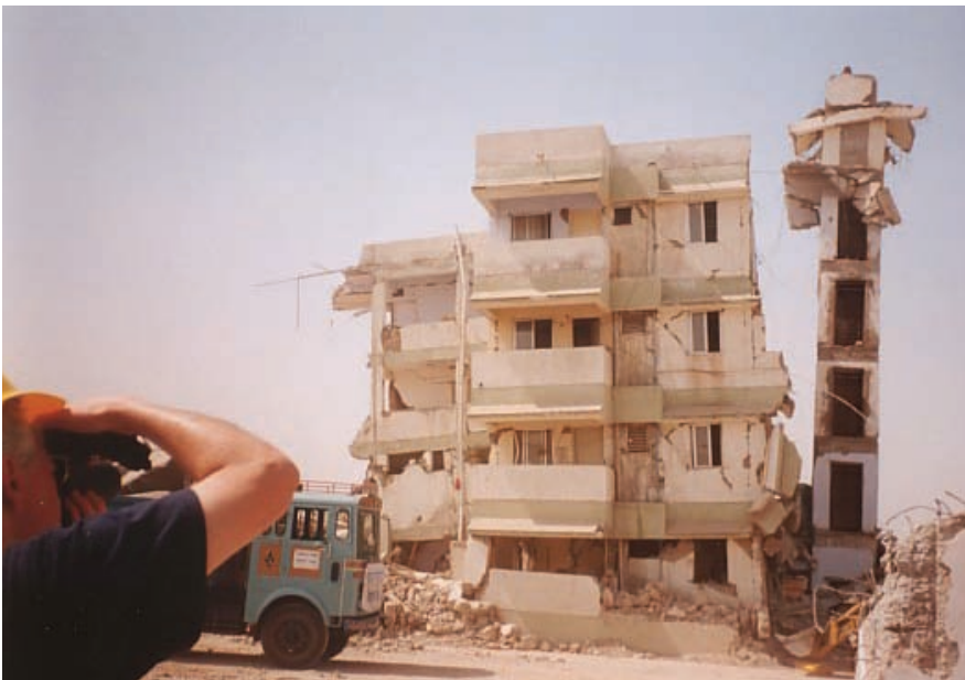
Fig. 10. Core separated from rest of building.
