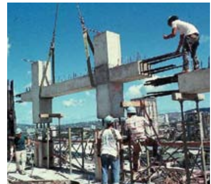
Fig. 17. For the 38-story Ala Moana Hotel in Honolulu, Hawaii, precast column trees were fabricated to support precast floor slabs.
