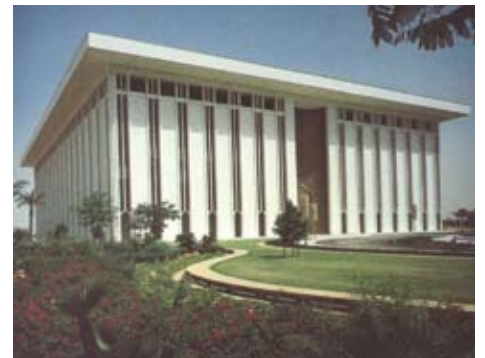
Fig. 4. Headquarters Building, Saudi Arabia Monetary Agency, Riyadh, Saudi Arabia. Precast components include floor beams and slabs, columns, and bearing wall panels.
