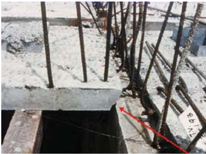
Fig. 10. Reinforcing steel for developing continuity and composite action. (top left) Note that an error in the precasting length resulted in the slab soffit not bearing directly on the precast wall as originally intended. (top right) However, when extended diagonal reinforcing steel is finally bent over the wall support, the composite slab will realize its full intended vertical shear strength without the need for bearing directly on the precast wall. (right) Cross section through wall.
