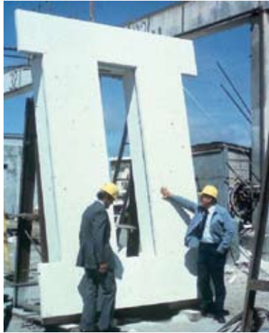
Fig. 16. The 22-story building at 100 Washington Square in Minneapolis, Minnesota. Precast panels were joined horizontally and vertically to form Vierendeel wall trusses.
