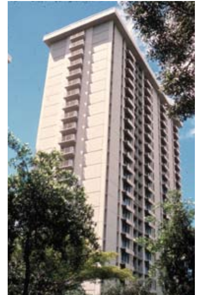
Fig. 2(b). The completed structure with precast façade walls, sunshades, and roof parapets.
