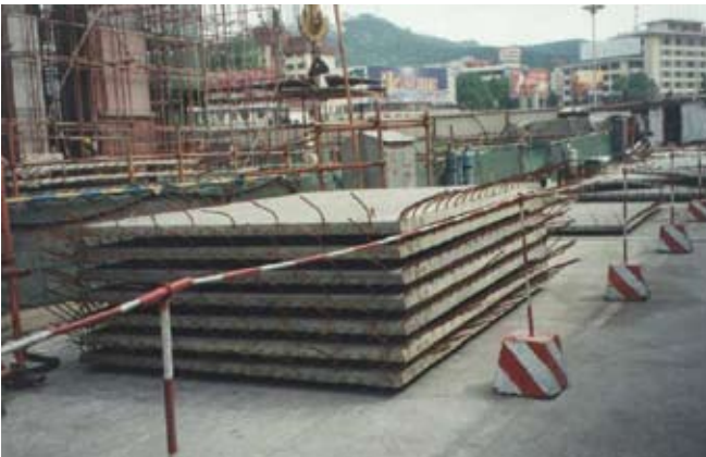
Precast slabs that receive composite cast-in-place topping.
