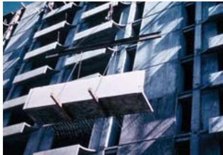
Fig. 2(a). Lifting roof parapets into place on the Queen Emma Gardens building in Honolulu.
