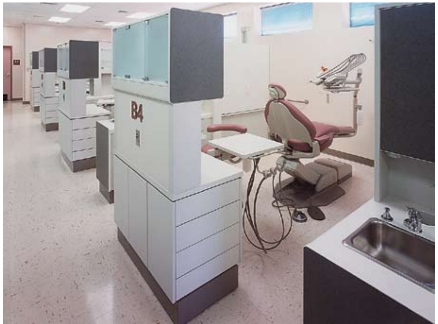
Fig. 10. Long double tees made it easy to lay out the interior medical spaces.
