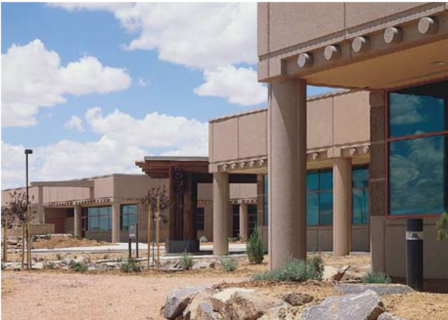
Fig. 8. To blend the facility with the desert environment, a variety of setbacks and corners were created to avoid a monolithic wall design.
