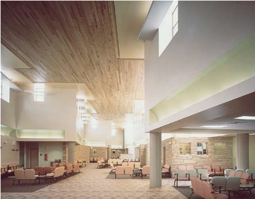
Fig. 12. Light shelves are prominent inside the facility, with daylight reflecting against the wood ceilings.
