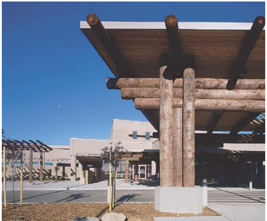
Fig. 15. The medical center's entry features large wood posts along with beams acting as vigas to support an overhead canopy.
