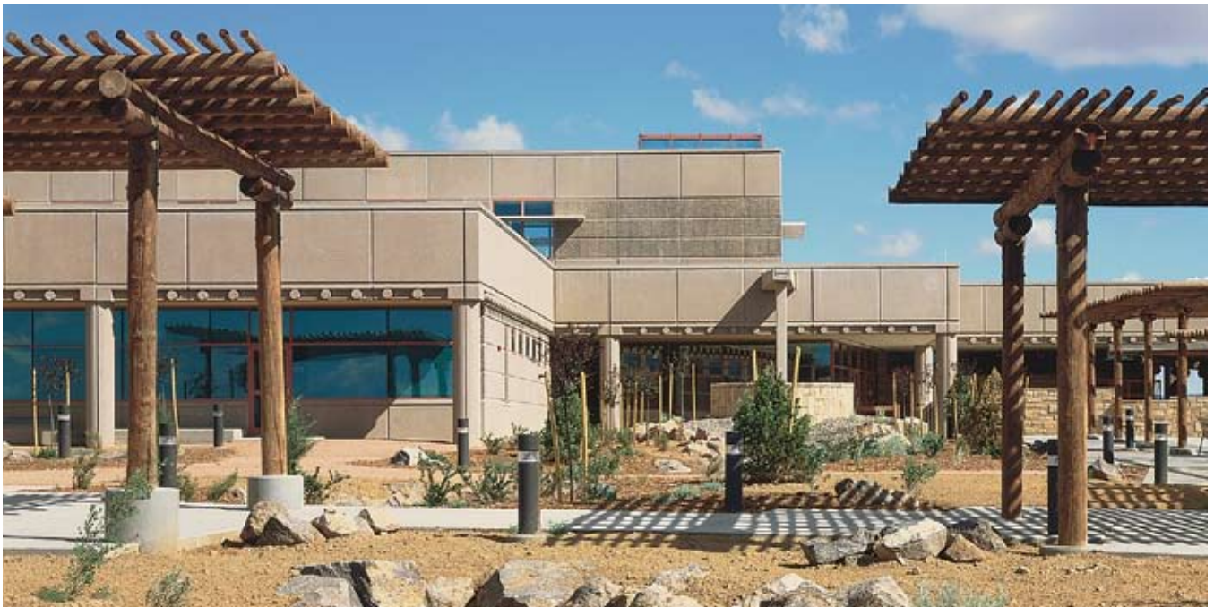
Fig. 1. Elements made of precast concrete, stone, and wood combine to blend the Hopi Health Care Center in Polacca, Arizona, into its environment.
