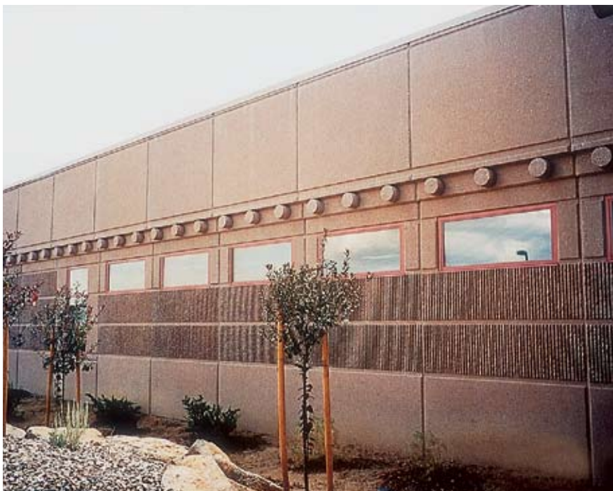
Fig. 4. The precast concrete panels use 5000 psi (35 MPa) strength concrete with an architectural concrete mix that includes imported Rosestone aggregate and dye.
