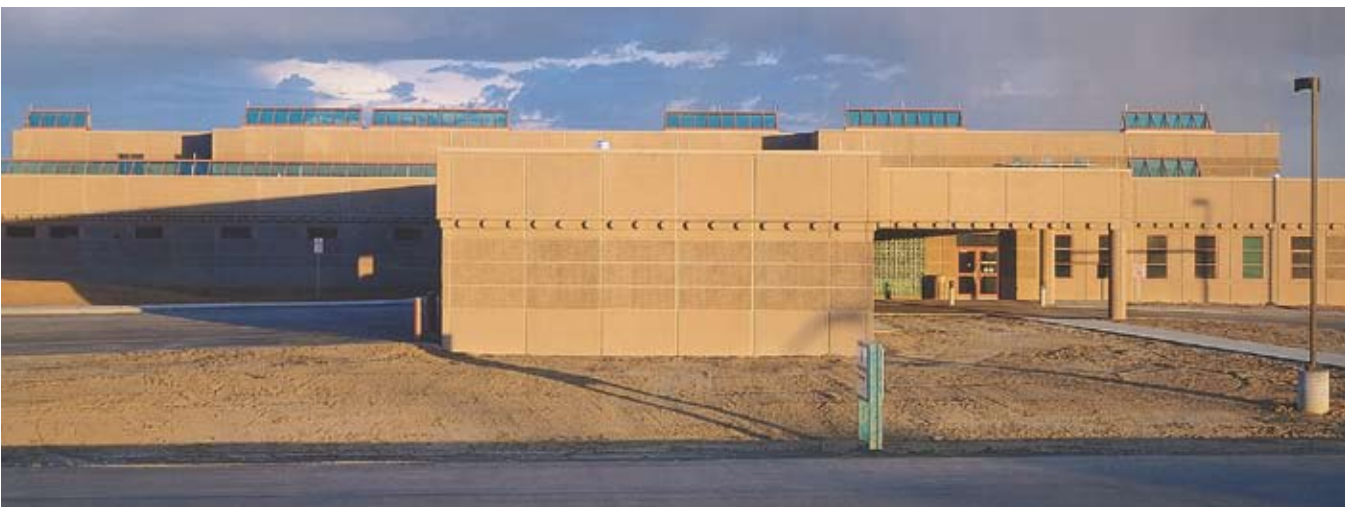
Fig. 19. The variety of corners and overhangs, combined with the viga-like projections on the panels, create a distinctive look for the long, low facility throughout the day.
