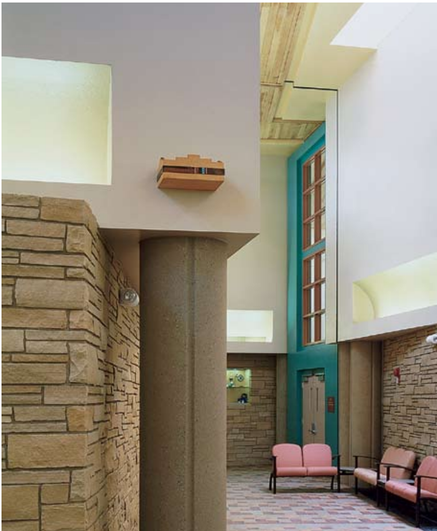
Fig. 17. Precast concrete columns also were used both outside and inside to tie the two areas together.
