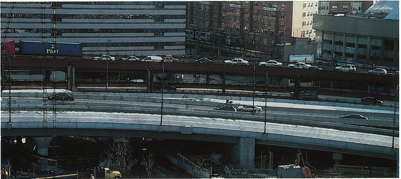
Fig. 8. Initial Leverett Circle Connector – the New England bulb-T girder structure is utilized to raise the roadway to the main bridge structure.
