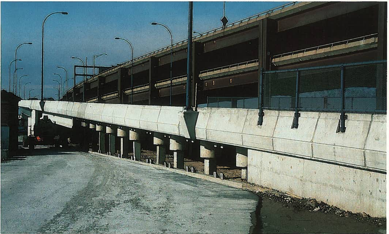
Fig. 1. View of slab-on-pile structure, the New England bulb-T girder structure, and the main steel structure.
