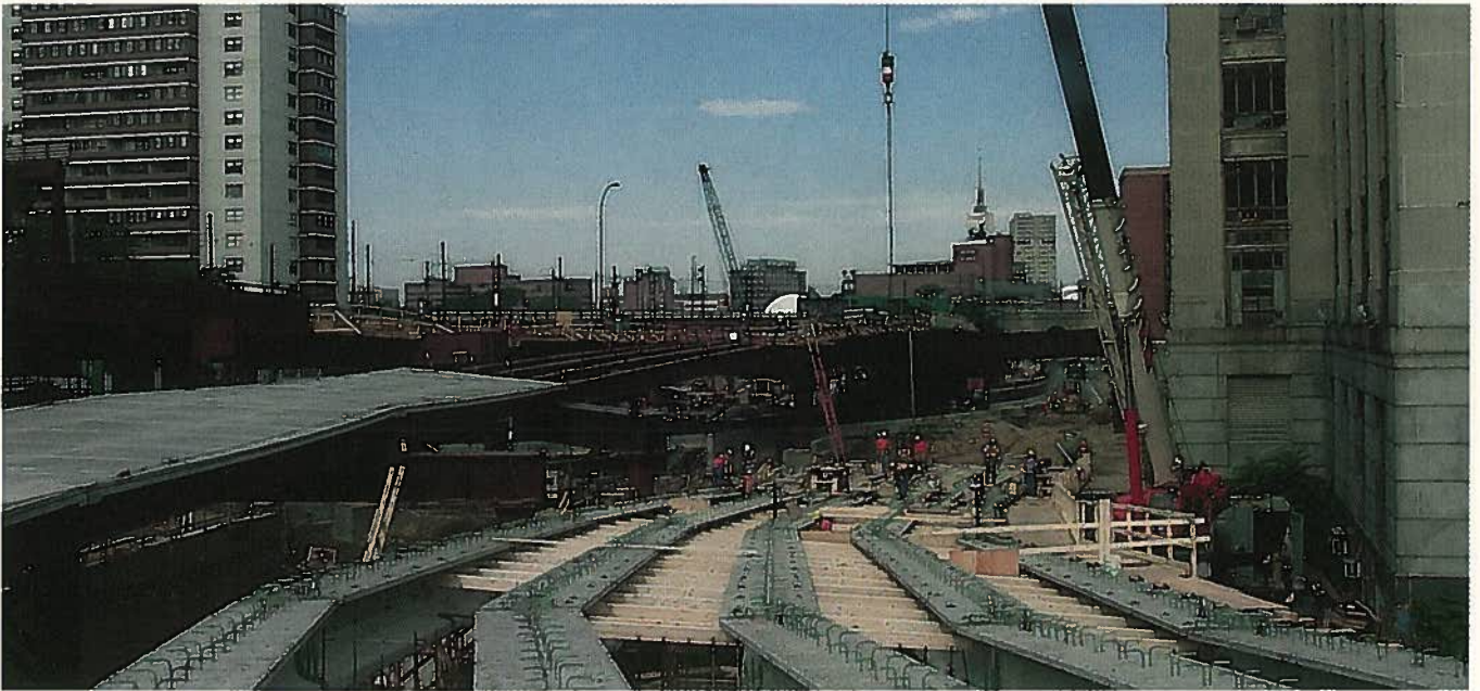
Fig. 6. Framing of the New England bulb-T girder structure.
