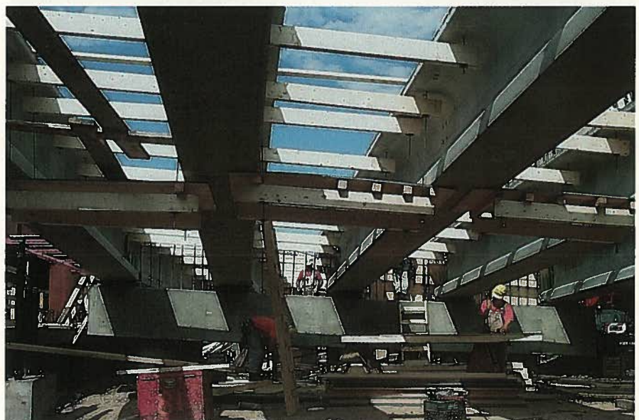
Fig. 2. Preparation of final deck placement for the New England bulb-T girder transition structure. The height of this structure allows for easy inspection and maintenance in the future.
