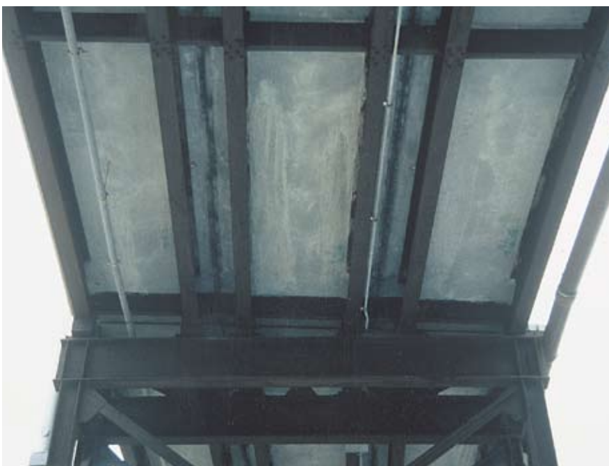
Fig. 4. Underside of bridge showing precast modular Inverset system.
