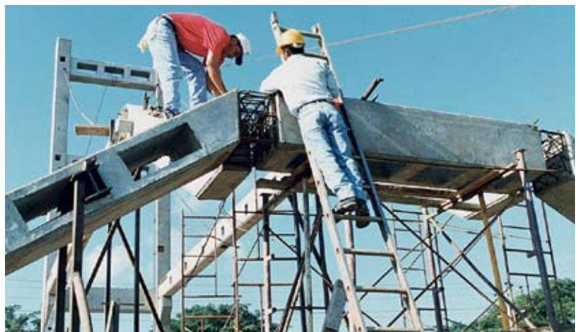
Fig. 20. Wet connection between upper chords of arch and inclined beam.
