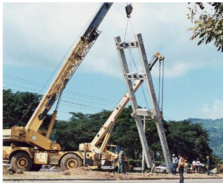
Fig. 8. Erection of H-frame.
