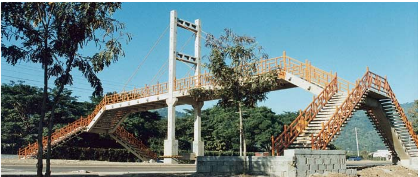
Fig. 2. End view of bridge showing folded arch form in middle and both sides of structure.
