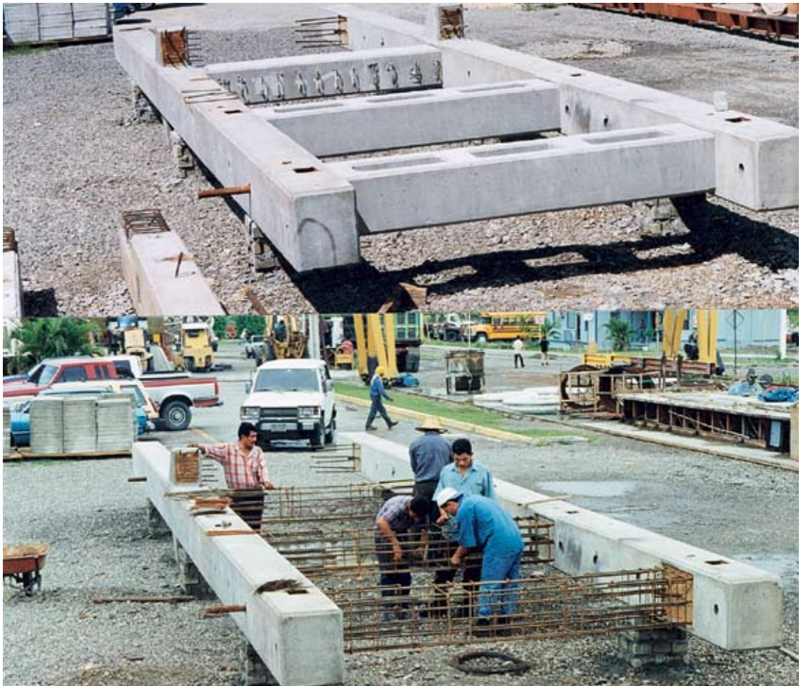
Fig. 22. Fabrication of H-frame in plant.
