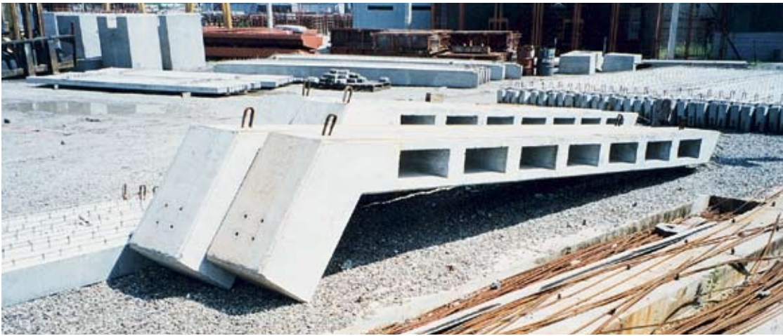
Fig. 23. Upper chord elements in plant.
