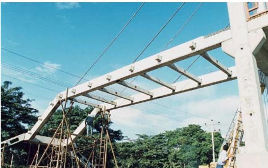
Fig. 11. Main beams and secondary beams in final position.
