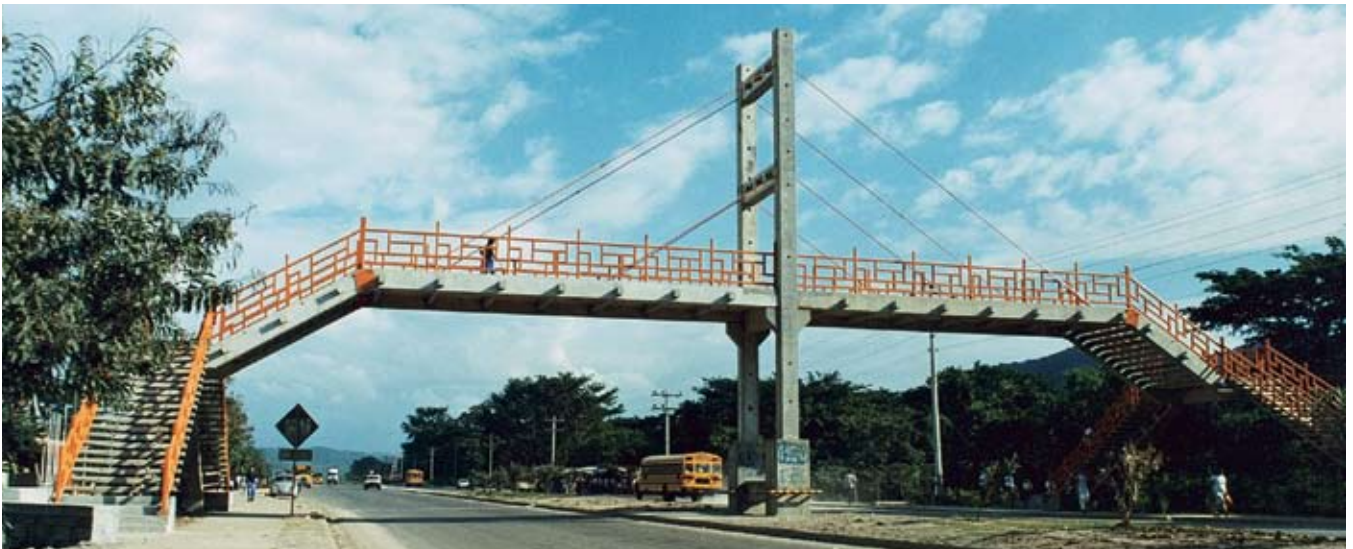
Fig. 1. Completed pedestrian bridge in San Pedro Sula, Honduras. Nearly 150 precast concrete components were used on this project.
