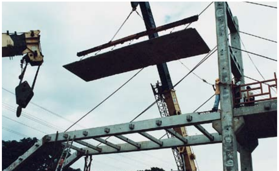
Fig. 13. Deck slab being lifted into place.
