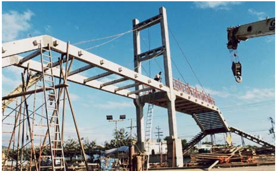
Fig. 12. Four main beams were installed on temporary scaffolding.
