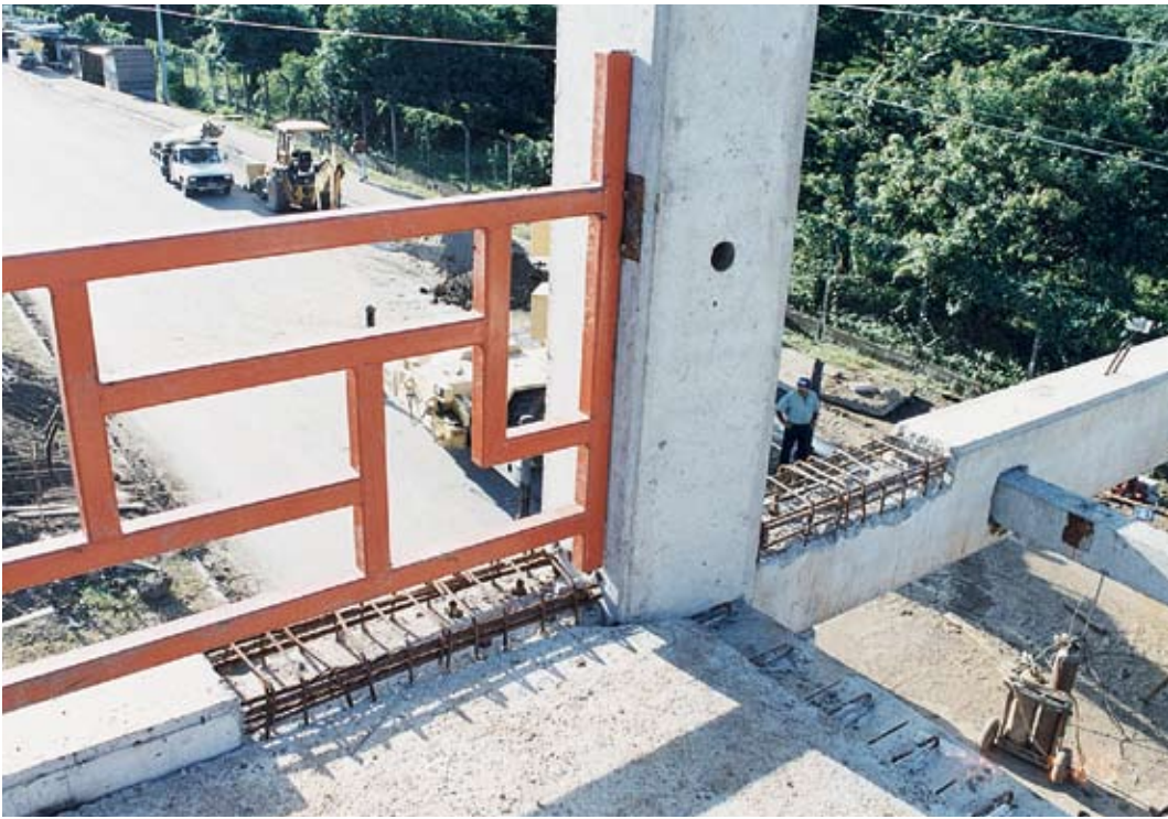
Fig. 17. Column, main beam, secondary beam and deck slab connection during erection.
