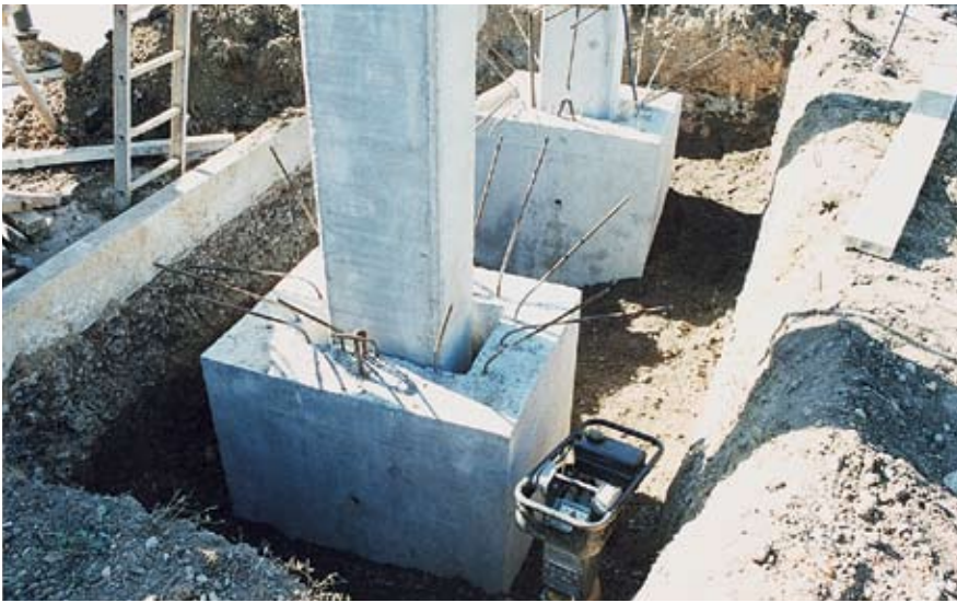
Fig. 9. Precast pocket footing of H-frame in final position.
