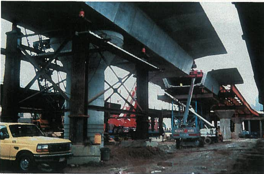
Fig. 8. Segmental concrete construction.
