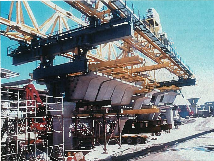
Fig. 10. Segmental concrete bridge erection gantry testing.
