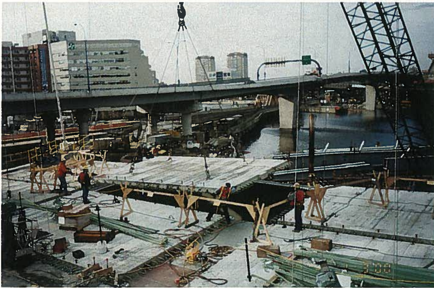
Fig. 2. Charles River Crossing deck slab installation.
