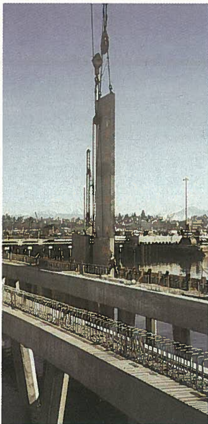
Fig. 16. Close-up view of installation of concrete breakwater panel.
