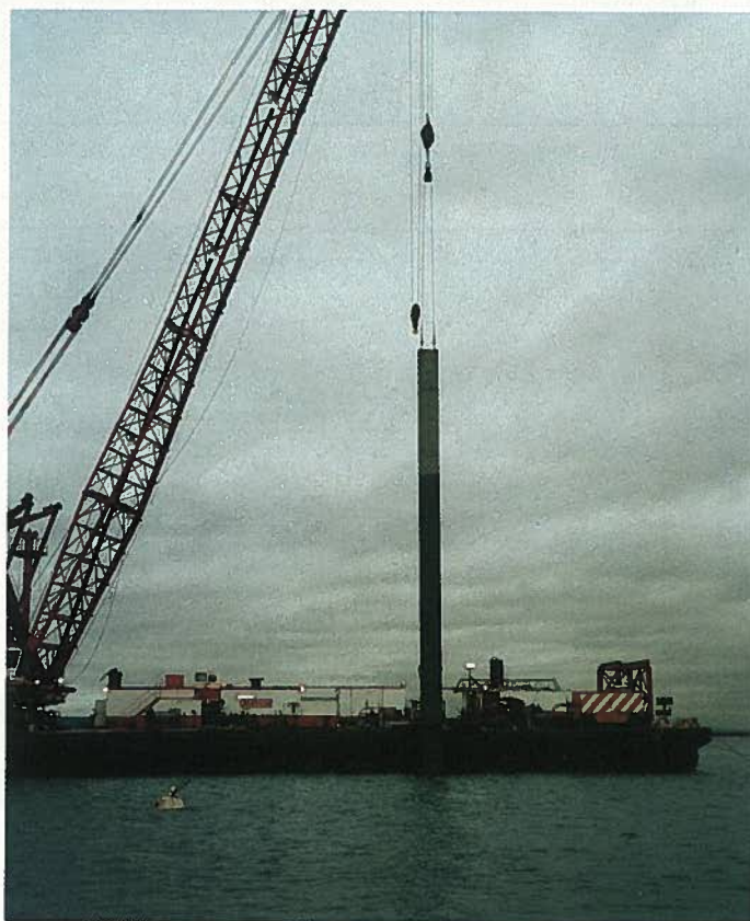
Fig. 15. Precast concrete breakwater panel being lifted into position for placement into template.
