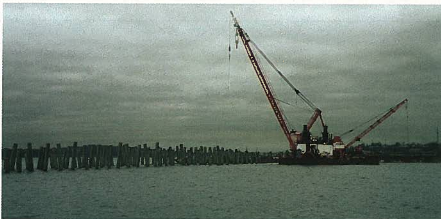
Fig. 14. Installed precast concrete piles.
