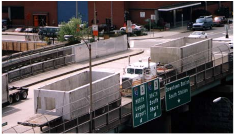
Fig. 9. Trucks transporting panels. Openings are visible in the components for unit heater and window.
