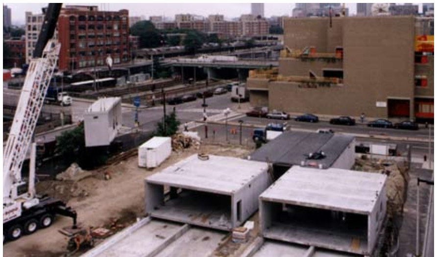
Fig. 11. Erection of a precast concrete modular ring just after it has been rotated for positioning.
