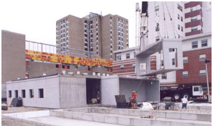
Fig. 10. Erection of a precast concrete modular ring for the classroom section. The administrative area has been erected. Note the opening for the window, unit heater and door in the component being erected.
