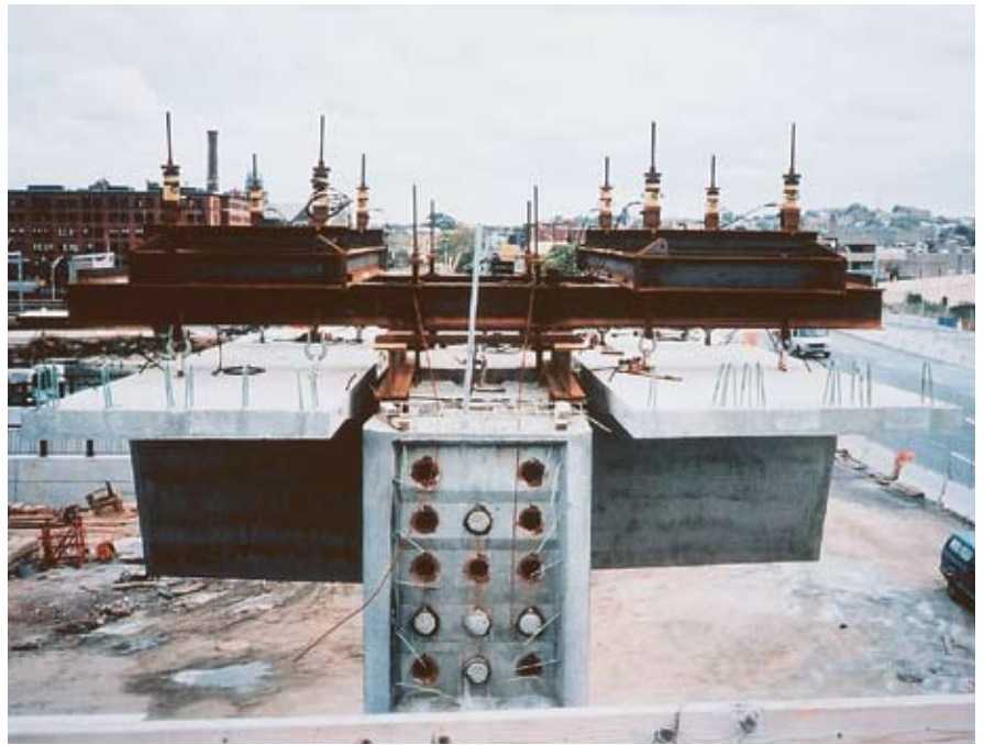
Fig. 12. Precast segment supported at straddle bent.
