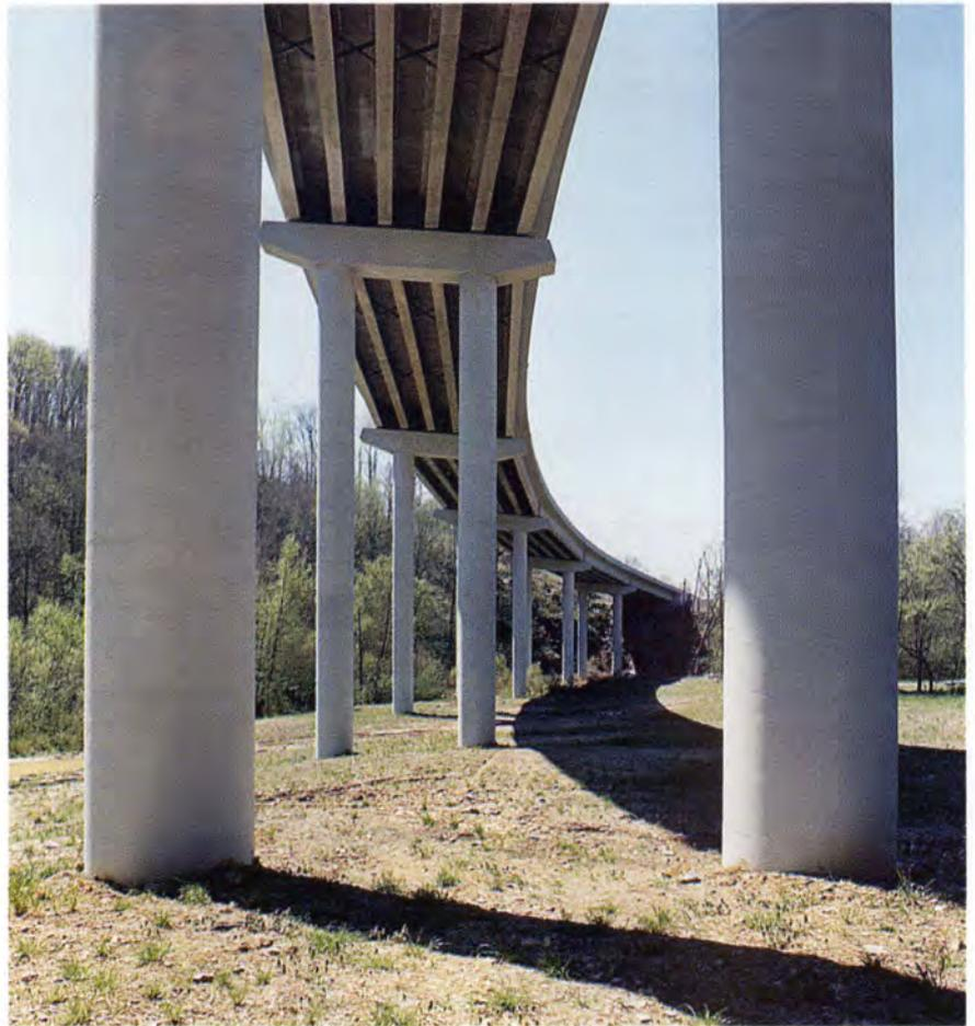
Fig. 10. Underside view of completed bridge showing bent and piers.
