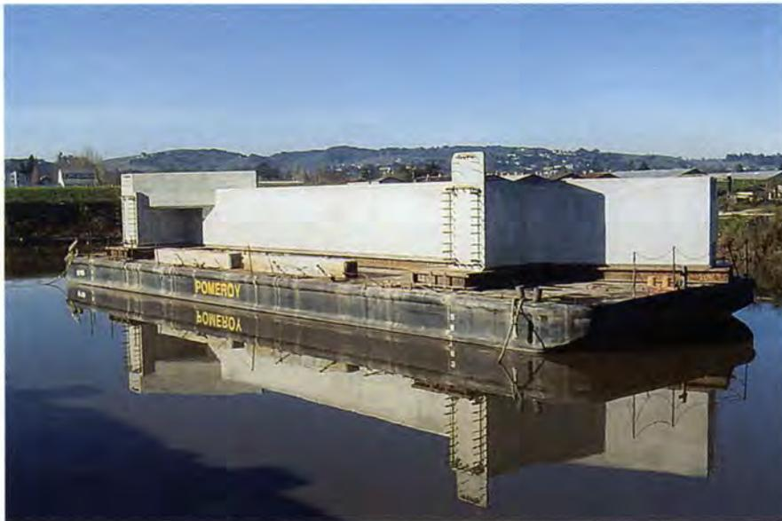
Fig. 4. Completed segment on barge ready for shipping.
