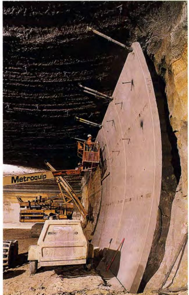
Fig. 4. Precast panels set in place and prepared for grouting.
