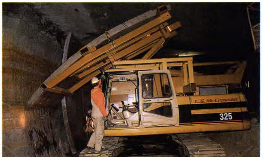
Fig. 2. Precast panel positioned on handling machine (top) and being tilted into position (bottom).
