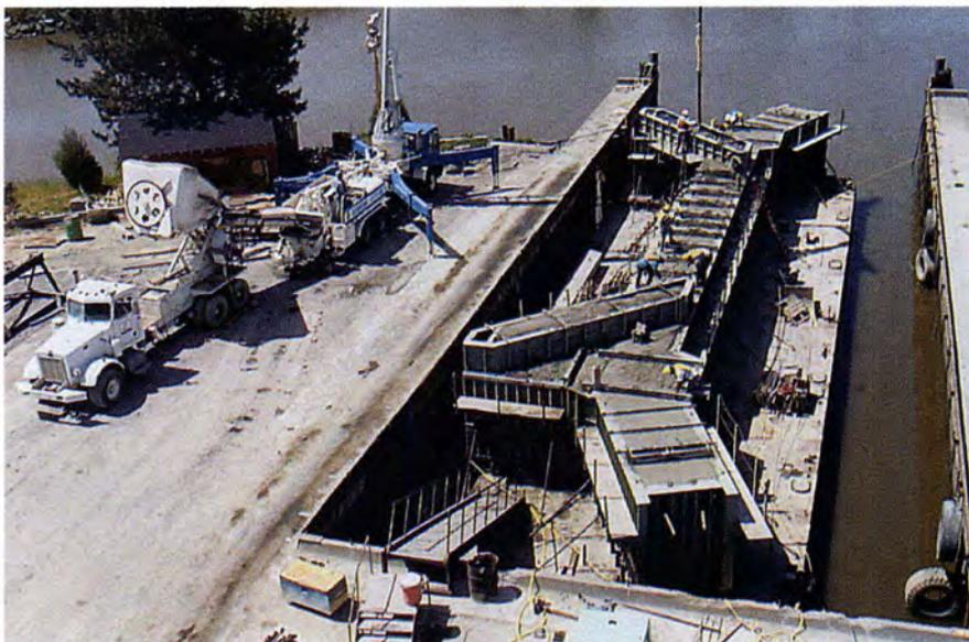
Fig. 3. Casting of segment on barge at precasting plant.
