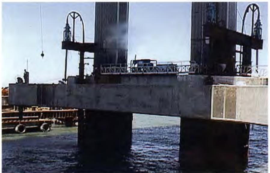
Fig. 5. Lowering completed frame after barge is removed.
