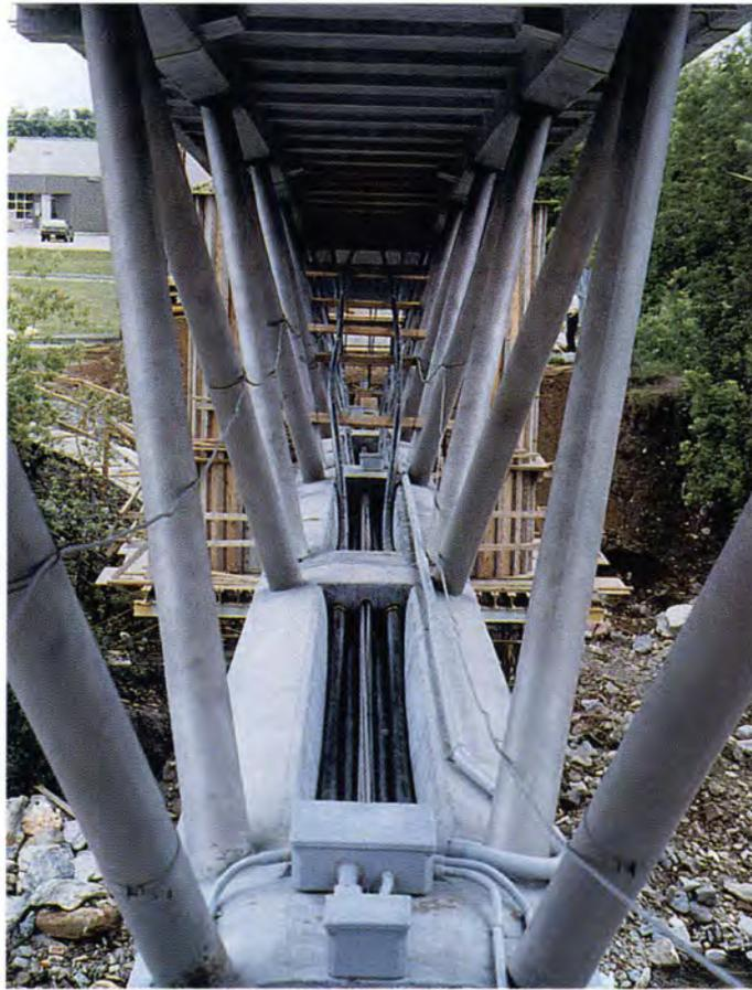
Fig. 17. Permanent external tendons were installed in the bottom chord of the truss, and incrementally tensioned before falsework could be removed.
