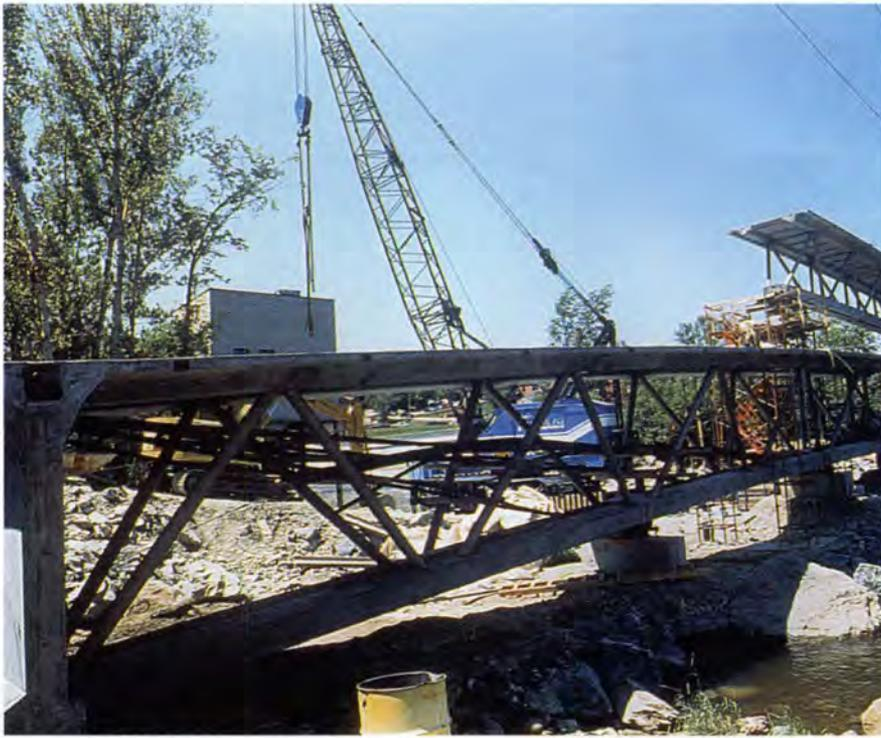
Fig. 15. Half of bridge supported on falsework support (background) awaiting the lifting of a second three-segment portion of truss (foreground).
