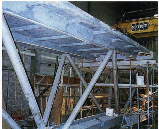
Fig. 12. Bridge segment just after form removal. Configuration of transverse and longitudinal stiffness can be seen.
