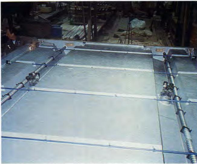
Fig. 9. Formwork for upper deck of bridge, showing location of transverse and longitudinal stiffening beams, with tendon anchors from diagonals positioned in form.
