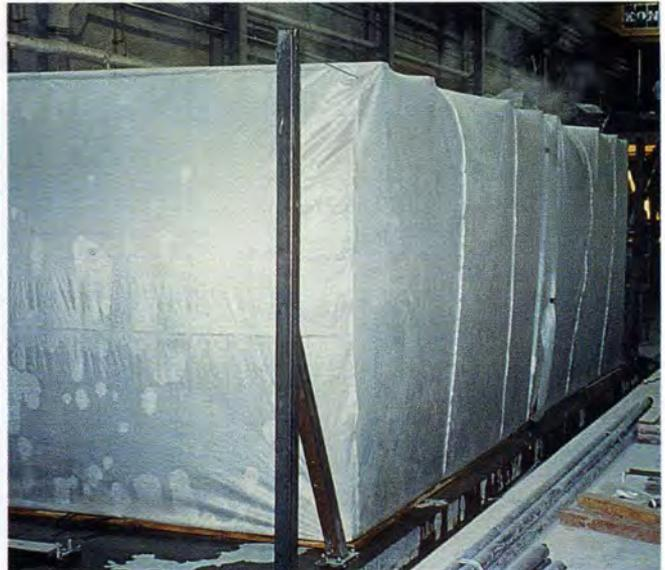
Fig. 11. Segment wrapped in polyethylene for 48-hour curing with hot water vapor.
