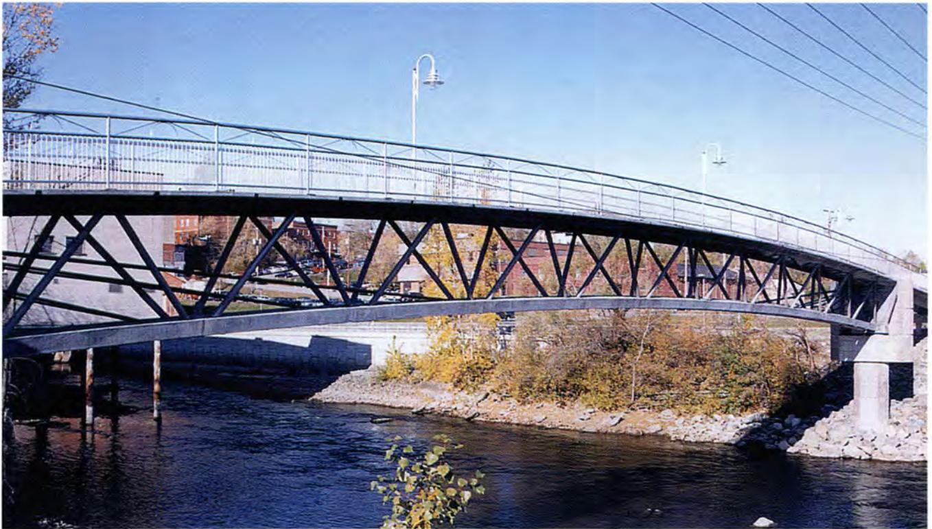
Fig. 1. The Sherbrooke Footbridge in Sherbrooke, Quebec, spans 197 ft (60 m) across the Magog River with a precast truss made of reactive powder concrete.
