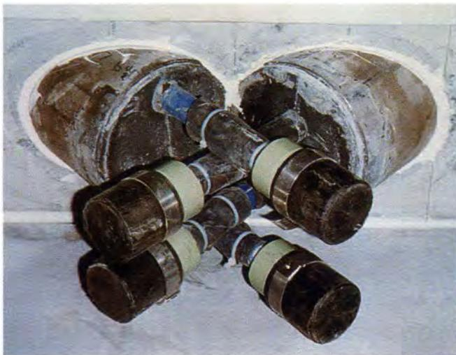
Fig. 10. Closeup of diagonal members positioned in form, with custom-designed, miniaturized anchorages for two greased-sheathed monostrands in each diagonal.
