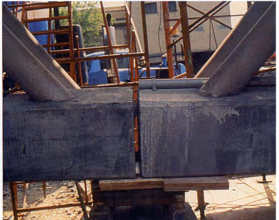
Fig. 14. Precise fitting of adjoining segments was possible because they were match cast.
