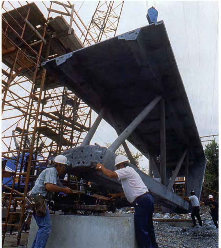
Fig. 13. Positioning a bridge segment for assembly with two others into a half span to be lifted for final erection.
