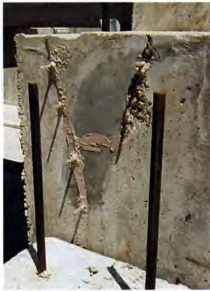
Fig. 4. Sealing cracks.
