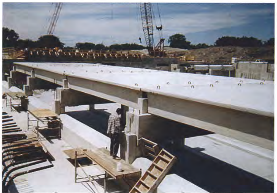
Fig. 2. Water Treatment Basin.
