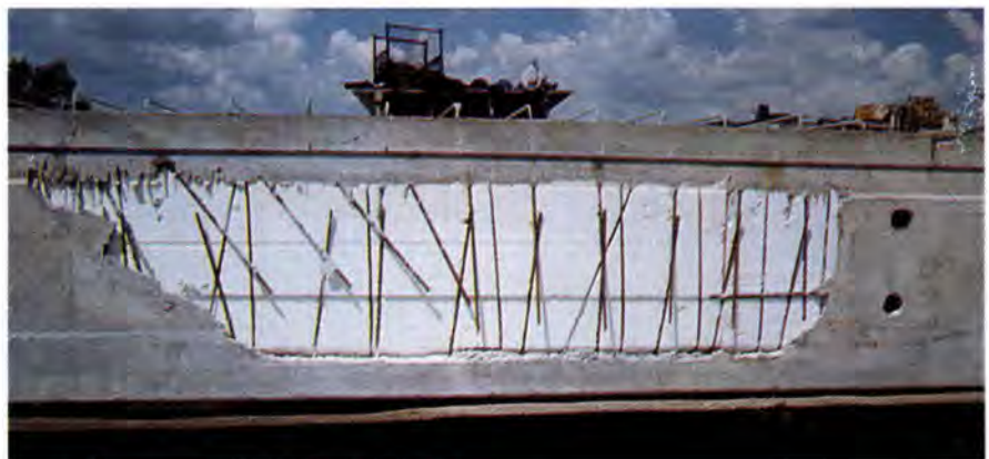
Fig. 11. Exposed voids in a box beam.
