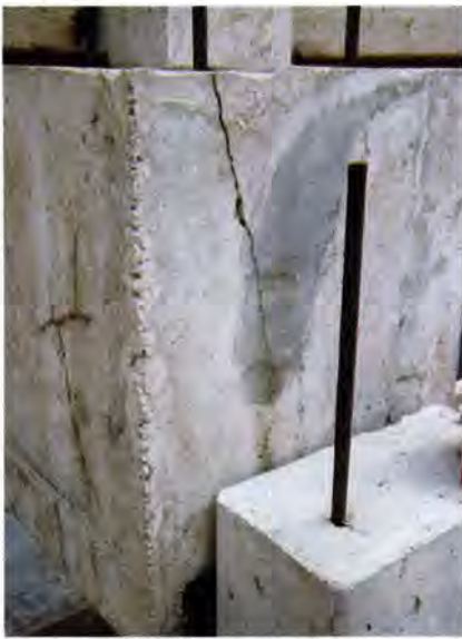
Fig. 3. Inverted tee beam cracks.
