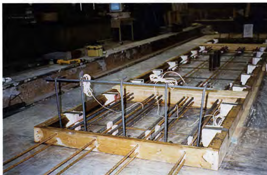
Fig. 10. Details of completed forming.
