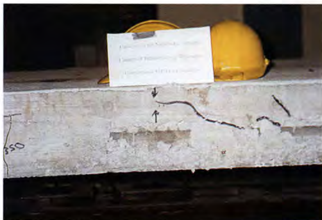
Fig. 16. Flexural cracking at ultimate load.
