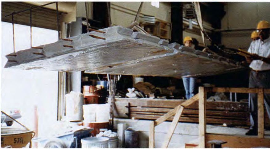
Fig. 11. Precast panel during handling displaying good stiffness.
