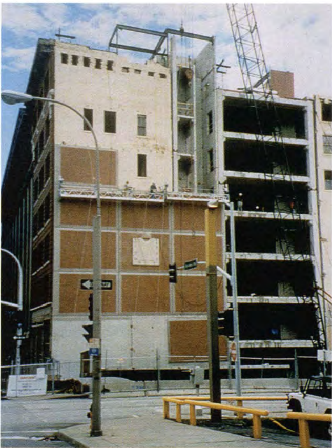
Fig. 10. Erection of precast façade.
