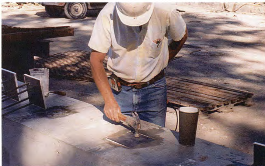
Fig. 4c. Tapping of plate to eliminate air voids.
