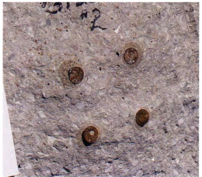
(b) Bottom surface of failure cone at the studs.
