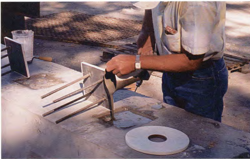
Fig. 4a. Filling void with fluid grout.
