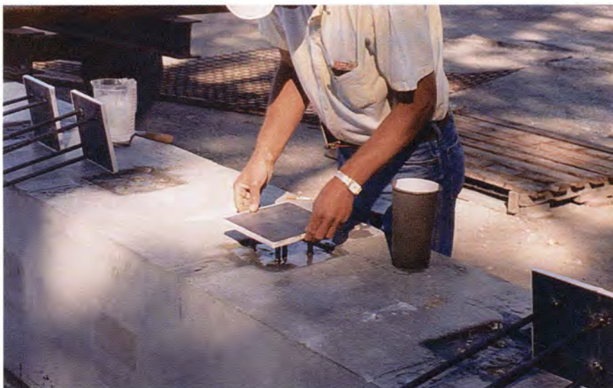
Fig. 4b. Placing plate in grout-filled void.
