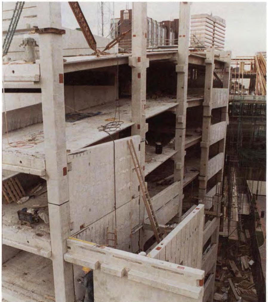
Fig. 4. Construction of a precast skeletal structure at The Bourse, Leeds, United Kingdom (Courtesy: Blatcon Ltd., United Kingdom).
