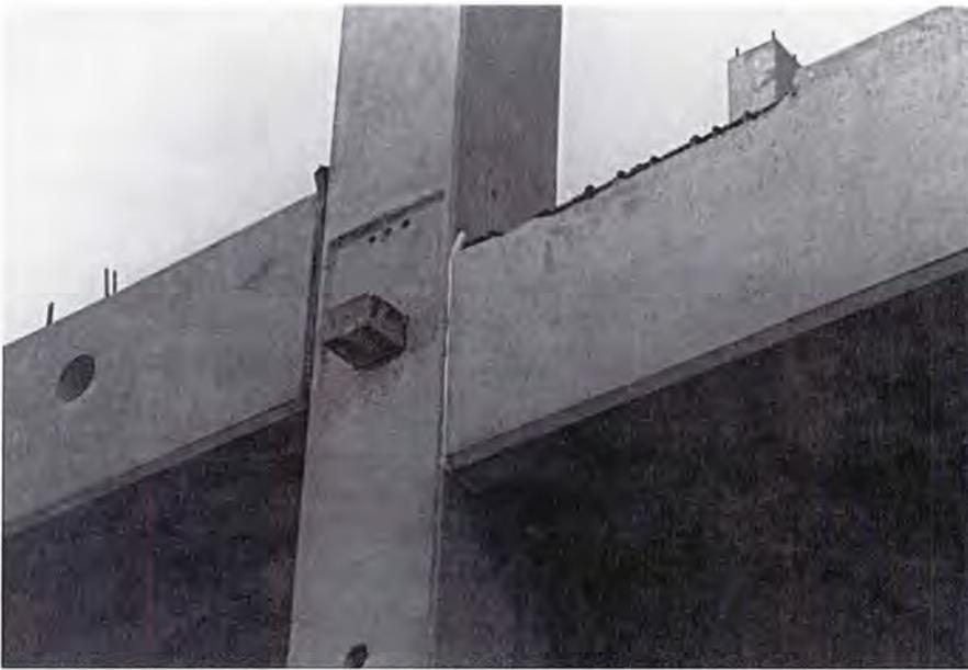
Fig. 8. Billet connector as used in multistory precast frames.
