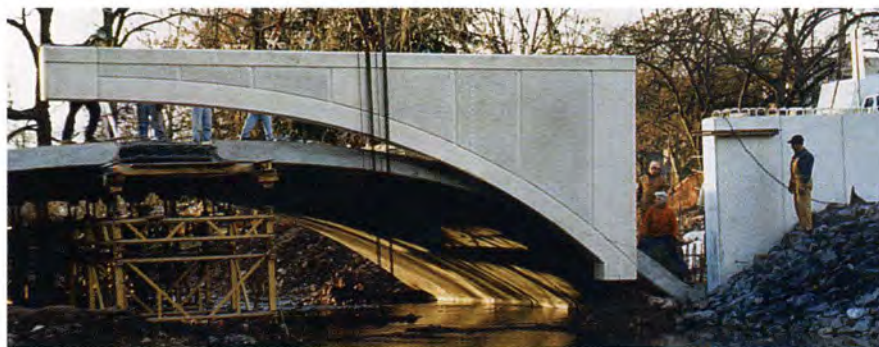
Fig. 11. Installing fascia panel.
