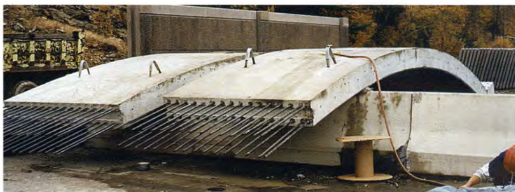
Fig. 9. Finished arched panels at precasting plant ready for shipment to project site.
