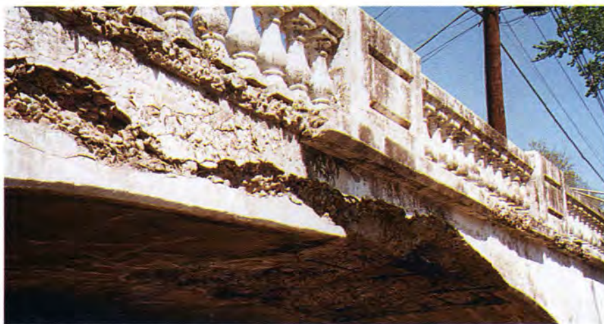
Fig. 3. Close-up of bridge showing significant deterioration of concrete.
