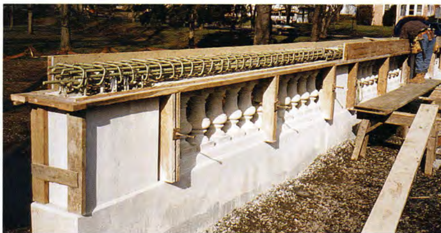
Fig. 13. Reinforcing cage for cast-in-place top rail.
