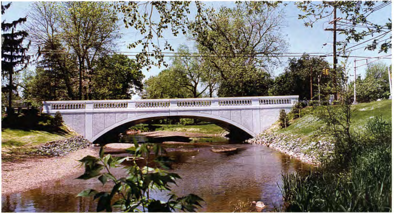
Fig. 16. Award winning bridge shows attractive precast panels integrated with cast-in-place keystone piece.
