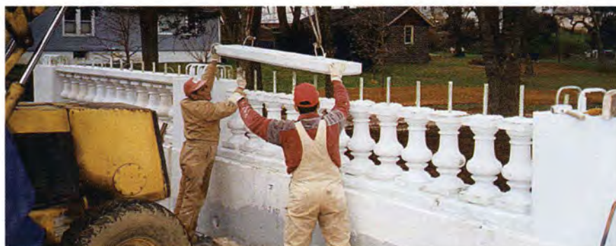
Fig. 12. Hoisting precast panel on top of balusters as a bottom form for cast-in-place top rail.
