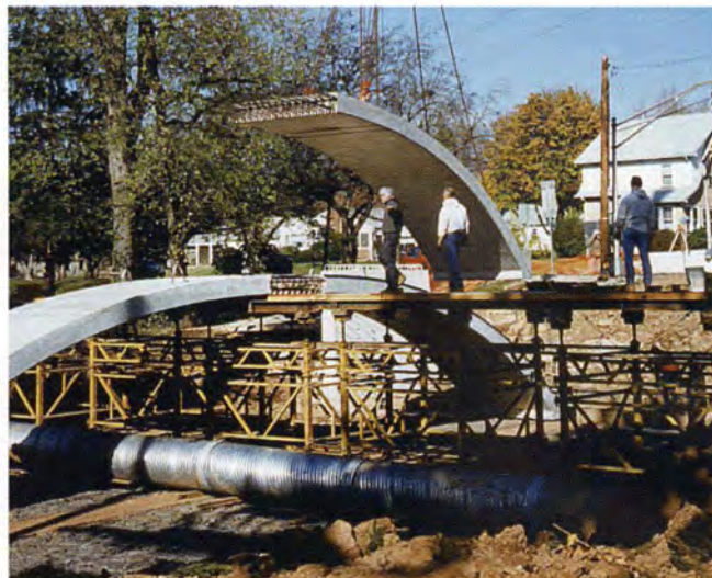
Fig. 10. Hoisting curved panel.
