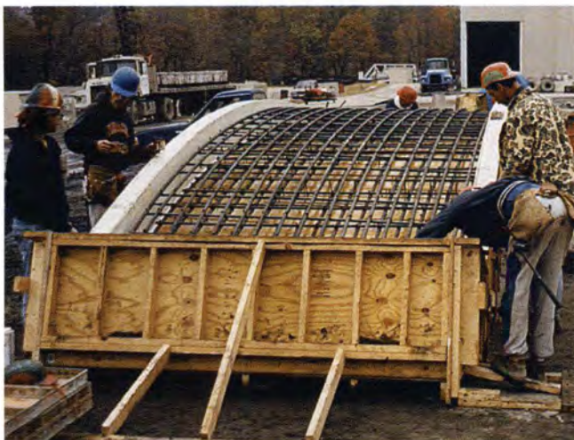
Fig. 8. Fabrication of arched panel showing reinforcement and formwork.
