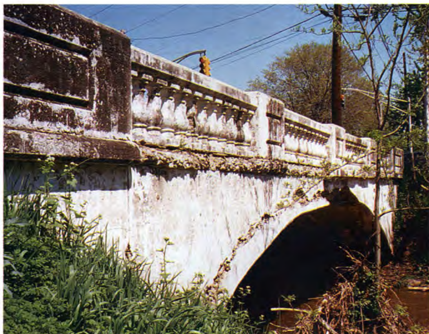
Fig. 2. Old deteriorated arch bridge showing extent of damage.
