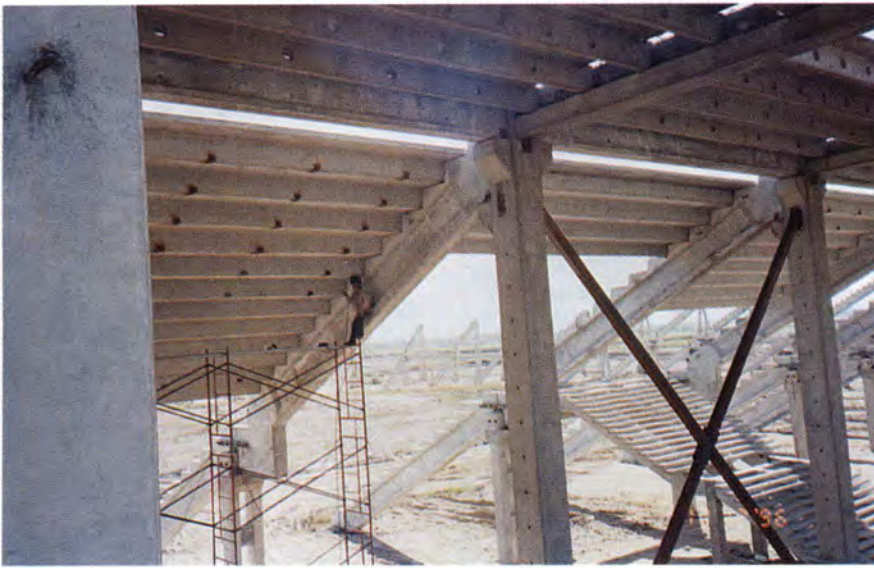
Fig. 9. The steel cross bracing and the staircases.
