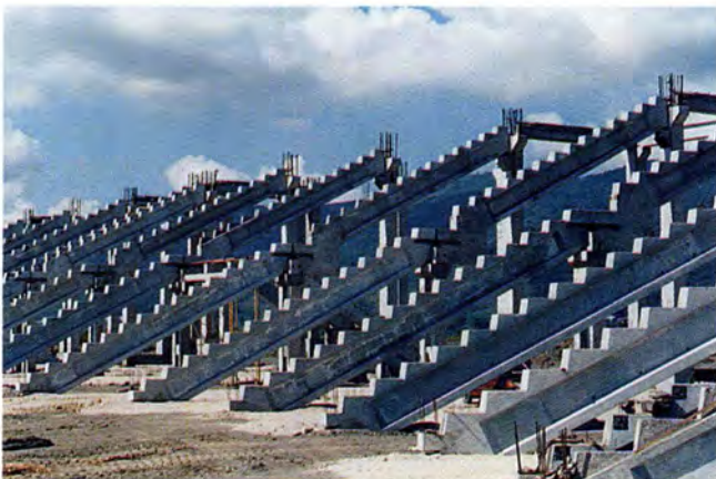
Fig. 7. Erection of primary beams.
