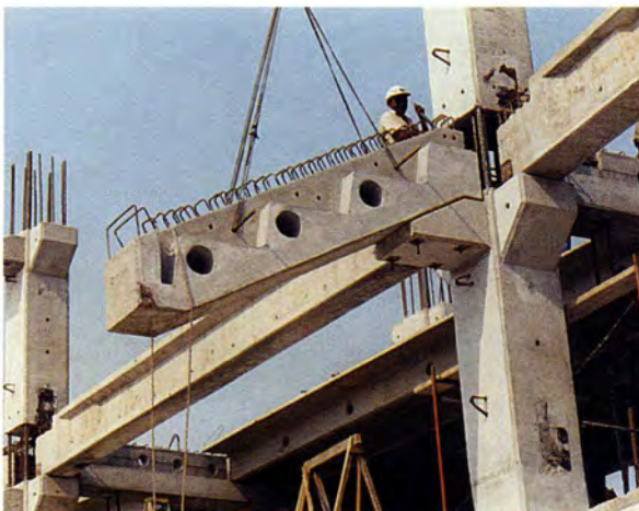
Fig. 15. Erection of cantilever beam.
