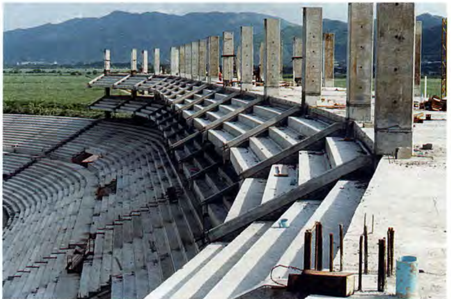
Fig. 27. Column, riser and cantilever beam on floor.
