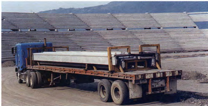
Fig. 18. Arrival of single riser at project site.
