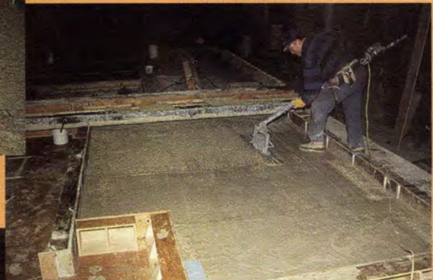
Fig. 4.1.d. Placing 2 in. (51 mm) thick insulation; insulation is pre-drilled at 16 in. (406 mm) on center to accept pin style connectors.
