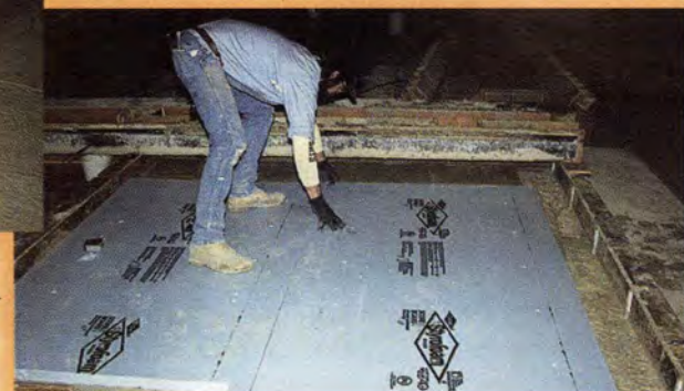
Fig. 4.1.d. Placing 2 in. (51 mm) thick insulation; insulation is pre-drilled at 16 in. (406 mm) on center to accept pin style connectors.
