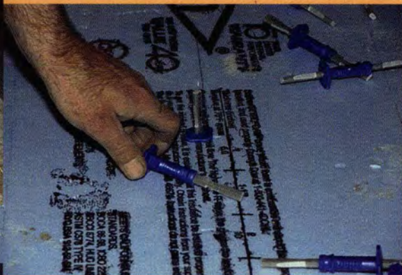
◀ Fig. 4.1.h. Placing pin connector through insulation.
