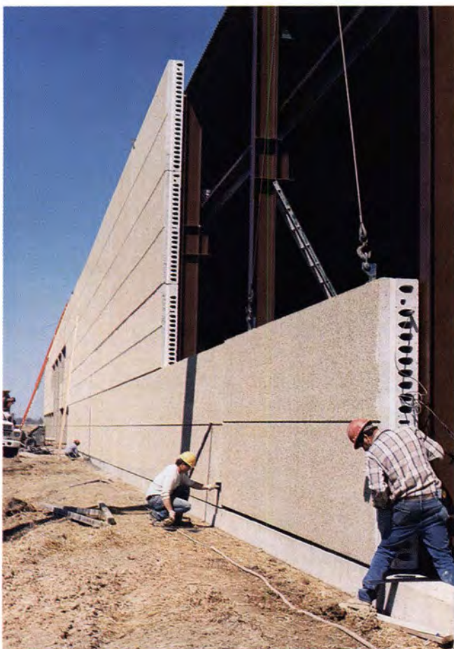
Fig. 1.5.e. Erection of sandwich wall panels – Spancrete Industries, Inc.
