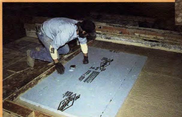
Fig. 4.1.e. Placing 2 in. (51mm) thick insulation; insulation can go outer edge to outer edge, and/or can incorporate certain areas of panels that are non-insulated, depending on design criteria required.
