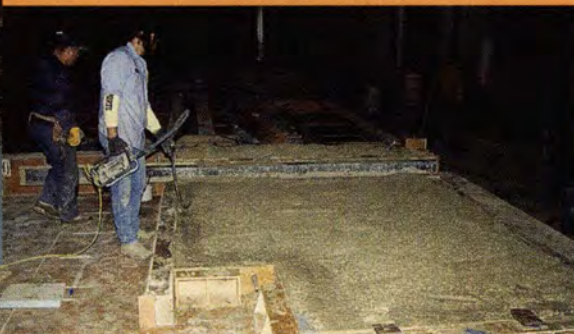
◀ Fig. 4.1.l. Blockout of foam around edge handling insert.
