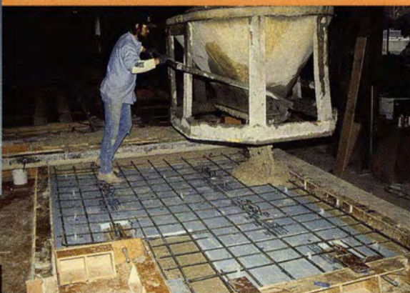
◀ Fig. 4.1.l. Blockout of foam around edge handling insert.
