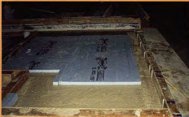
Fig. 4.1.g. Pin connector in place through insulation and full pin connectors. ▶
