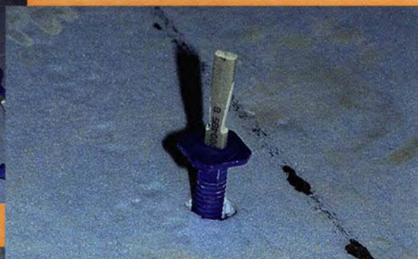
◀ Fig. 4.1.j. Pin connectors in place.
