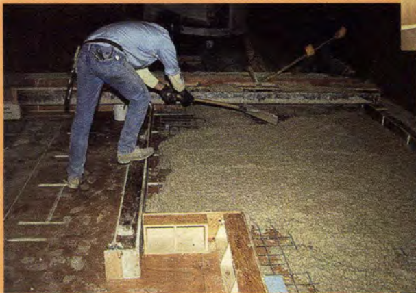
Fig. 4.1.c. Vibrating face mix using bull float vibrator.
