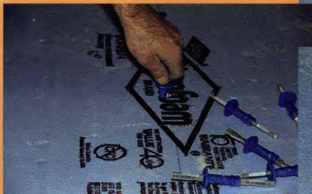
Fig. 4.1.i. Pin connector partially through insulation. ▶
