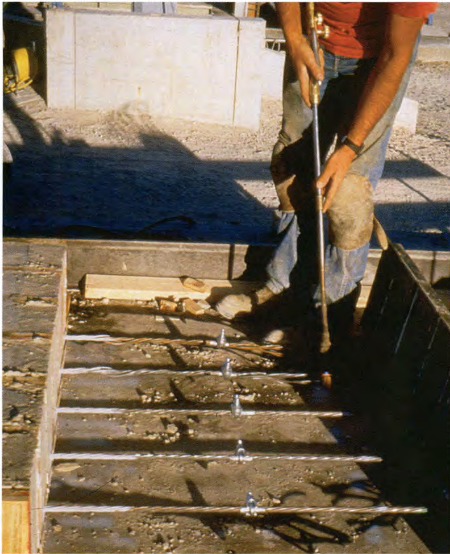
Fig. 13. Release of prestress force by flame-cutting at ends of 90 ft (27.4 m) beam length (May 18, 1996).
