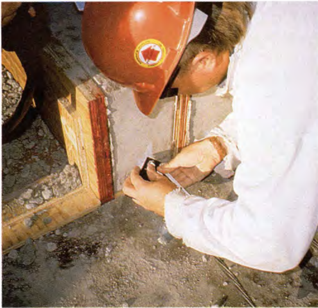
Fig. 20. Measurement of initial strand slip at release of prestress, flame-cut end (May 18, 1996).
