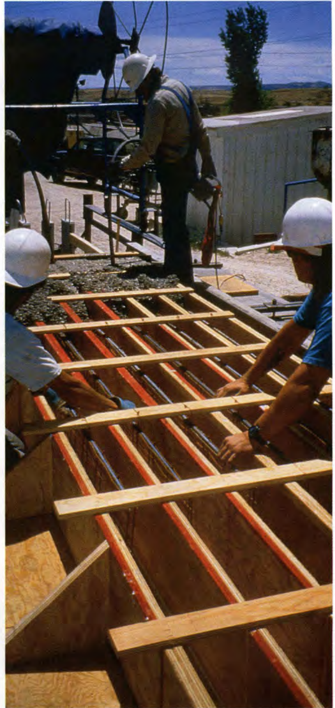
Fig. 12. Casting beam specimens (May 17, 1996).
