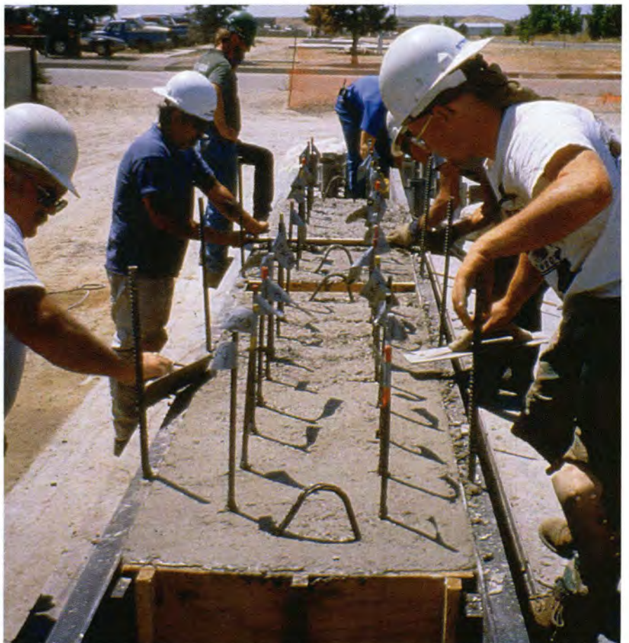
Fig. 6. Completion of casting and finishing pull-out test blocks (May 17, 1996).
