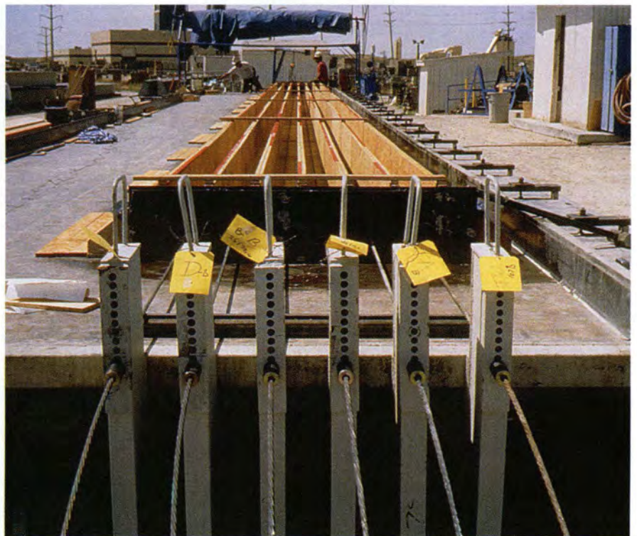
Fig. 10. Beam test specimens. Six strand specimens after prestressing (May 17, 1996).
