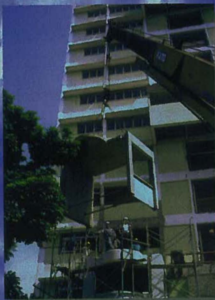
Precast core volumetric being stack into place
