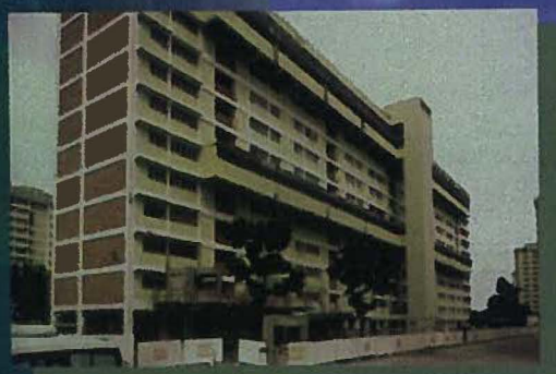
Front view of blk 24 before completing of pilot upgrading works
