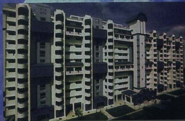
The same blk 24 totally transformed after upgrading
