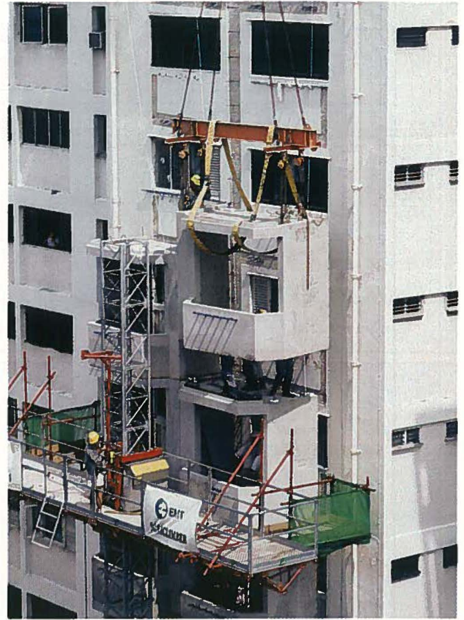
Fig. 15. Work platform and precast volumetric stacking system combination improves erection speed.
