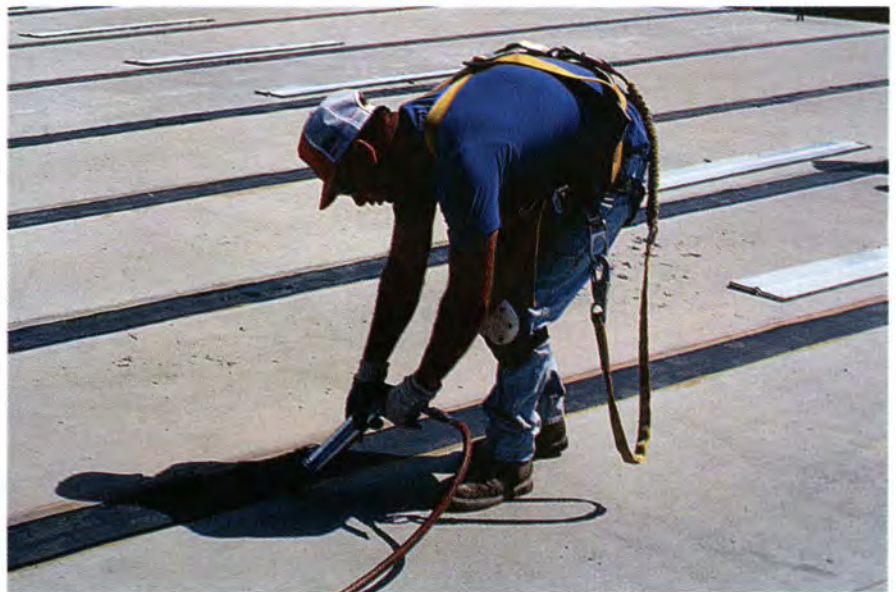
Fig. 18. EPDM placed at roof joints.
