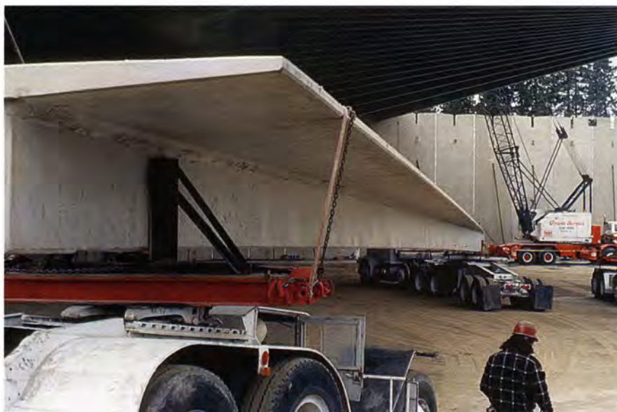
Fig. 14. Steering trailers were used to deliver roof tees to the jobsite.
