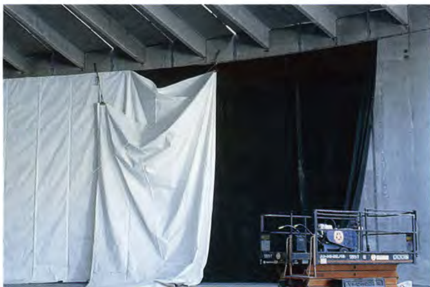
Fig. 16. Placement of geotextile material and tank liner.
