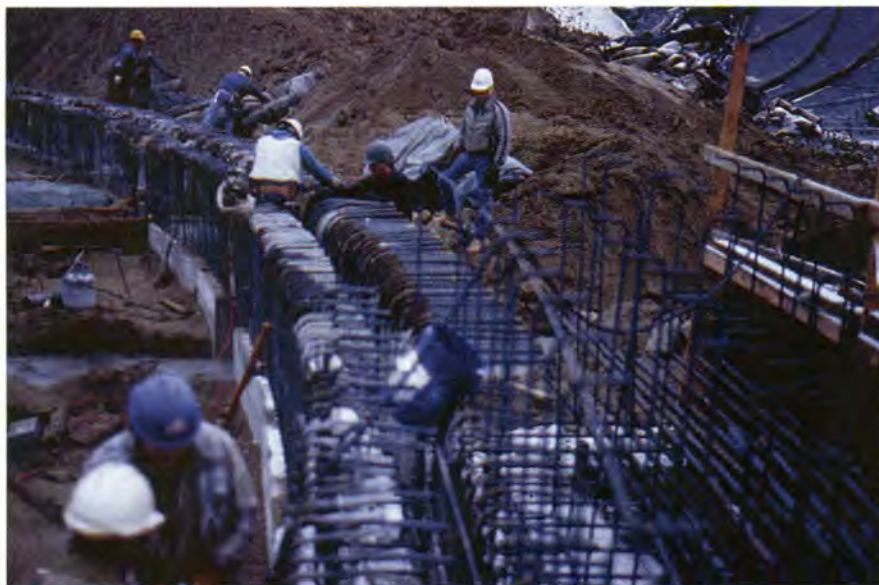
Fig. 12. Placement of reinforcing bars in footings.
