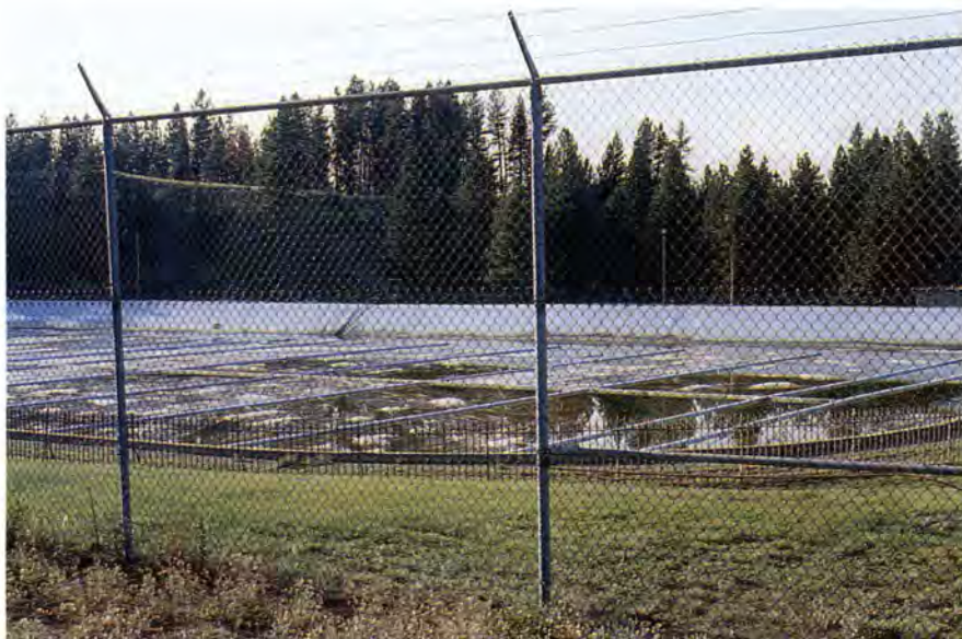
Fig. 2. The existing Lincoln Heights reservoir with deteriorating floating cover.
