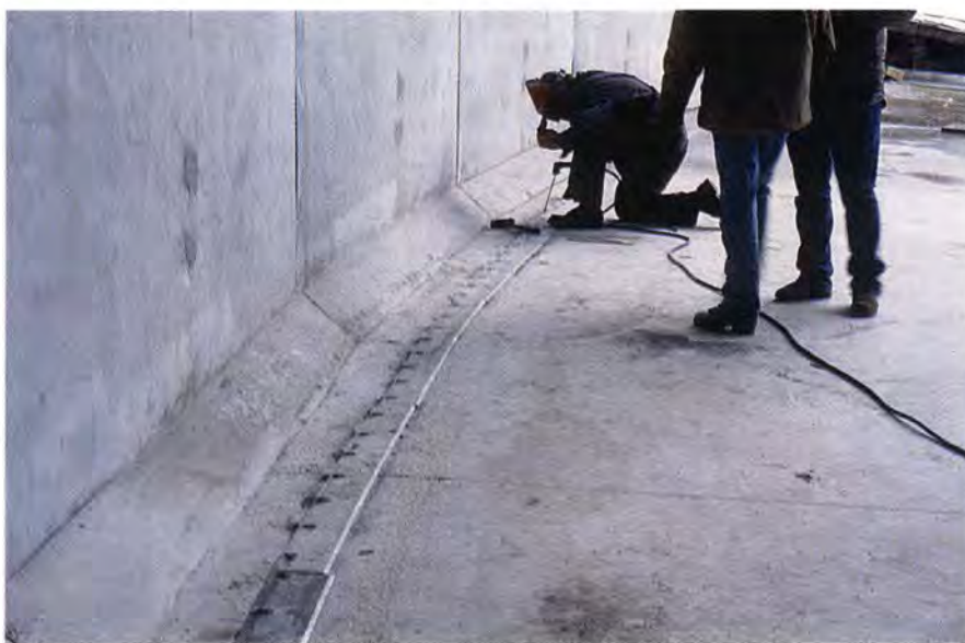
Fig. 15. A stainless steel sliding plate was welded across the joint in the bottom slab between the footing and floor.
