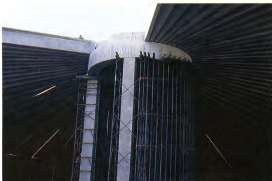
Fig. 13. Ring beam shoring for roof tee placement.
