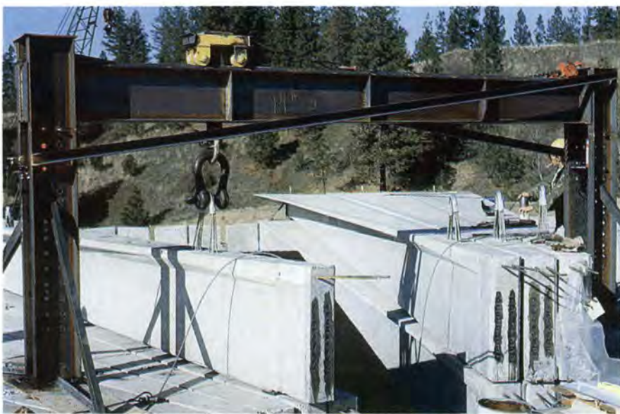
Fig. 17. A hanger and trolley system was used to position roof members.
