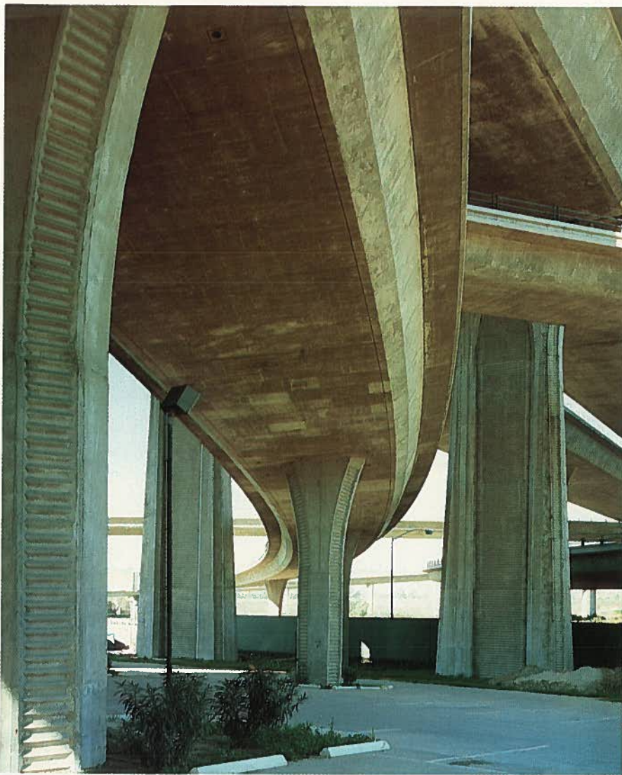
Fig. 3. The cast-in-place box girder became popular in California bridge construction.
