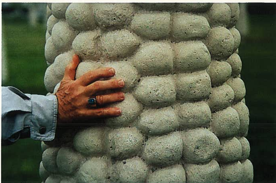
Fig. 8. Detail of the precast concrete kernels. (© M. K. Hurd)
